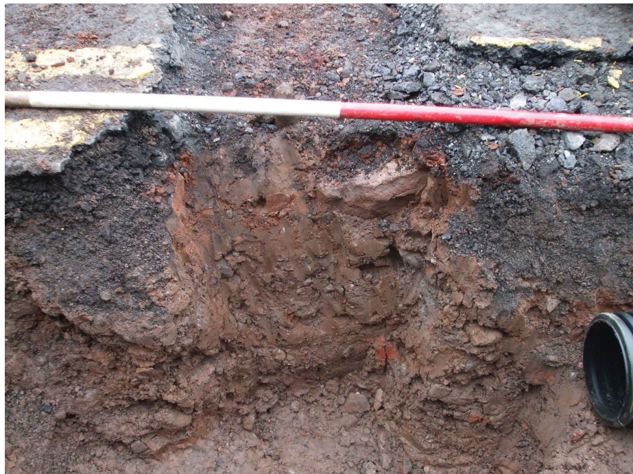
Fig 4 - Pit for side entry gully, Northeast-facing
