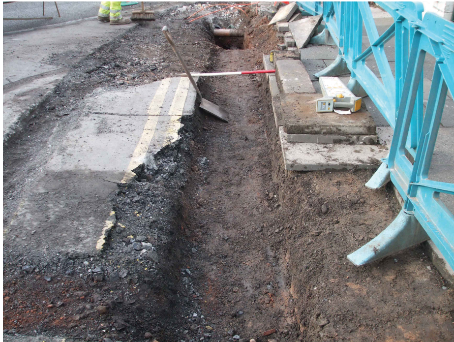
Fig 3 - Trench for connecting pipe taken from Southeast
