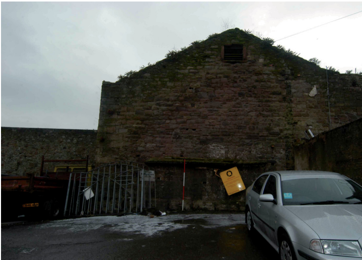
Plate 9 - North facing gable of the former engineering workshop (Unit 5)
