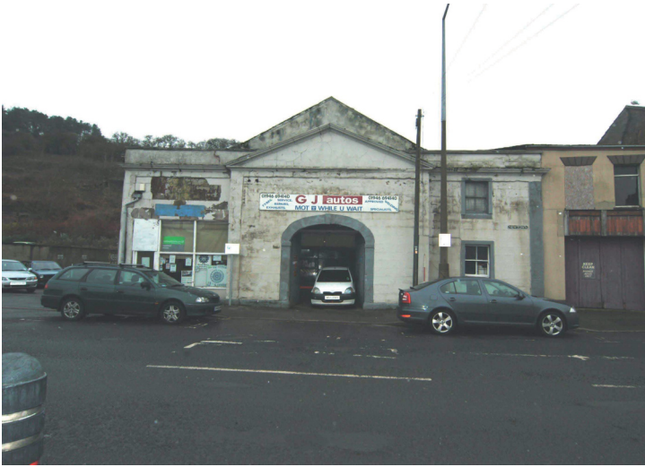
Plate 1 - The east-facing elevation of J & G Autos Garage (Unit 1) fronting Newtown Road
