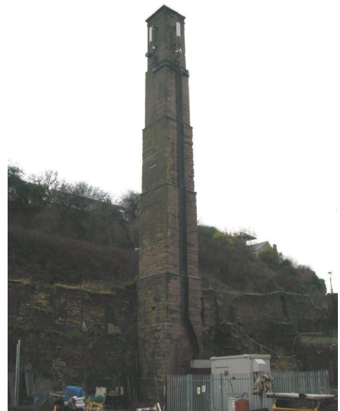
Plate 12 - South-east corner of the Phoenix Foundry chimney (Unit 20)
