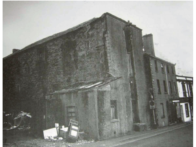
Plate 8 - A photograph taken in 1990 of the former warehouse (Unit 15) prior to its demolition
