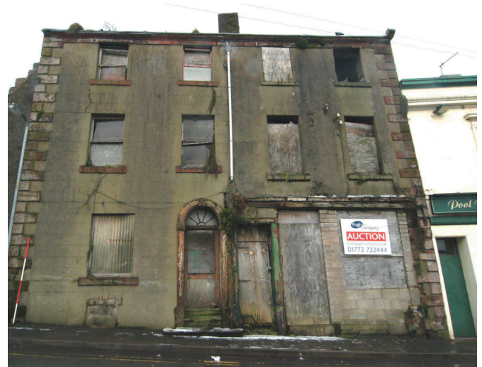
Plate 6 - South-facing elevations of No's 15-17 Albion Street (Units 13 and 14)
