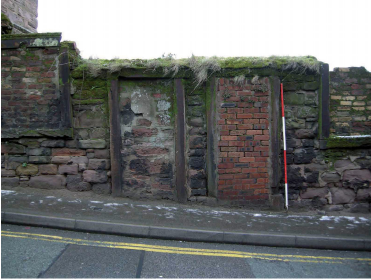
Plate 13 - West-facing building remains (Unit 21) fronting Rosemary Lane
