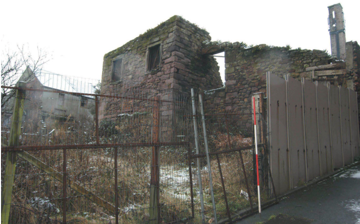
Plate 11 - East facing gable of the former Phoenix Foundry (Unit 18)
