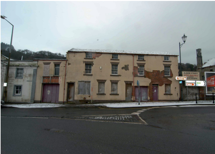
Plate 3 - The east-facing elevations of the 1-3 Newtown Cottages (Unit 6) fronting Newtown Road
