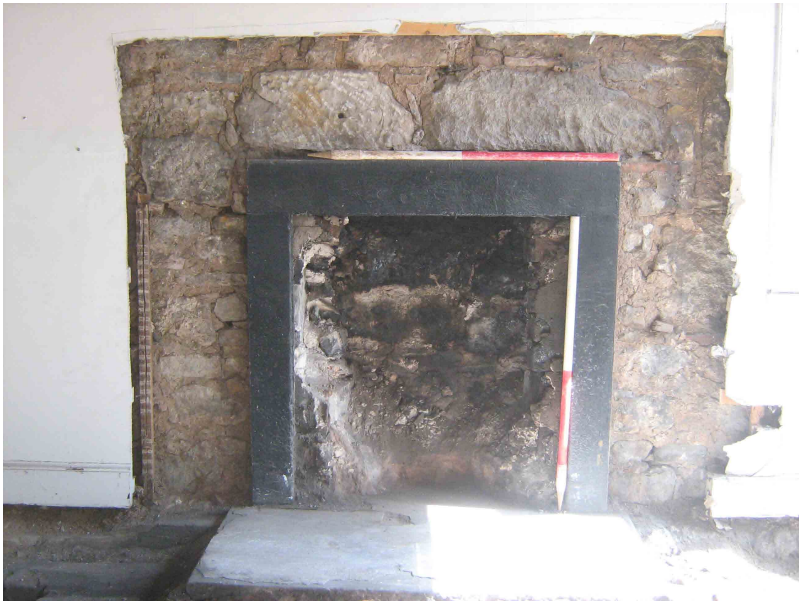
Fig. 3 - Fireplace in Unit 25 after removal of horseshoe surround
