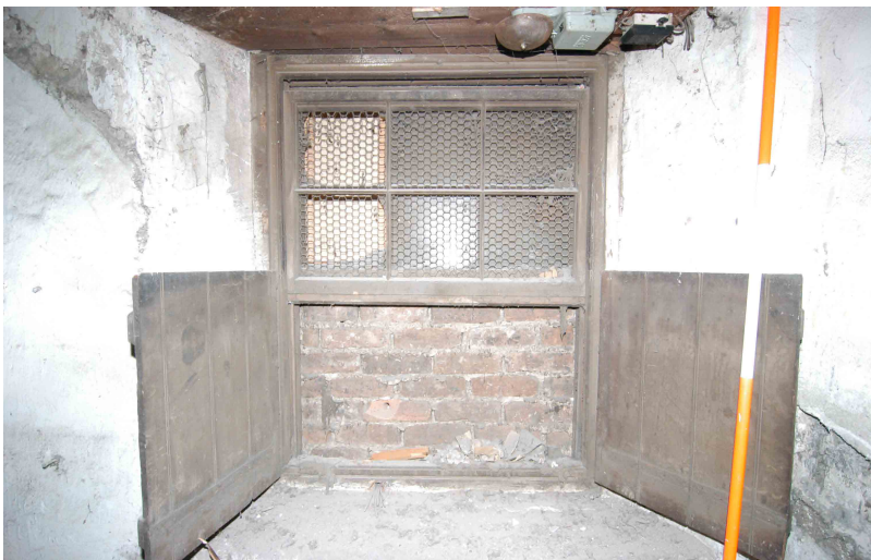
Fig. 5 - Blocked window in Unit 19 after removal of the staircase
