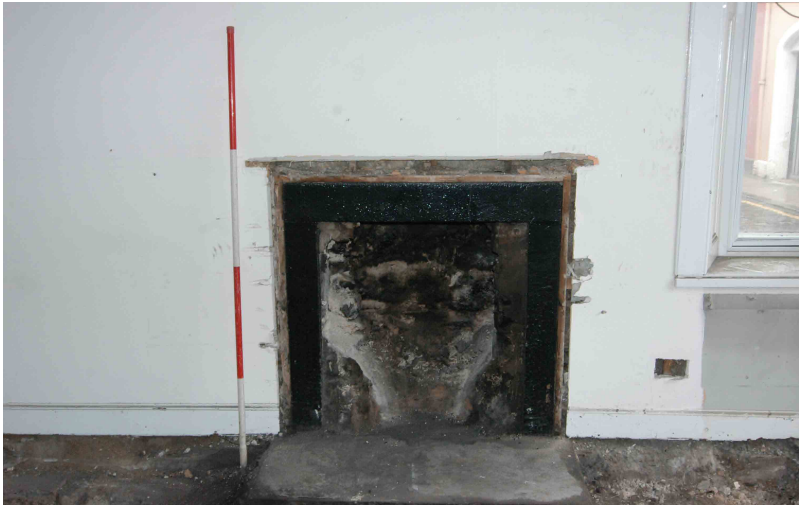
Fig. 4 - Fireplace in Unit 38 after removal of horseshoe surround
