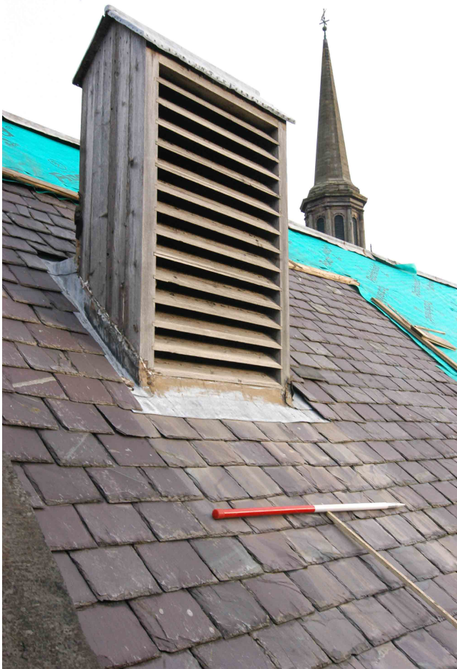
Fig. 6 - Roof vent on the south-facing roof elevation
