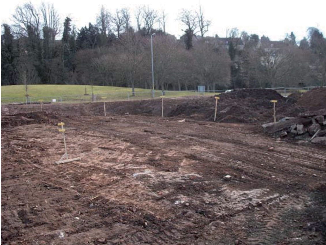
Fig. 6 Eastern half of site following excavation
