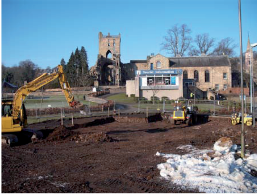
Fig. 2 General shot of site under excavation
