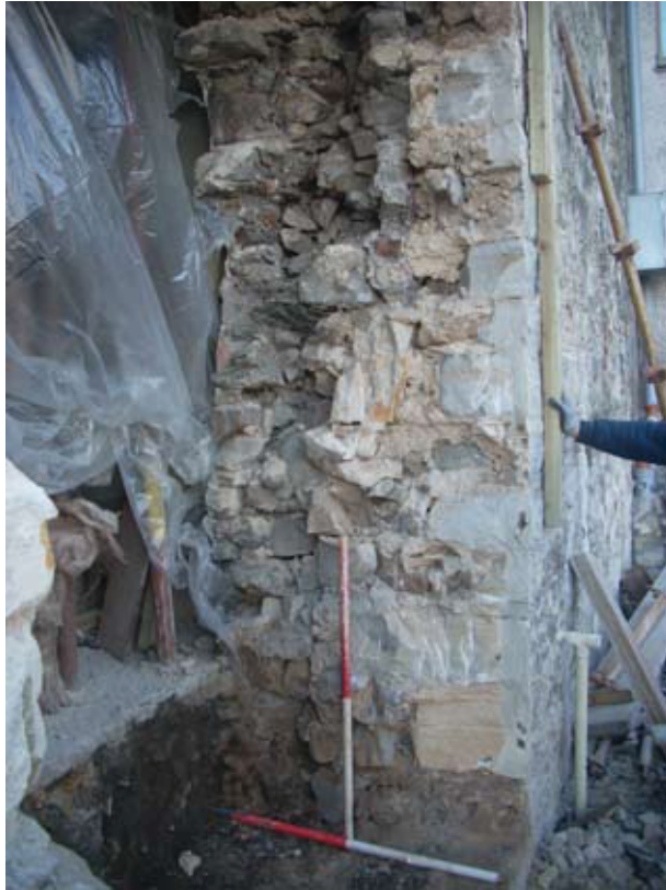
Fig. 2a Shot of north-facing section through wall
