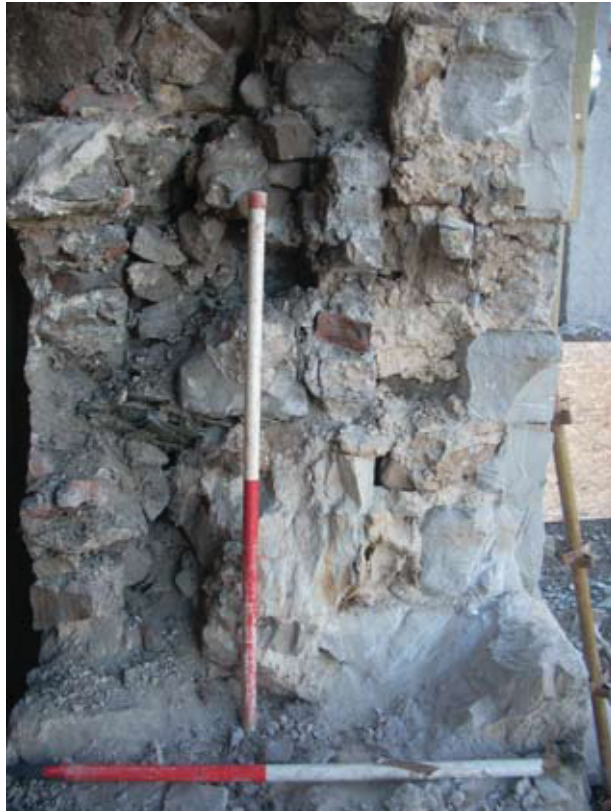
Fig. 2b Detail of north-facing section
