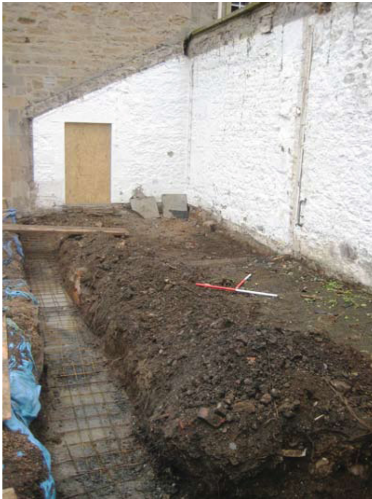
Fig. 2 General shot of site from east
