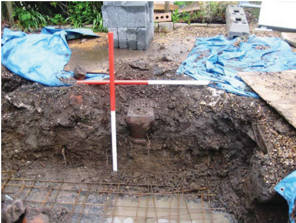
Fig. 5 General shot of south-west facing section of foundation trench
