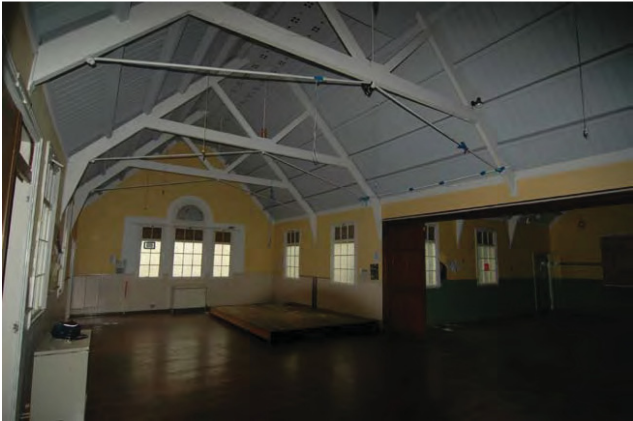
Fig 9. Interior: view of north and east elevation of church
