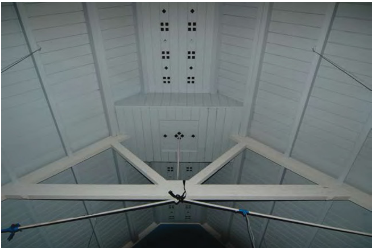
Fig 20. Interior: detail of church roof ridge vents and spire box
