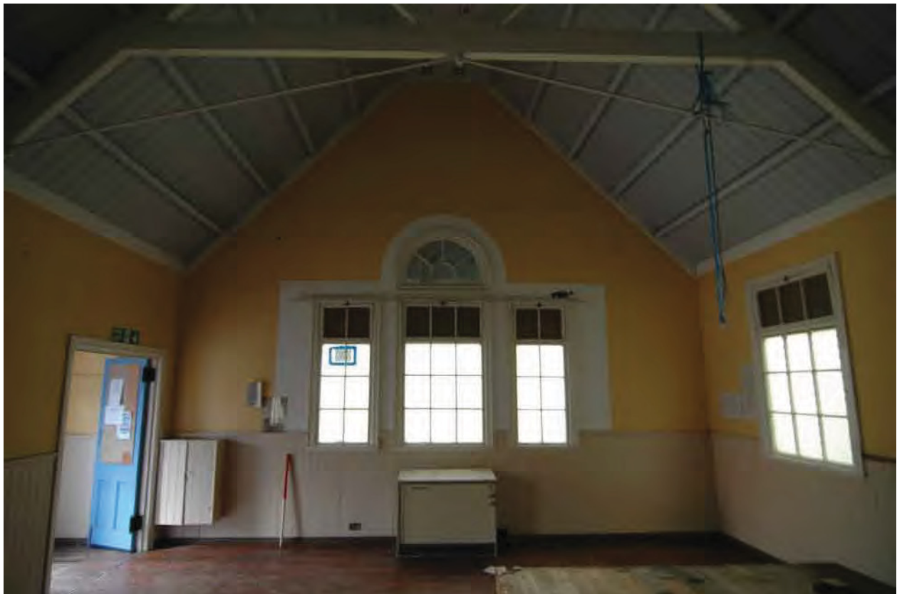
Fig 8. Interior: north elevation of church
