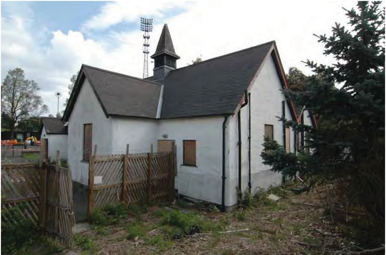
Fig 6. Exterior: view from south-west
