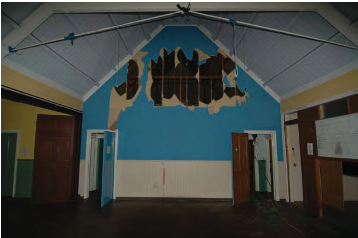
Fig 10. Interior: south elevation of church
