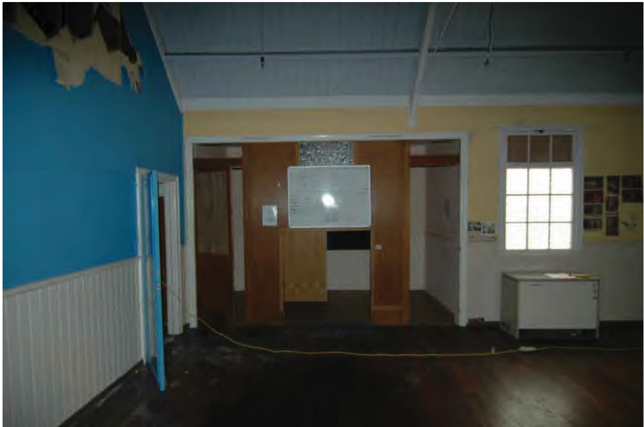
Fig 11. Interior: west elevation, pulpit area
