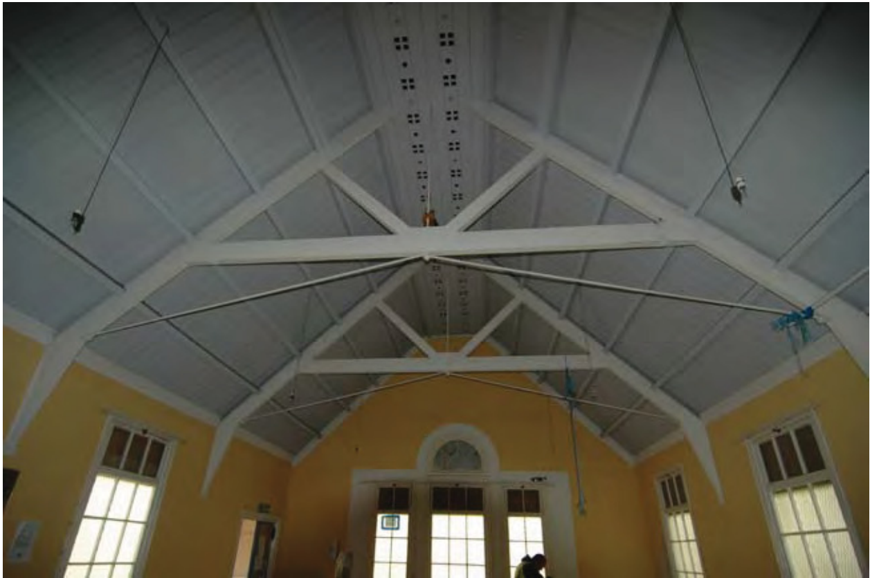
Fig 19. Interior: detail of church roof
