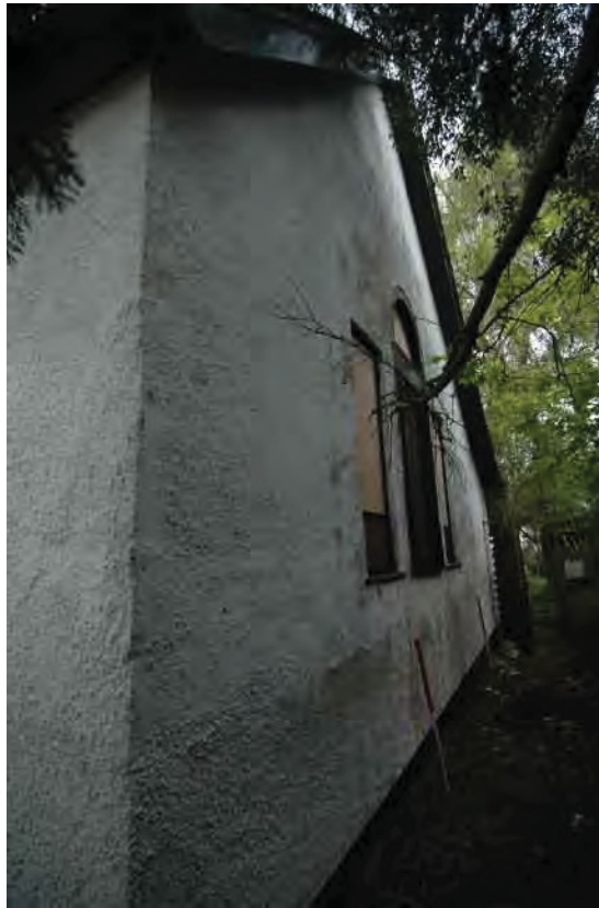
Fig 7. Exterior: oblique view of east elevation
