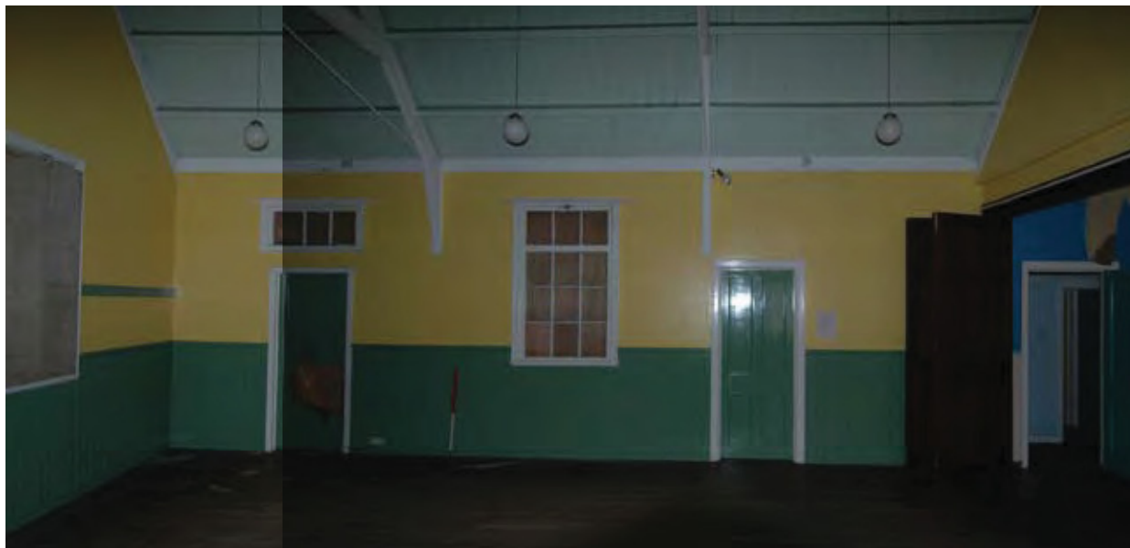
Fig 14. Interior: south elevation of hall
