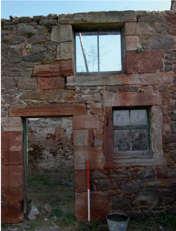
Plate 3 - Building 1, west-facing elevation
