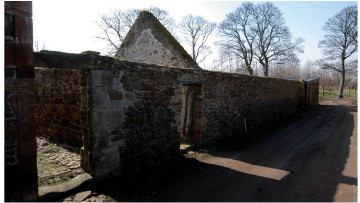
Plate 6 - Building 2, north-facing elevation, Oblique view
