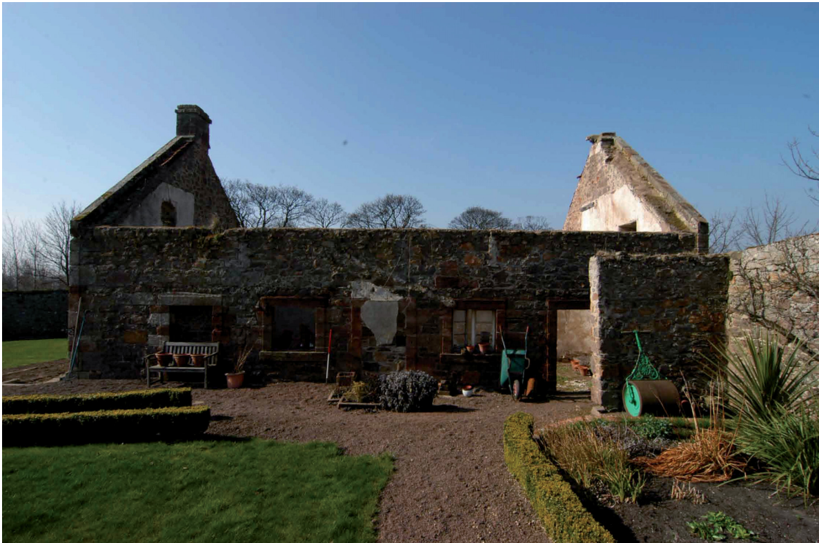
Plate 2 - Building 1 east-facing elevation
