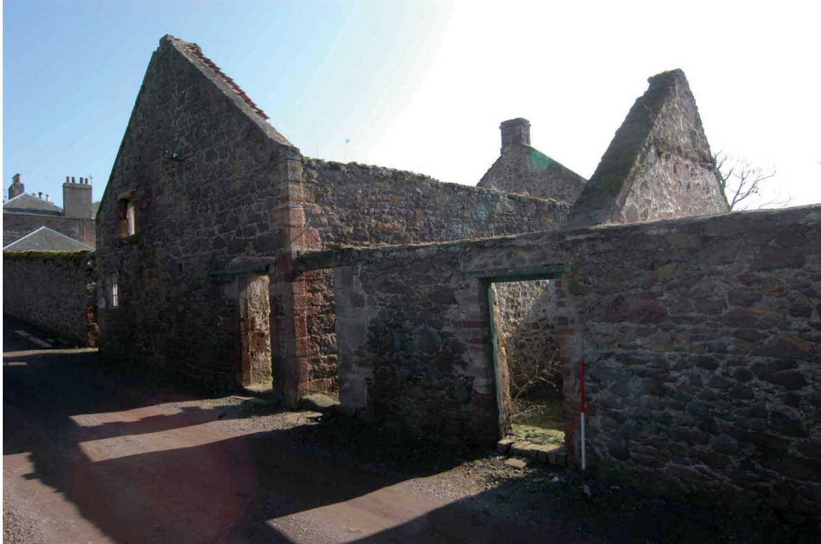
Plate 1 - Building 1 & 2 north-facing elevation
