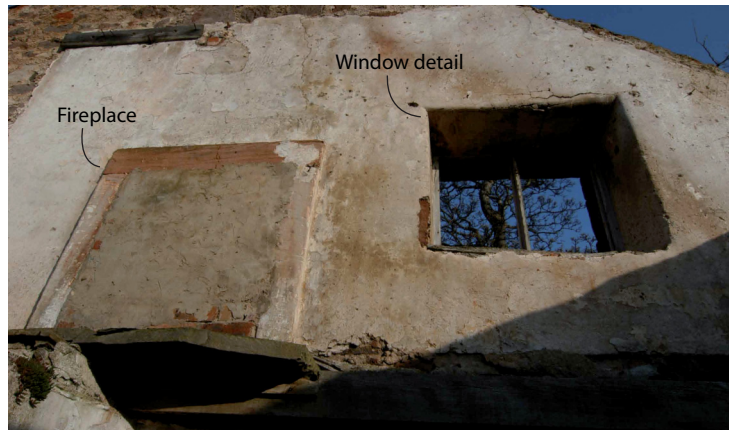
Plate 5 - Building 1, attic interior south-facing elevation
