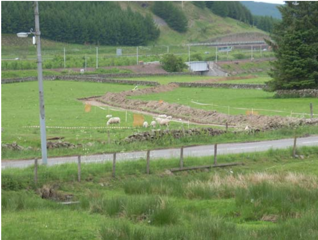
Fig 2. General View of the excavated trench from the north-west
