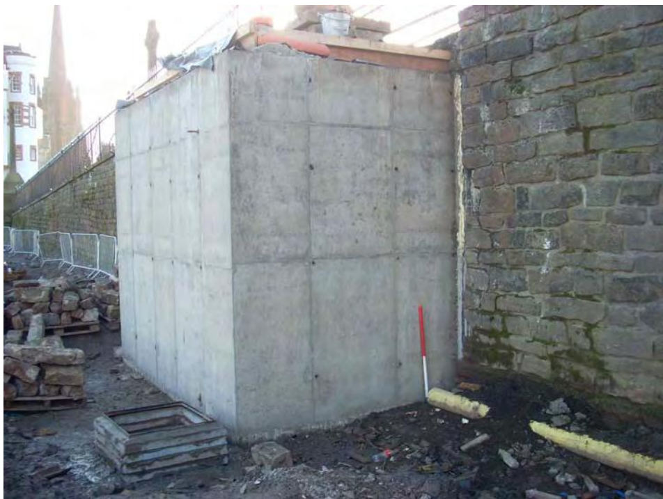
Fig. 9 - General view from the west of the concrete structure of the new abutment
