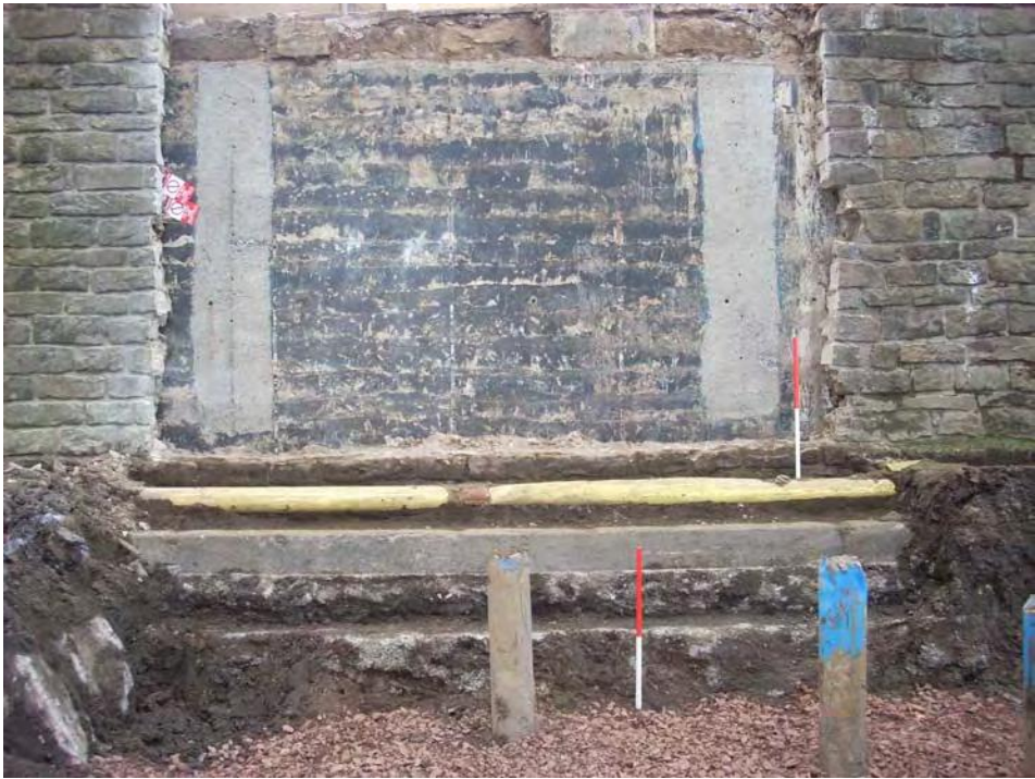
Fig. 7 - View from the north of the concrete wall exposed following the removal of the stone cladding. The concrete foundations are below
