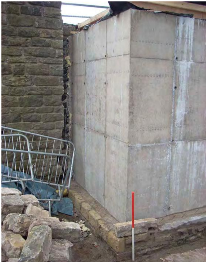
Fig. 10 - The stone cladding being replaced on the new abutment
