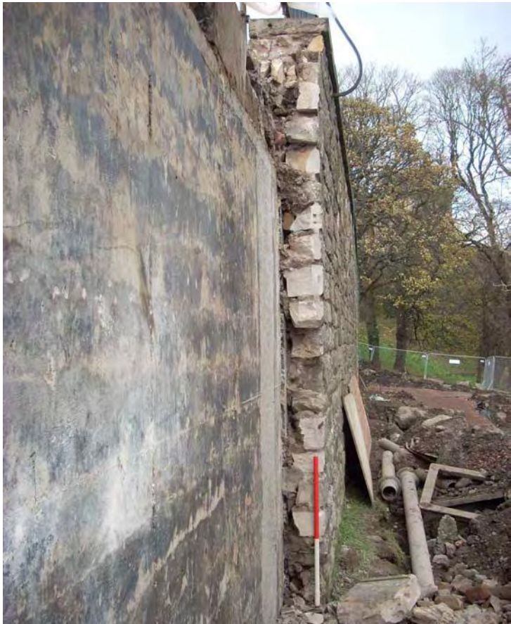
Fig. 8 - View from the east showing the stone cladding of the concrete wall
