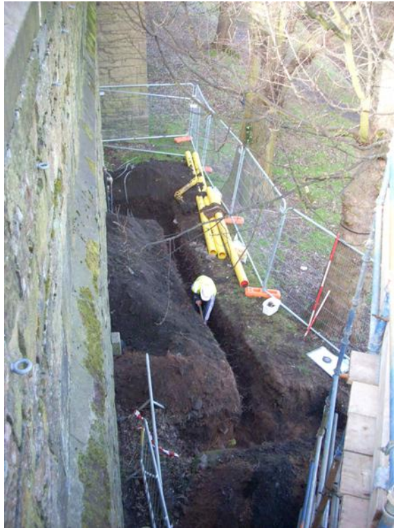
Fig 7. Gas trench in Princes Street Gardens from the east
