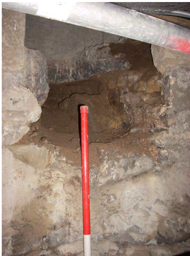
Fig 13. Slapping through Moat Vault wall in section
