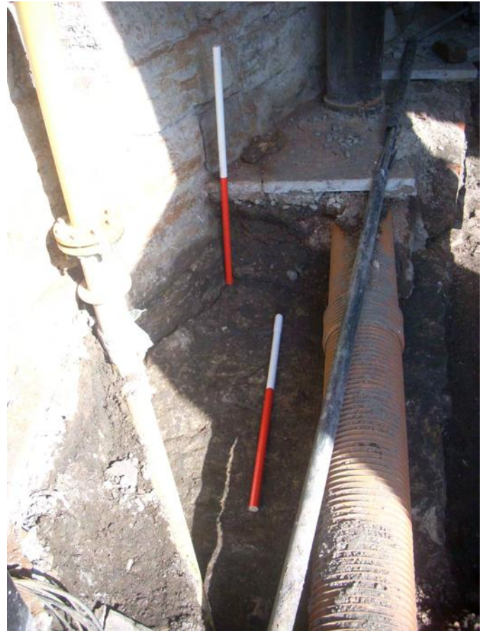
Fig 18. Moat Vault. Masonry 429 abutting west wall 428
