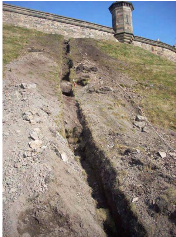
Fig 30. Water Main trench between the Esplanade and Johnston Terrace
