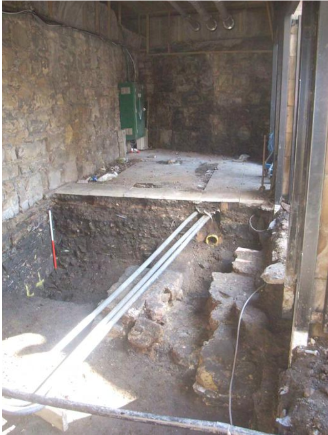
Fig 17. General view of trench in Moat Vault, eastern side
