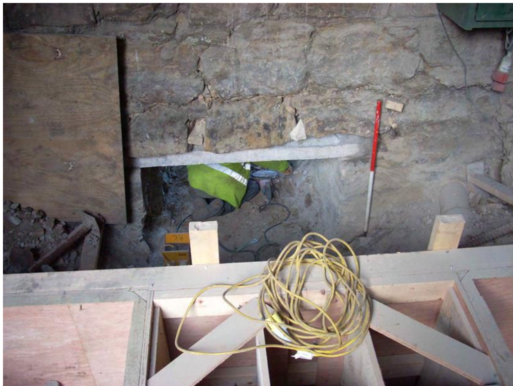
Fig. 24 View of the initial slapping through the Moat Vault 400
