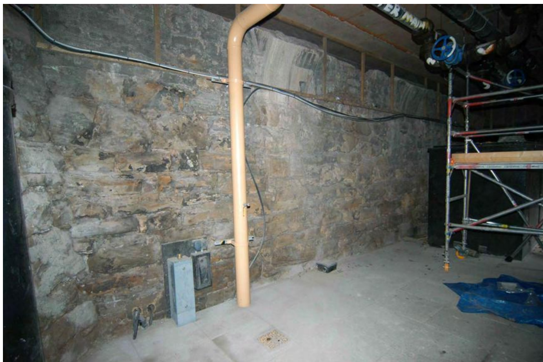
Fig 11. General view of Moat Vault south-facing wall prior to slapping
