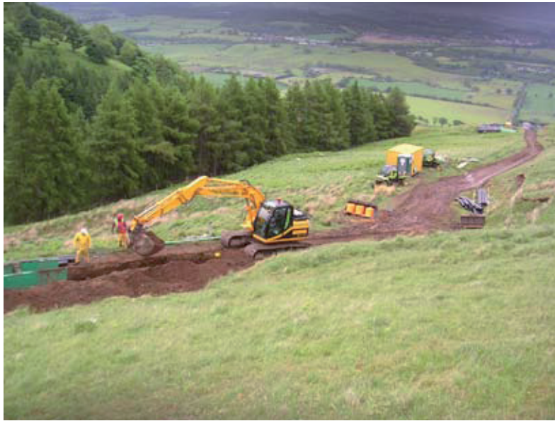
General shot of excavation of grid connection cable from NW
