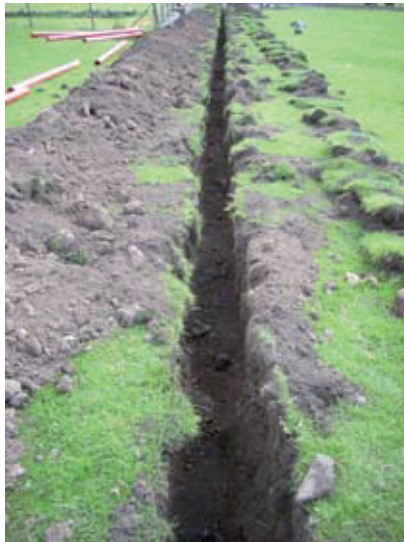
General shot of small electricity cable duct from W
