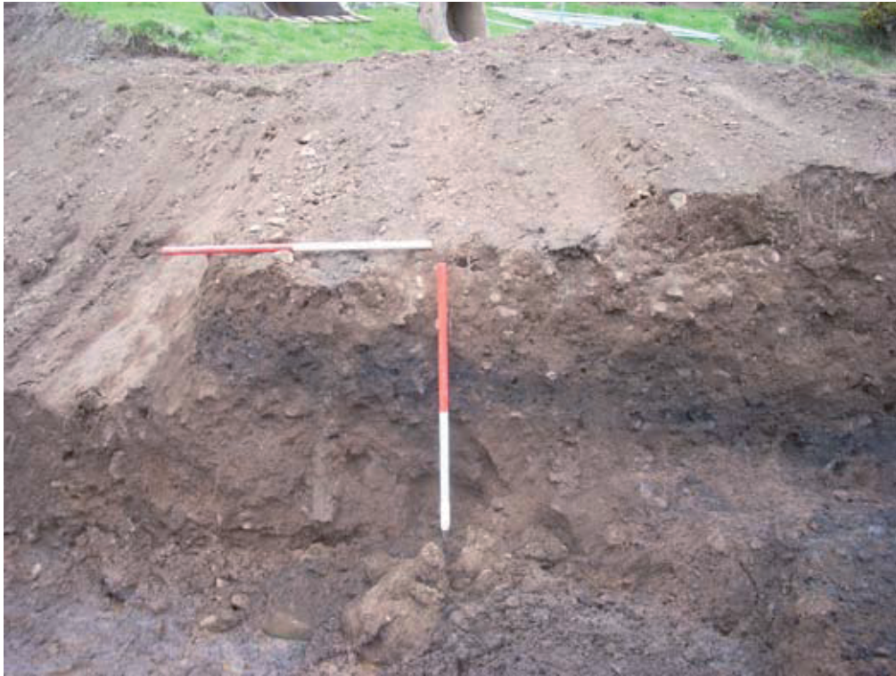
Shot of SSW facing section of part of switching station excavation showing layer (014)
