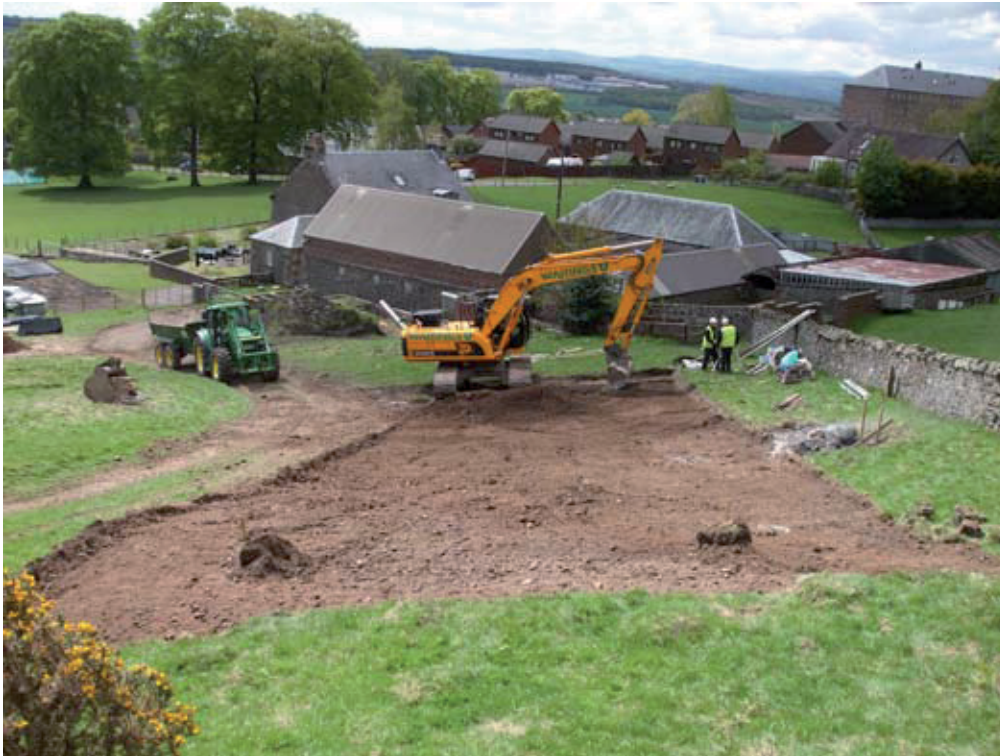
General shot of area being stripped for switching station from N
