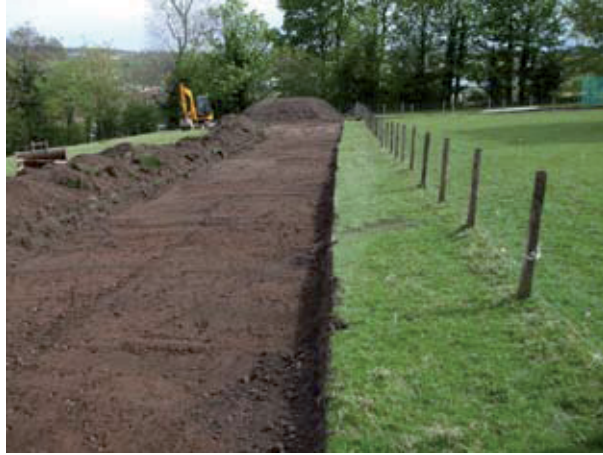
General shot of excavation of access track from NW
