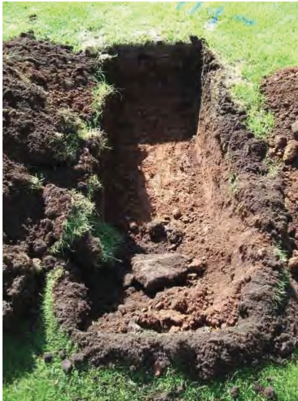
Fig. 4 Topsoil removed from hole for Sign Post 1, from the east
