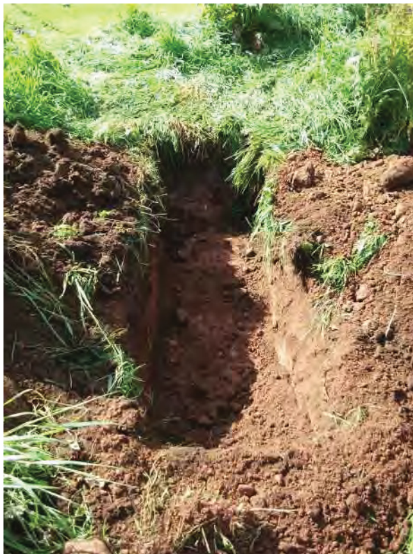
Fig. 5 Topsoil removed from hole for Sign Post 2, from the east
