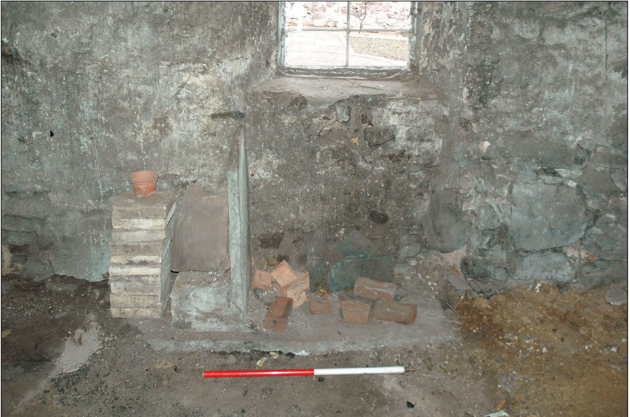
Plate 13: Detail of concrete floor and stone partition on northern internal elevation
