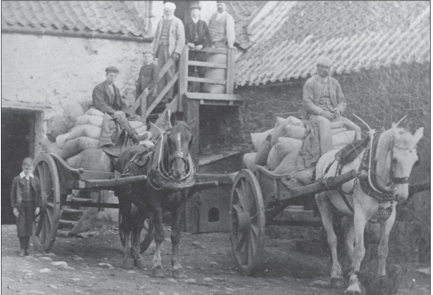
Plate 15: Archive photograph showing southern external elevation. Courtesy of property owners
