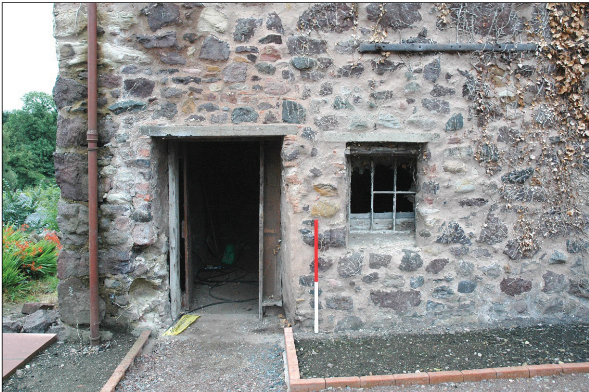
Plate 4: Detail of door and window on northern elevation
