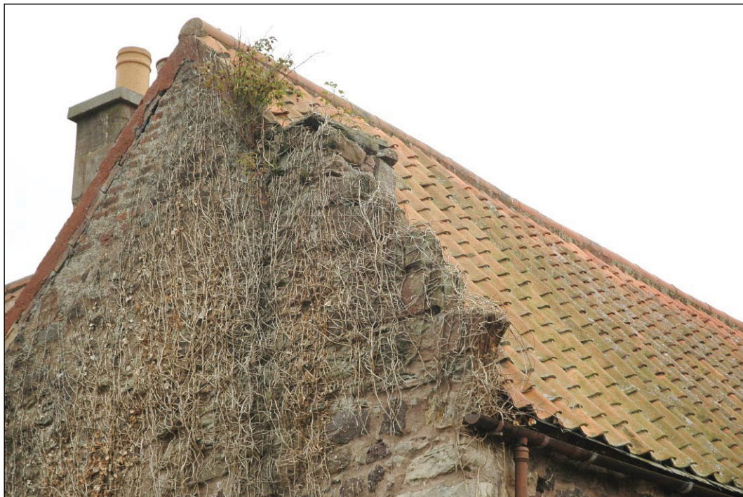
Plate 2: Detail of crow-step gable
