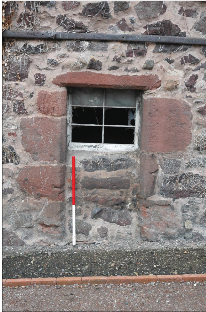
Plate 5: Detail of blocked door on northern elevation
