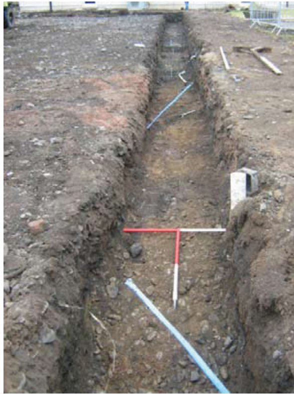
Fig. 4 General view of foundation trenches
