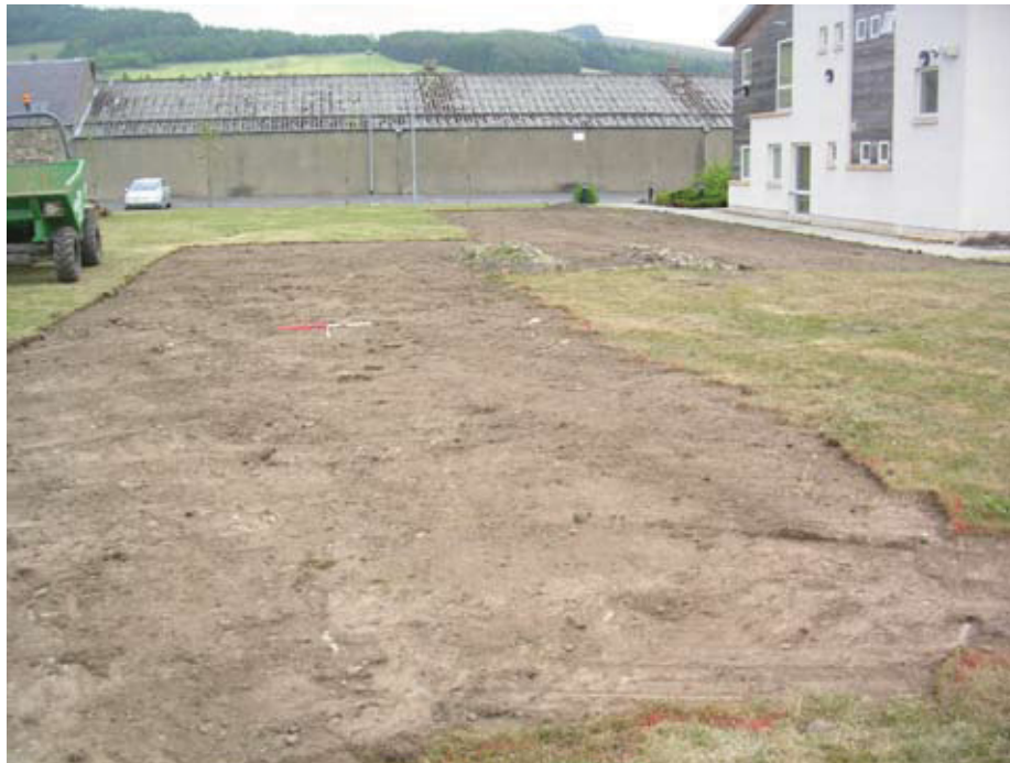
Fig. 2 General view of site and exposed 001 after the removal of turf
