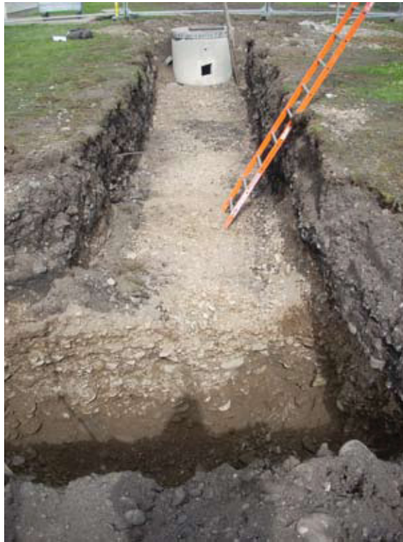
Fig. 6 General shot of excavations for the filtration trench
