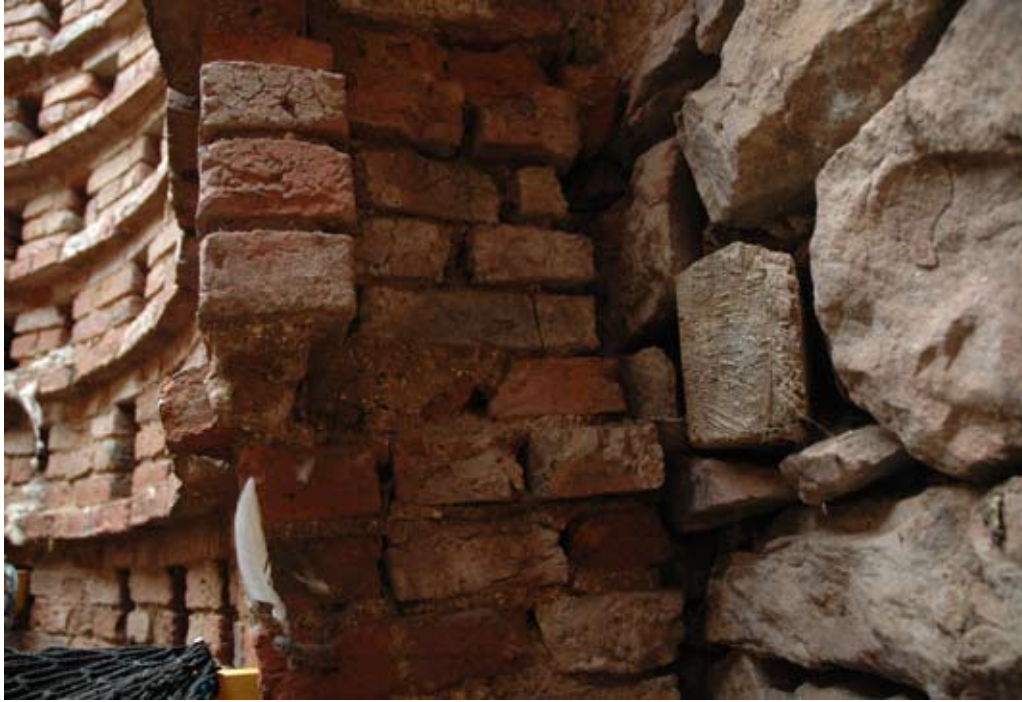
Fig. 10 Joist stub and section of brick nest boxes
