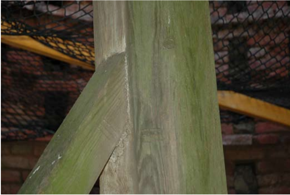
Fig.14 Dowel pin and carpenter's marks
