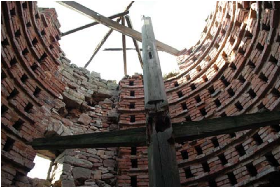
Fig. 6 - Interior of dovecote showing potence, nest boxes and surviving roof timbers
