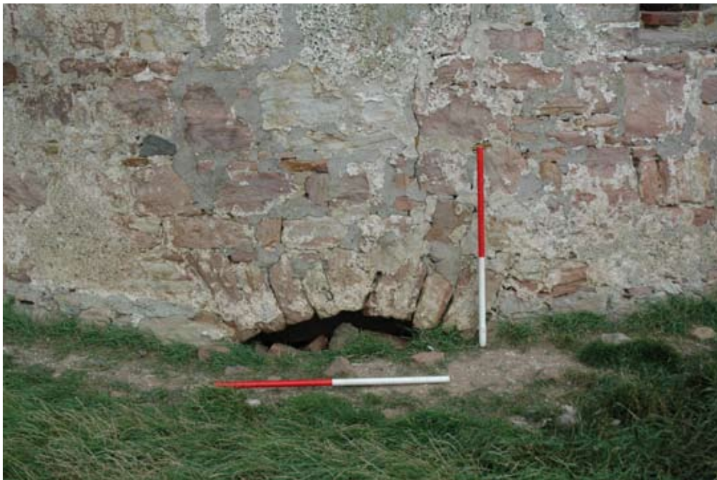
Fig. 18 - Relieving arch above subterranean blocked doorway prior to trench excavation
