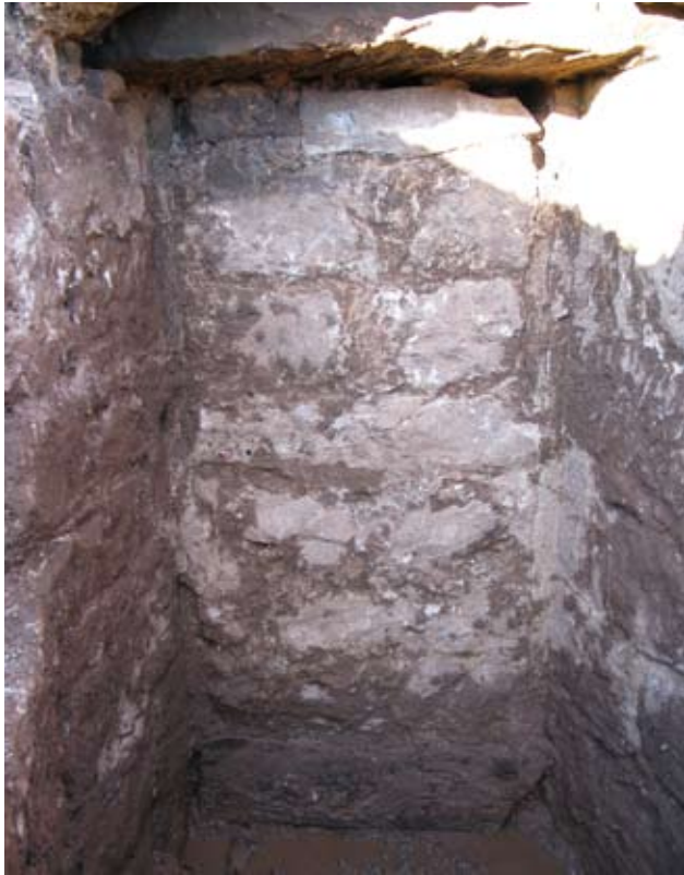
Fig. 21 Detail of basement door blocking
