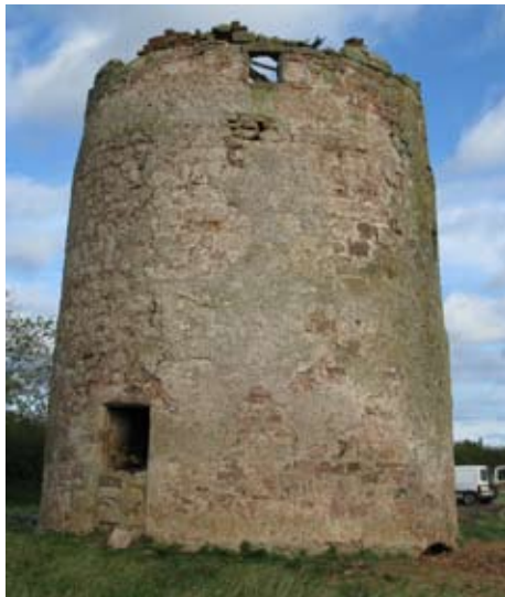
Fig.5 Exterior view of dovecote from the south-west
