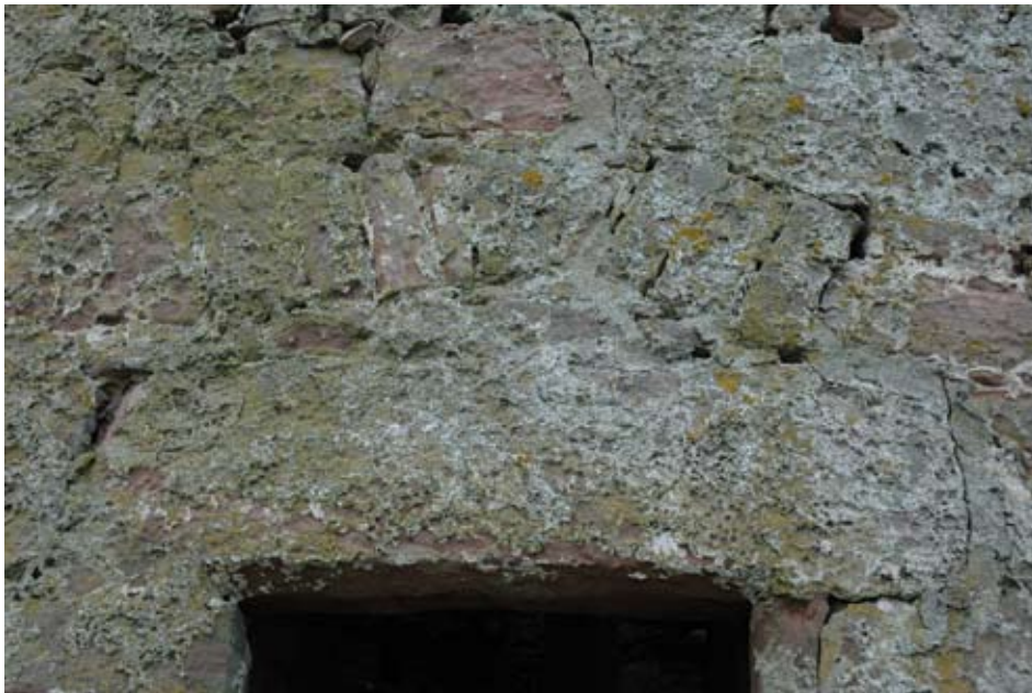
Fig. 7 Relieving arch and lintel detail, main entrance
