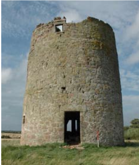
Fig.3 Exterior view of dovecote from the east
