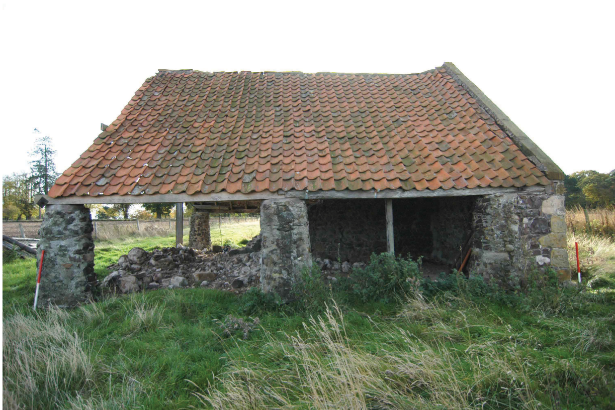
Plate 2. North-facing elevation of the barn
