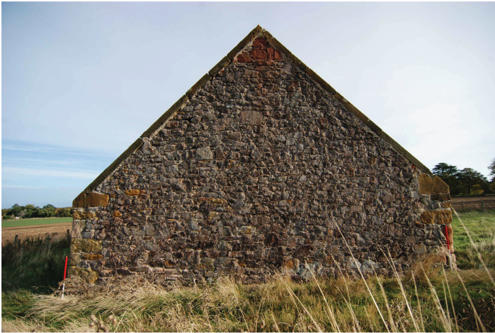
Plate 5. West-facing gable of the barn
