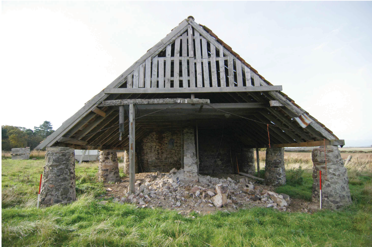
Plate 3. East-facing elevation of the barn
