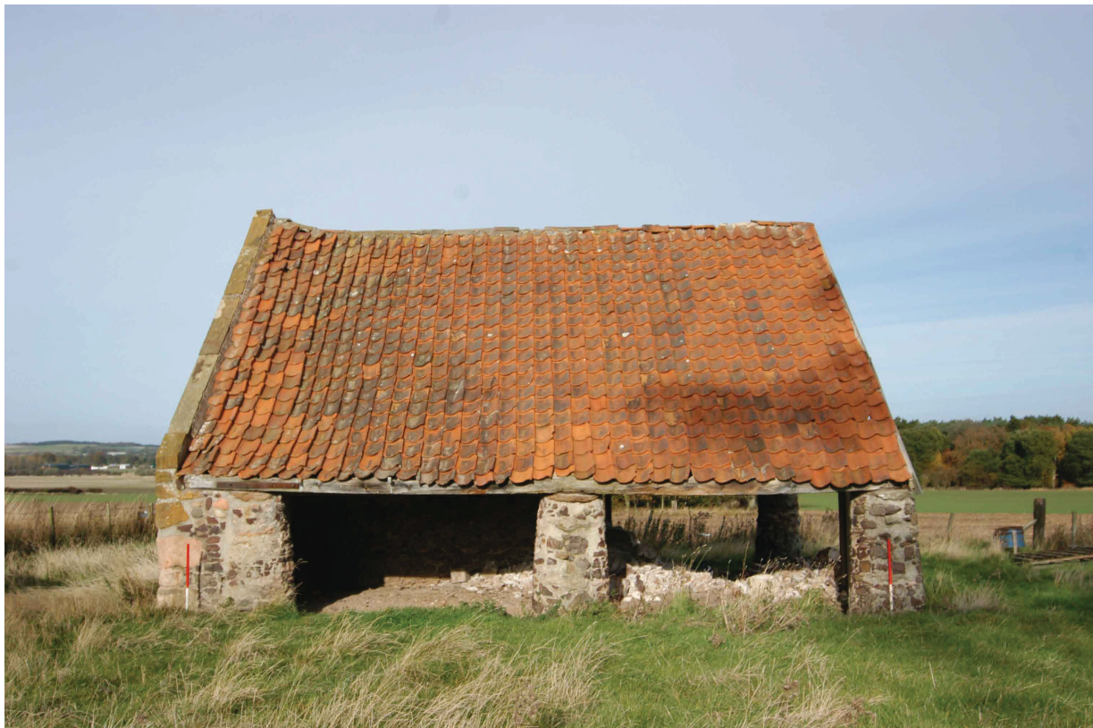
Plate 4. South-facing elevation of the barn
