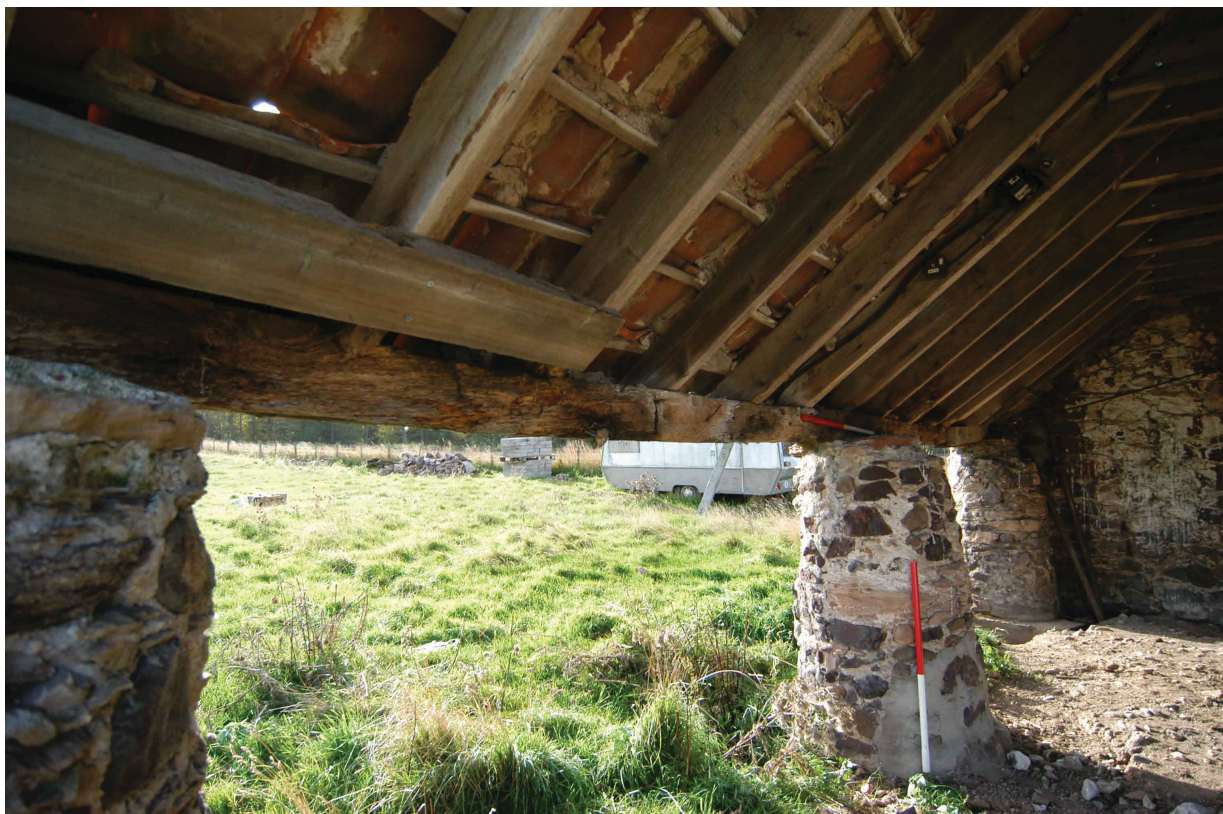
Plate 10. North-facing elevation, middle pier and wall plate
