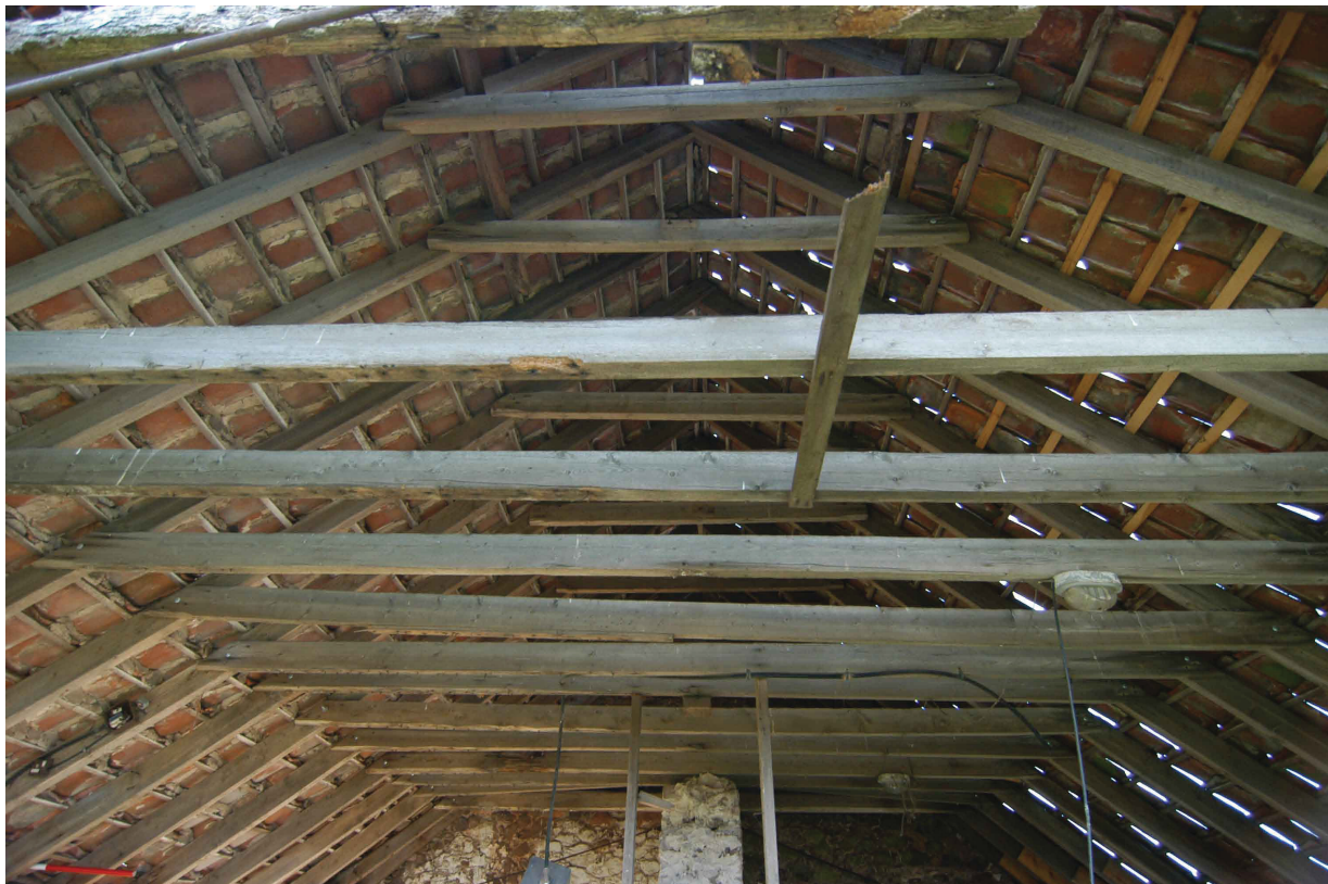
Plate 9. General view of the A-frame roof joists
