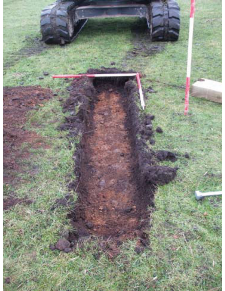
Figure 6 - Anchor Pit 3 excavated to natural subsoil
