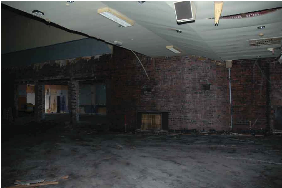
Fig. 6 Interior of main hall (Unit 1) east elevation
