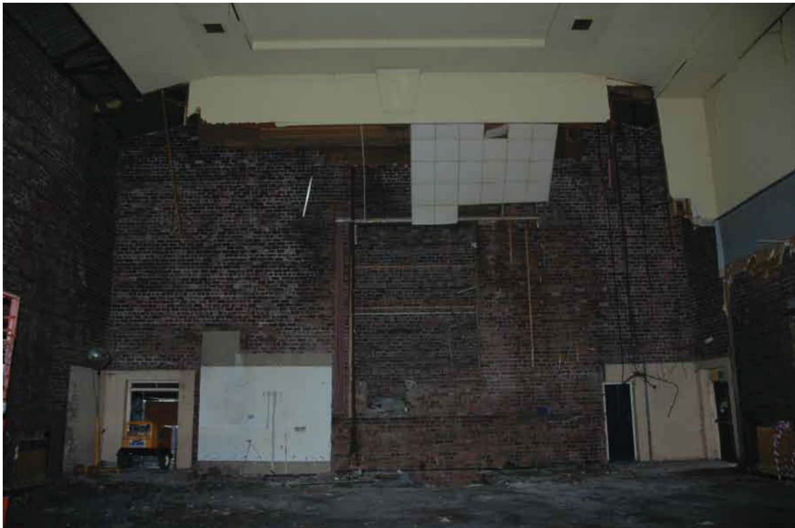
Fig. 5 Interior of main hall (Unit 1) north elevation
