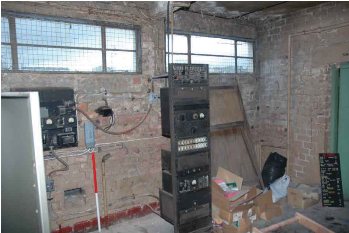
Fig. 21 View inside projector room (Unit 16)
