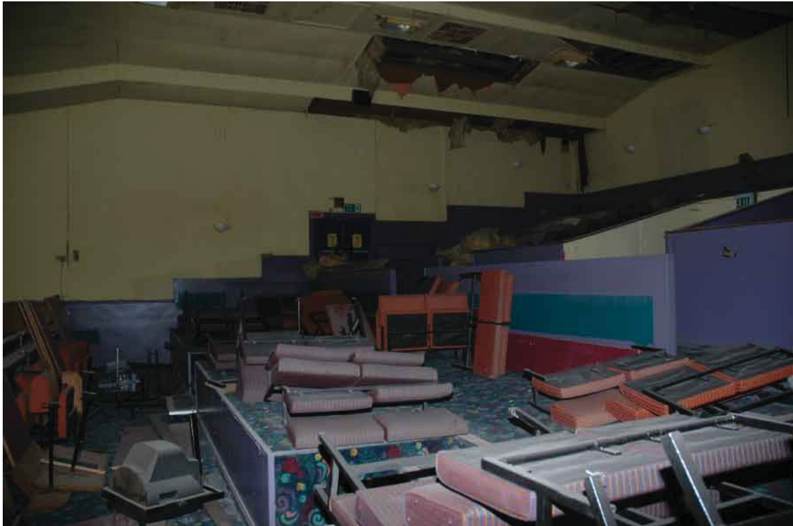
Fig. 14 General view of balcony (Unit 1)
