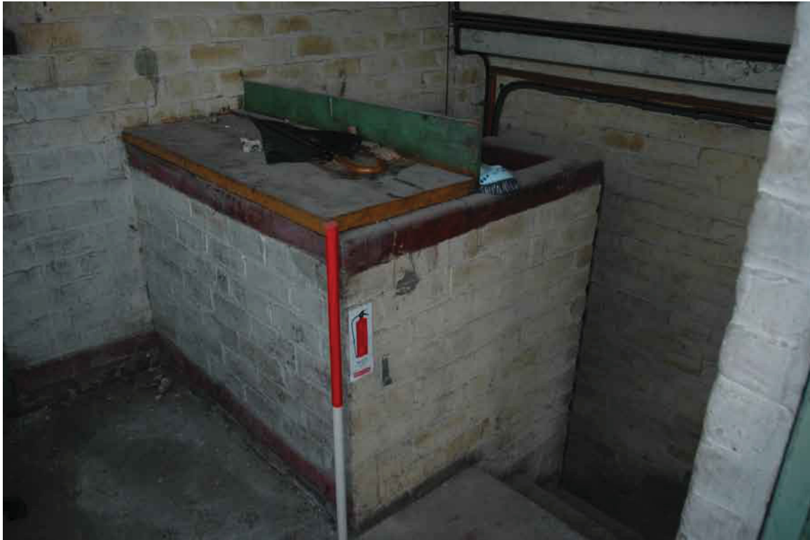
Fig. 18 Second floor landing (Unit 15)
