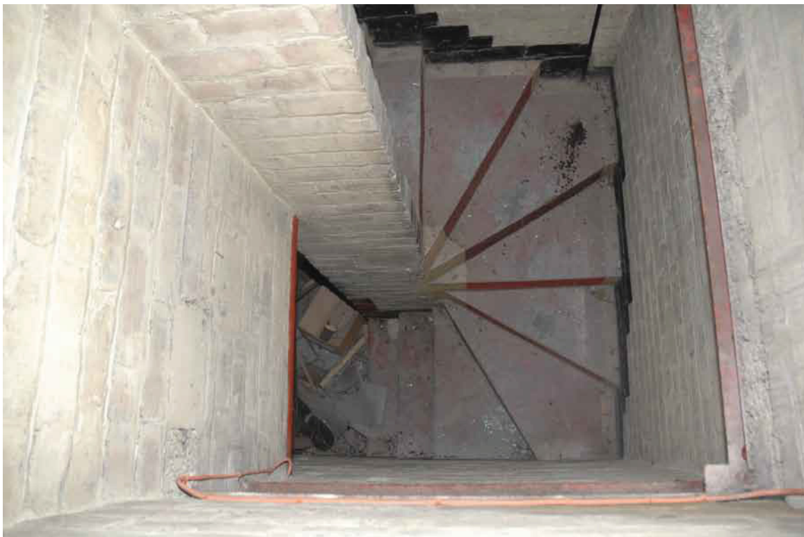
Fig. 19 View down stairwell (Unit 17) from second floor landing (Unit 15)
