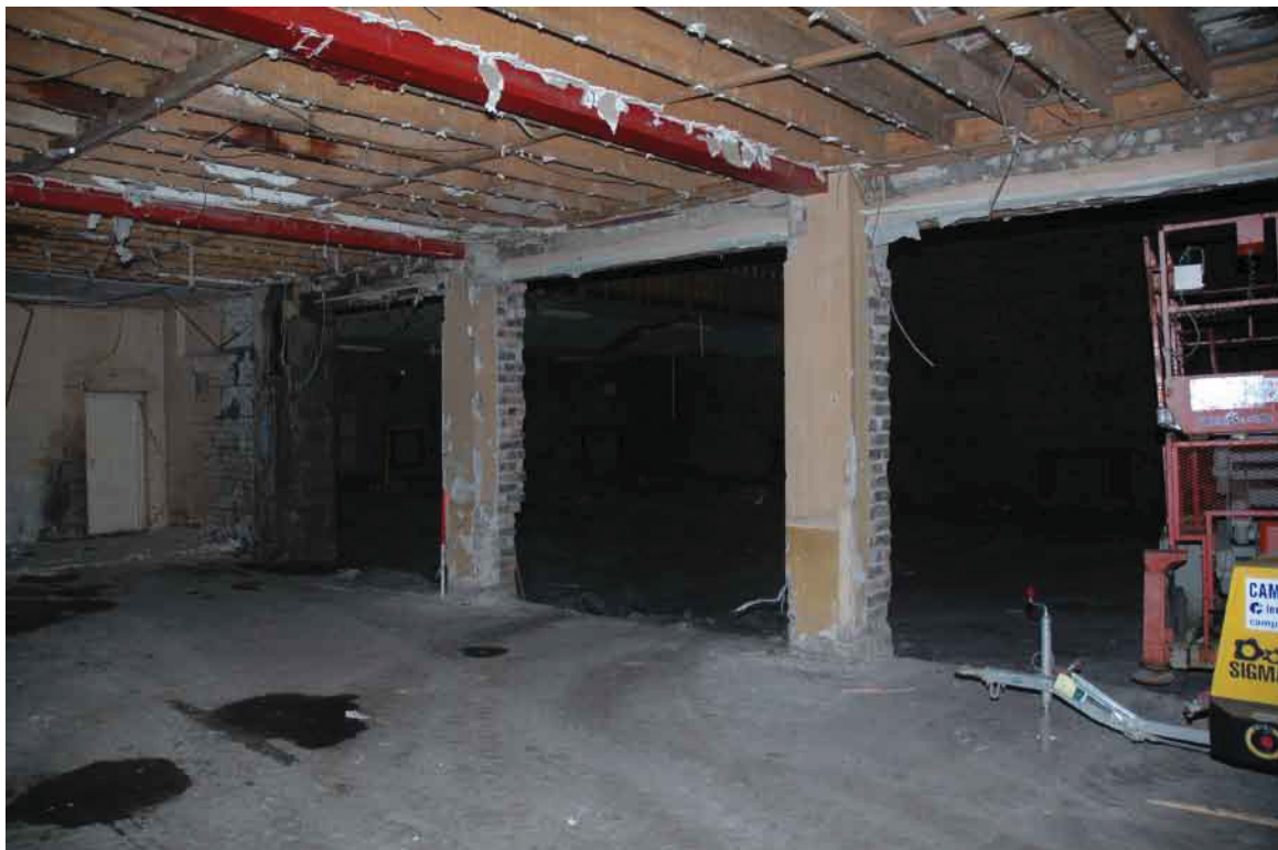
Fig. 11 General view of (Unit 2)
