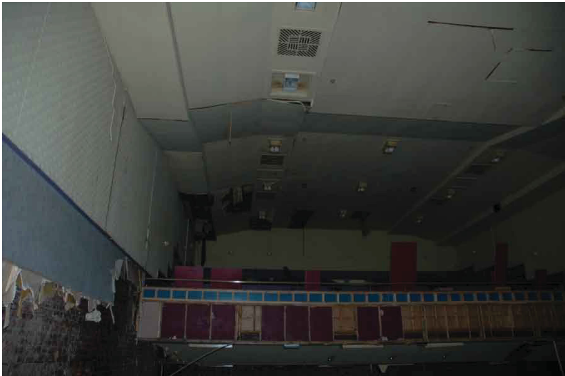
Fig. 8 General view of ceiling in main hall (Unit 1)
