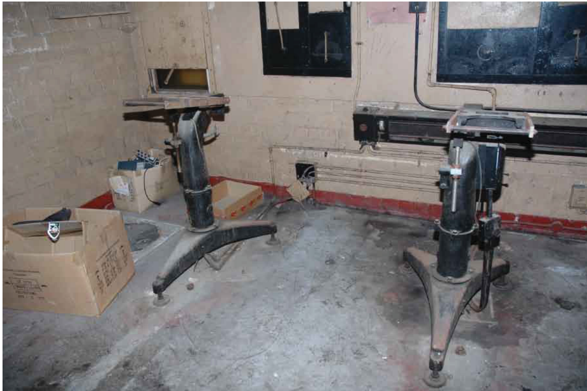
Fig. 22 View inside projector room (Unit 16)
