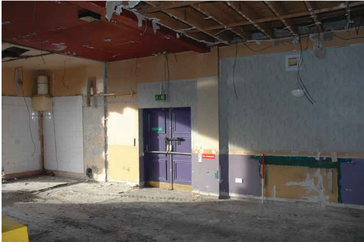
Fig. 10 General view of (Unit 2)
