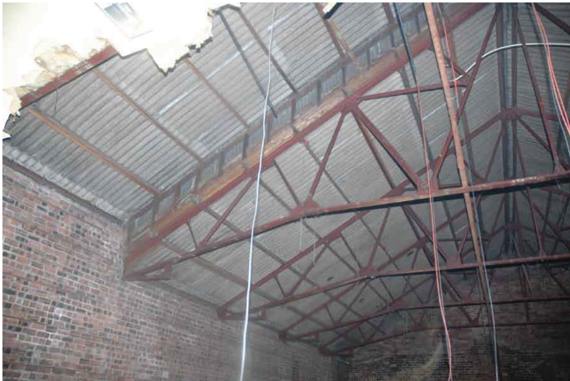
Fig. 26 View of roof structure (Unit 20)
