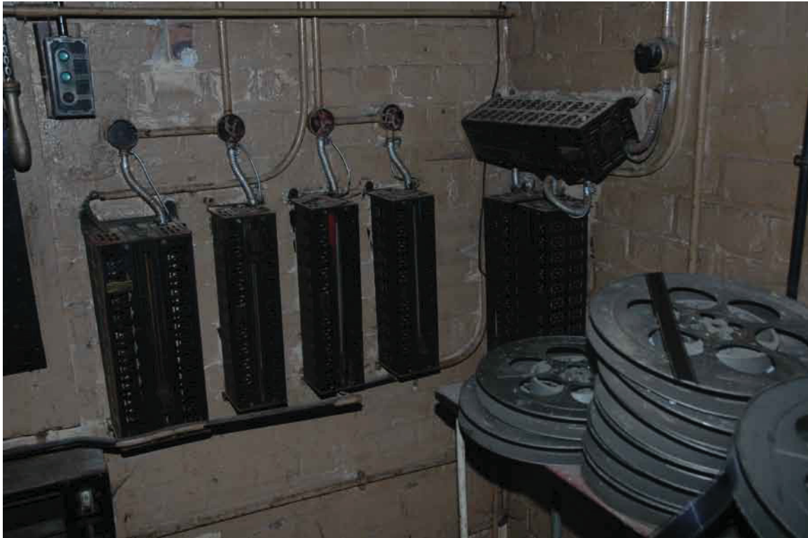
Fig. 24 View inside projector room (Unit 16)
