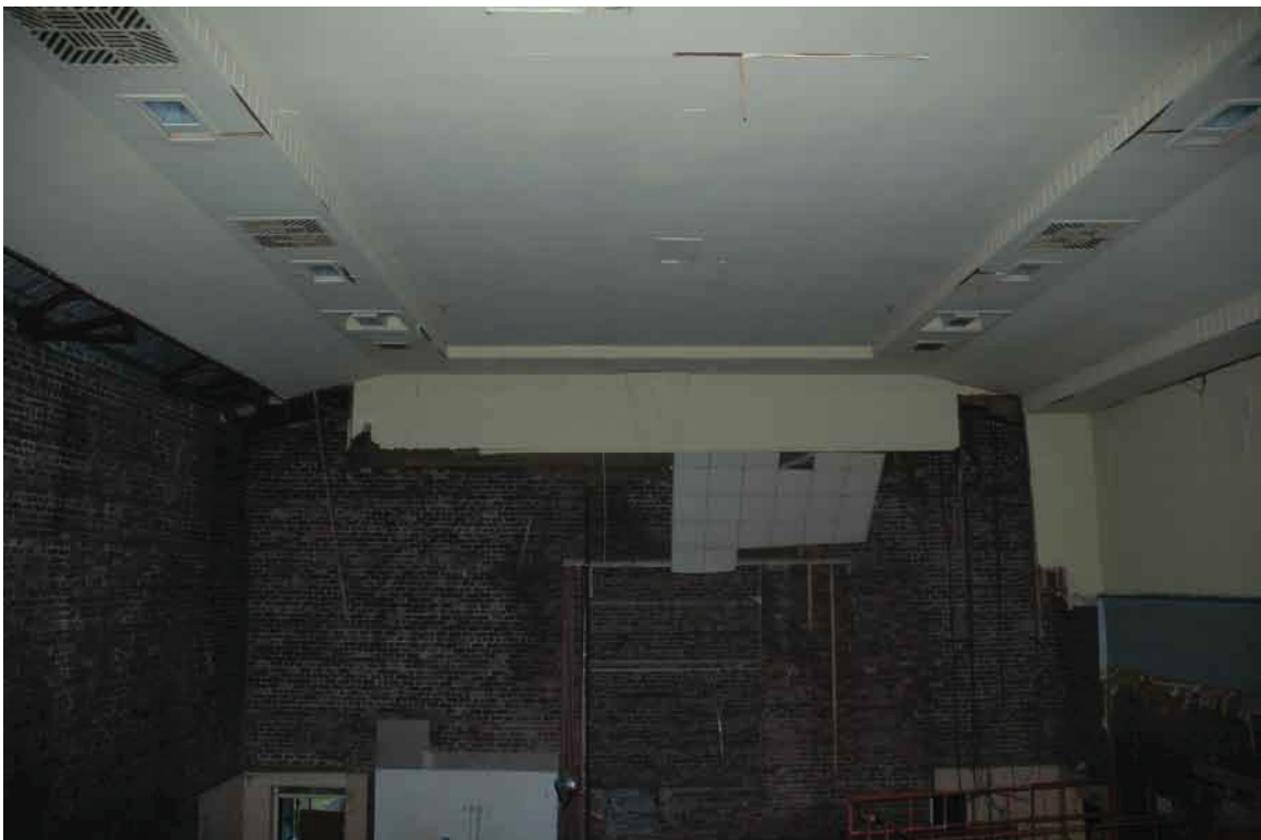
Fig. 9 General view of ceiling in main hall (Unit 1)
