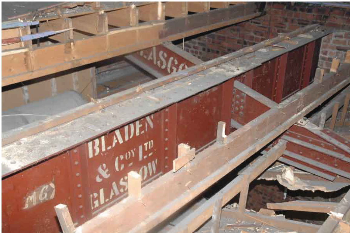
Fig. 27 View of girders within balcony structure (Unit 1)
