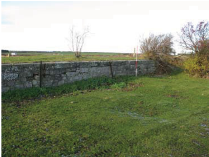
Fig. 11 - View of railway platform (Position 18)
