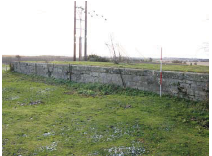
Fig. 10 - View of railway platform (Position 17)
