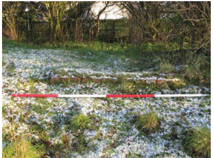
Fig. 12 - Brick structure in situ on embankment (Position 21)
