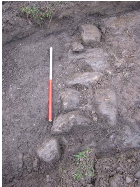
Fig. 4 Wall footing remains (2201)
