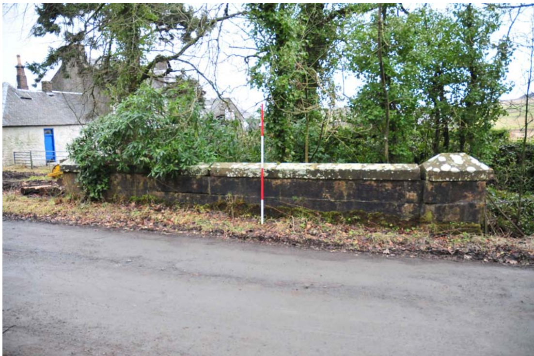
Fig. 5 General view of parapet
