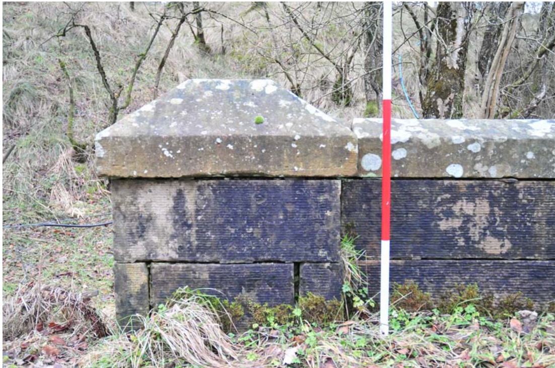
Fig. 3 Detail of pier and parapet capstones
