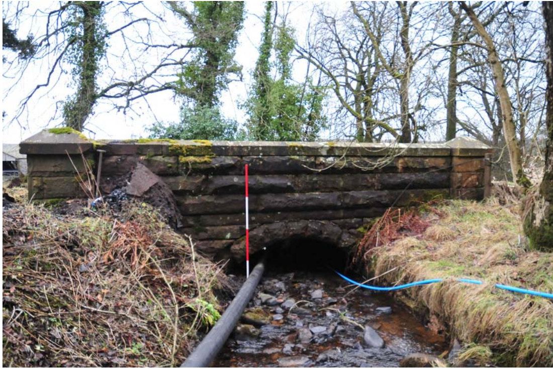
Fig. 6 NW elevation of bridge
