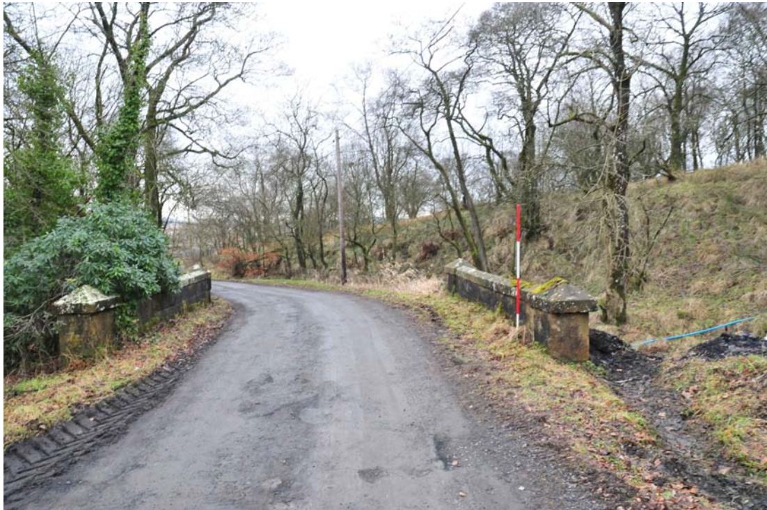
Fig. 2 View of bridge from the road
