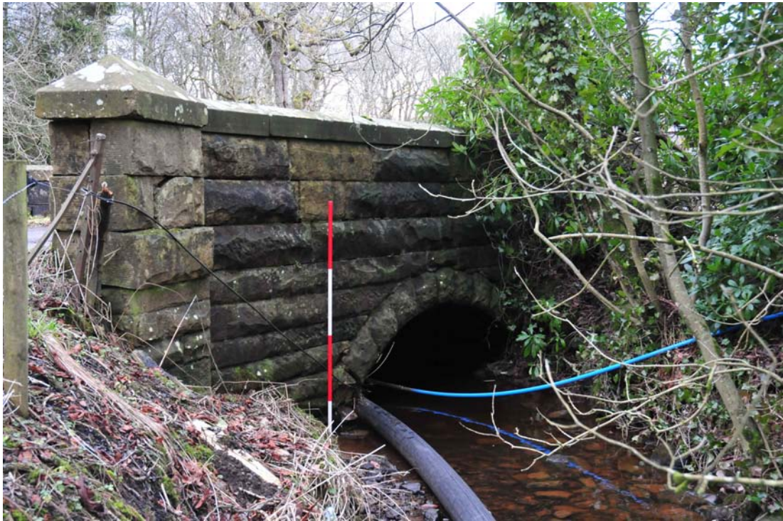
Fig. 9 General view of bridge
