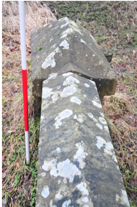
Fig. 4 Detail of pier and parapet capstones
