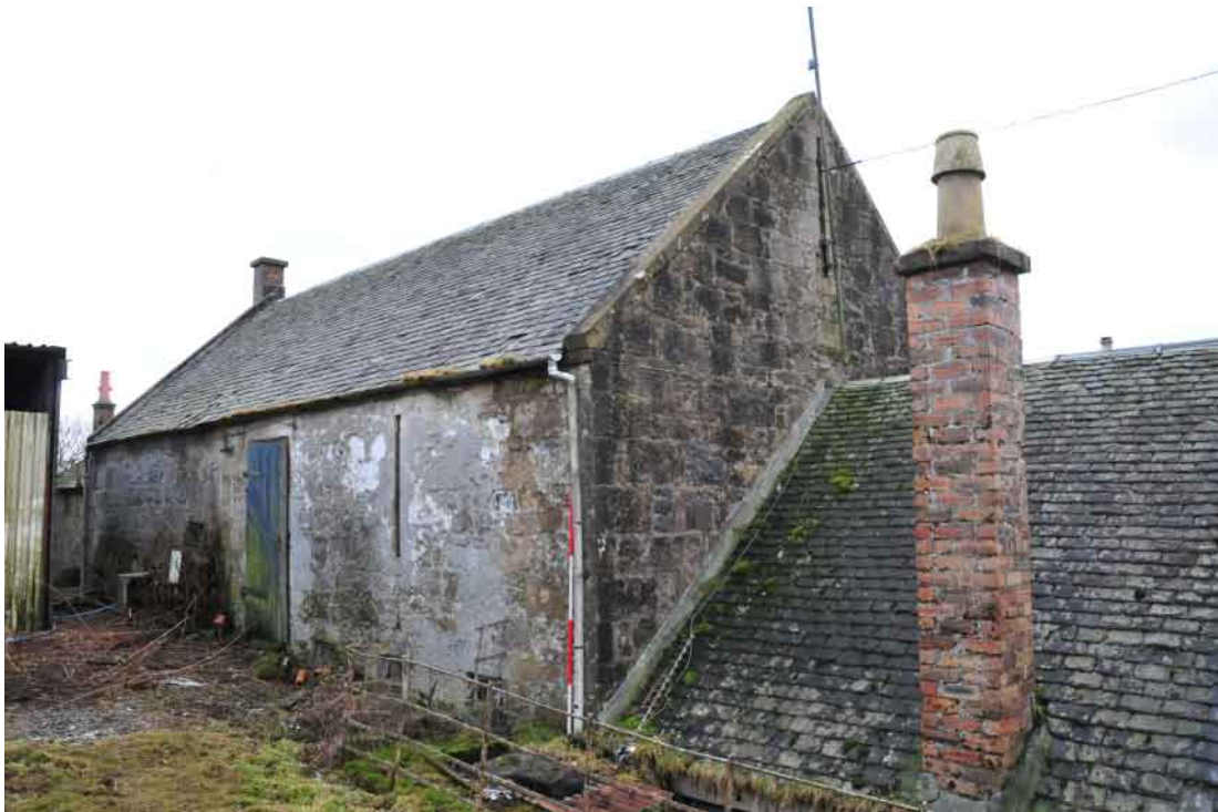
Fig. 22 Building 4 from the north
