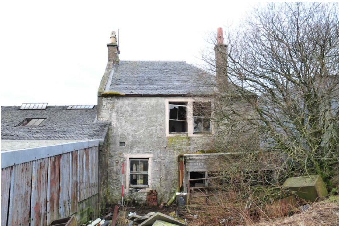
Fig. 26 Building 5 exterior from the south east
