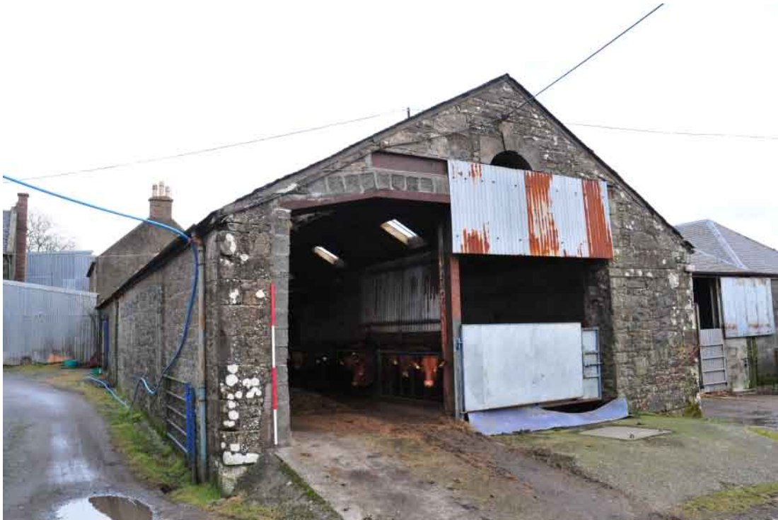
Fig. 29 Building 6 exterior from the south west
