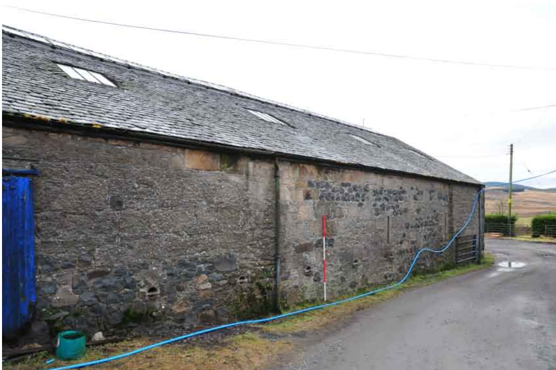
Fig. 30 Building 6 exterior from the north
