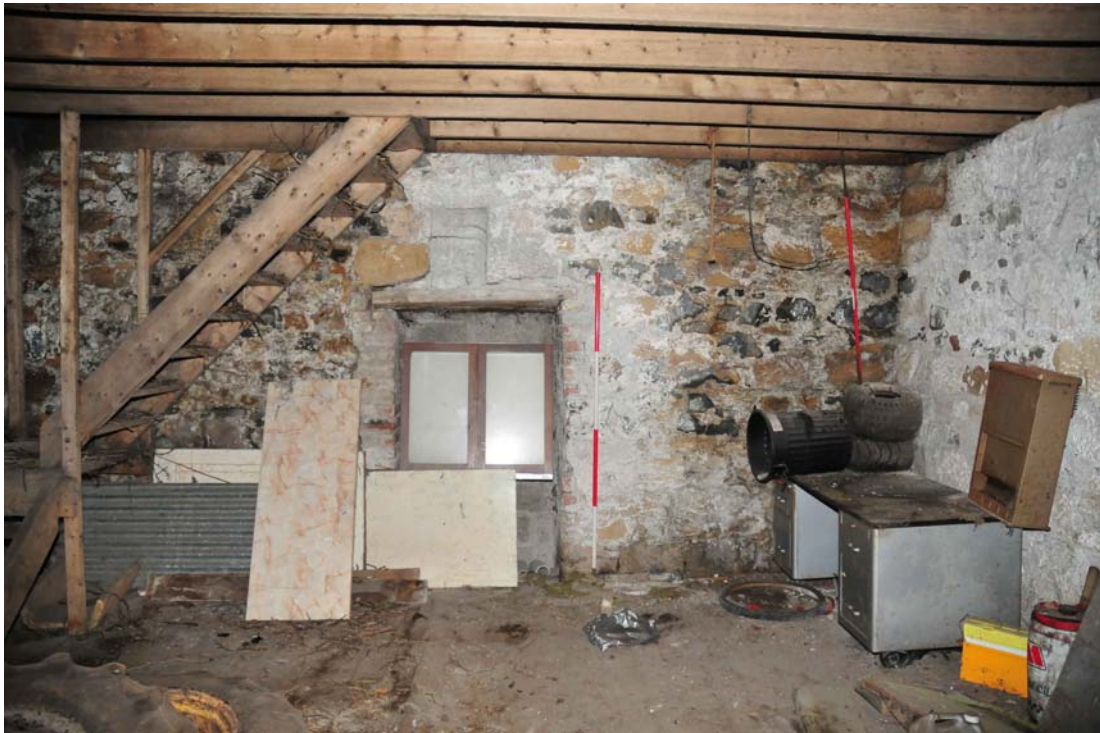
Fig. 25 Building 4 interior first floor blocked pitching window
