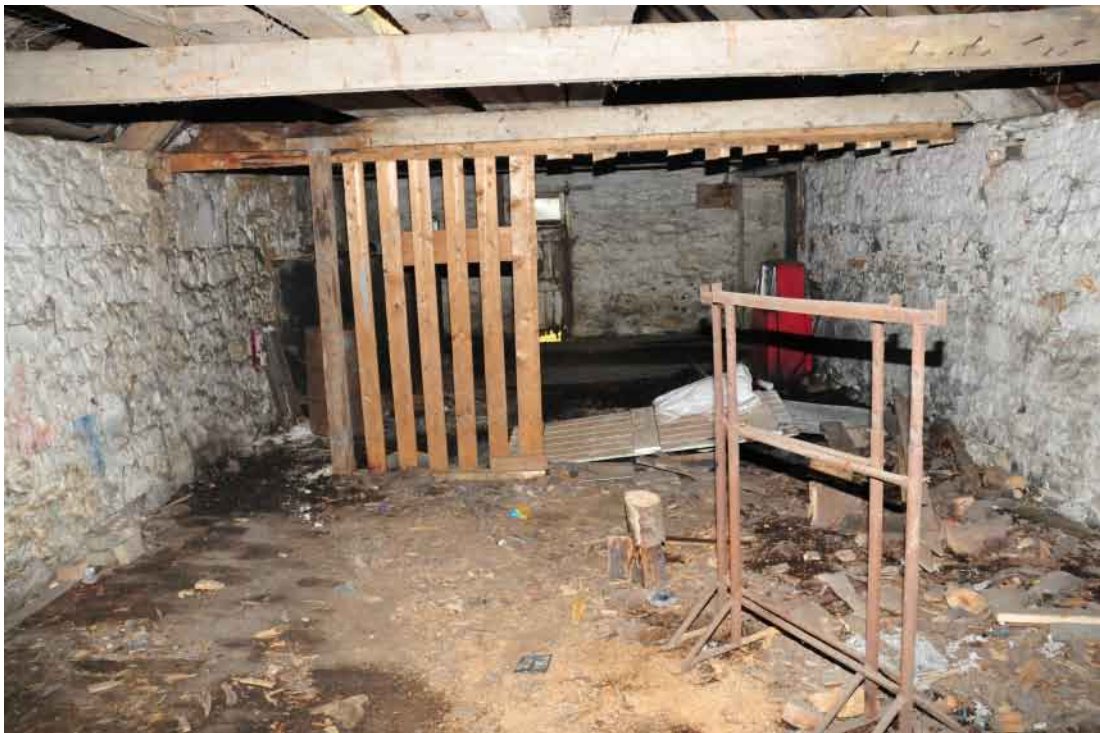
Fig. 16 Building 2 interior, Out building 2
