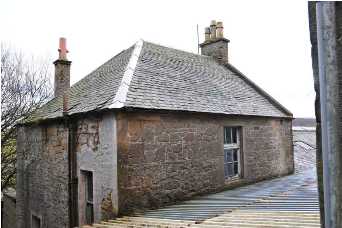
Fig. 27 Building 5 exterior from the north
