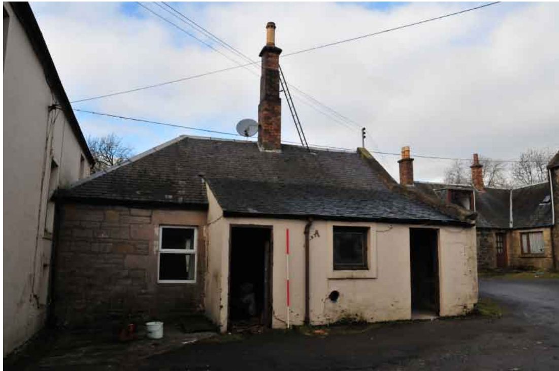
Fig. 11 Building 1 rear extension from the south east
