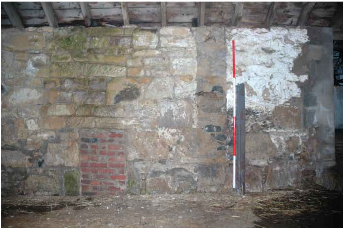
Fig. 36 Building 7 interior detail of blocked hatch and partition mark
