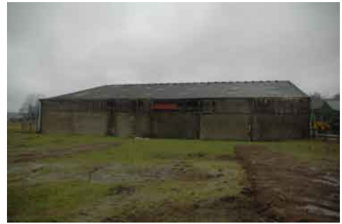
Shed 3, SE elevation
