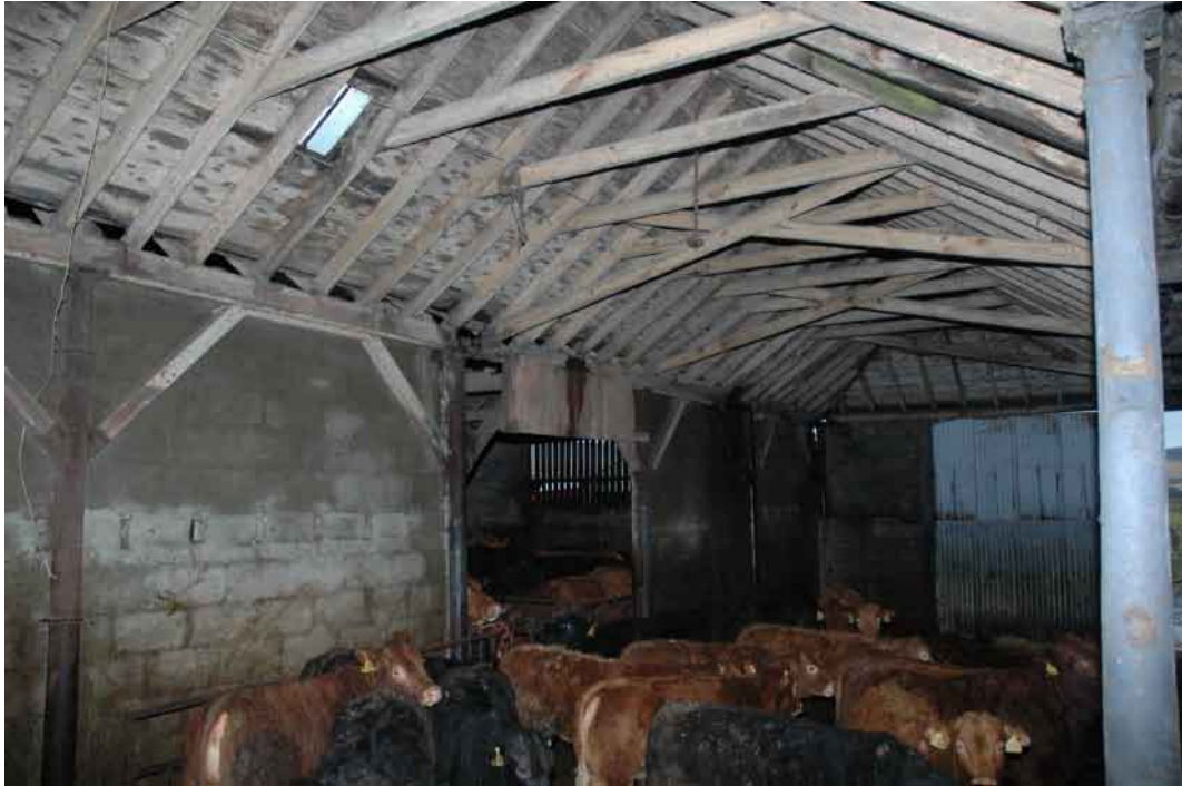
Fig. 37 Shed 1, detail of Victorian pillars and roof truss
