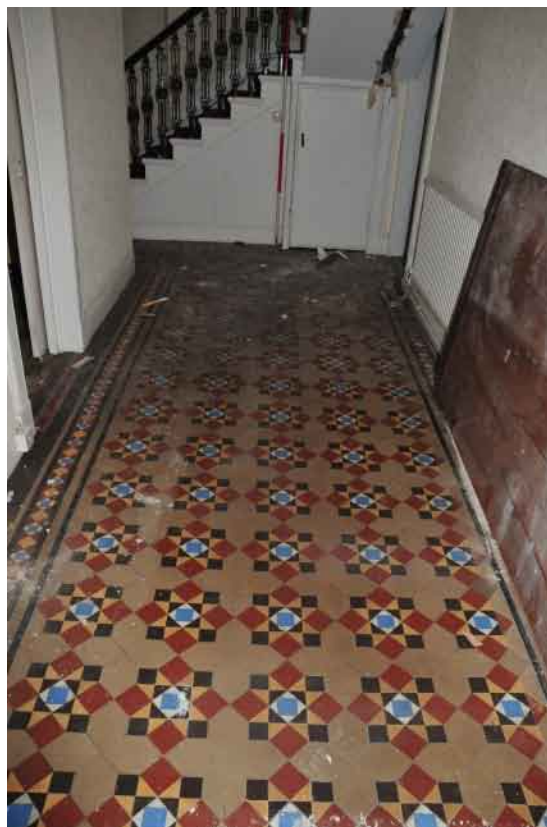
Fig. 12 Building 1 interior, ground floor hallway floor
