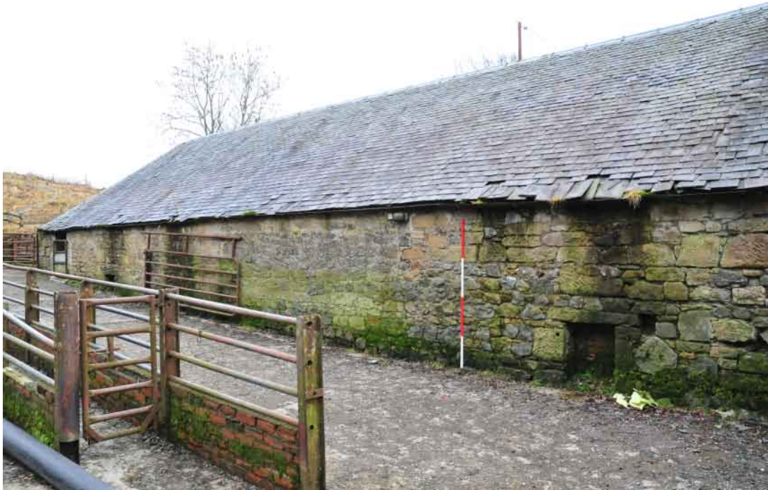
Fig. 35 Building 7 exterior from the west
