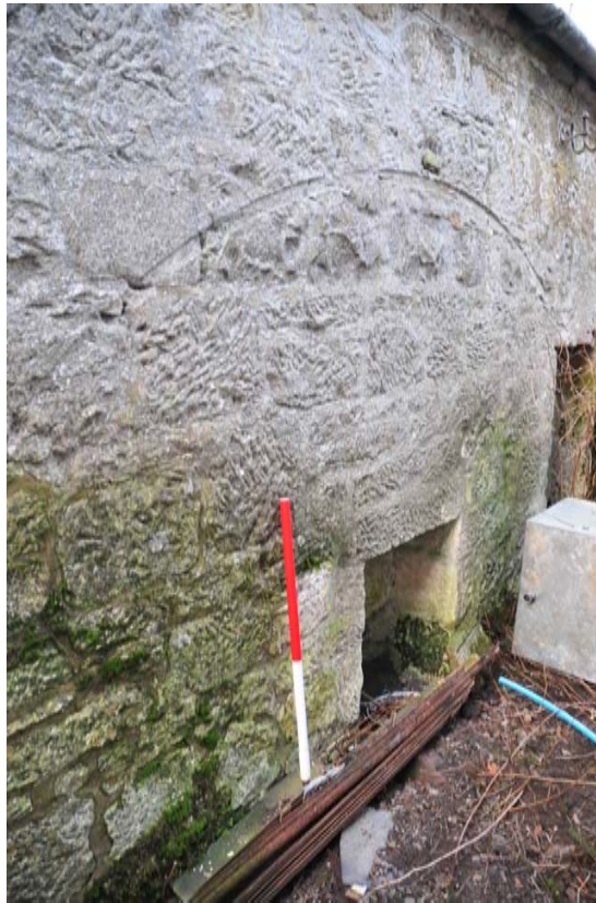
Fig. 23 Building 4, water wheel rim wheel scar and axle box
