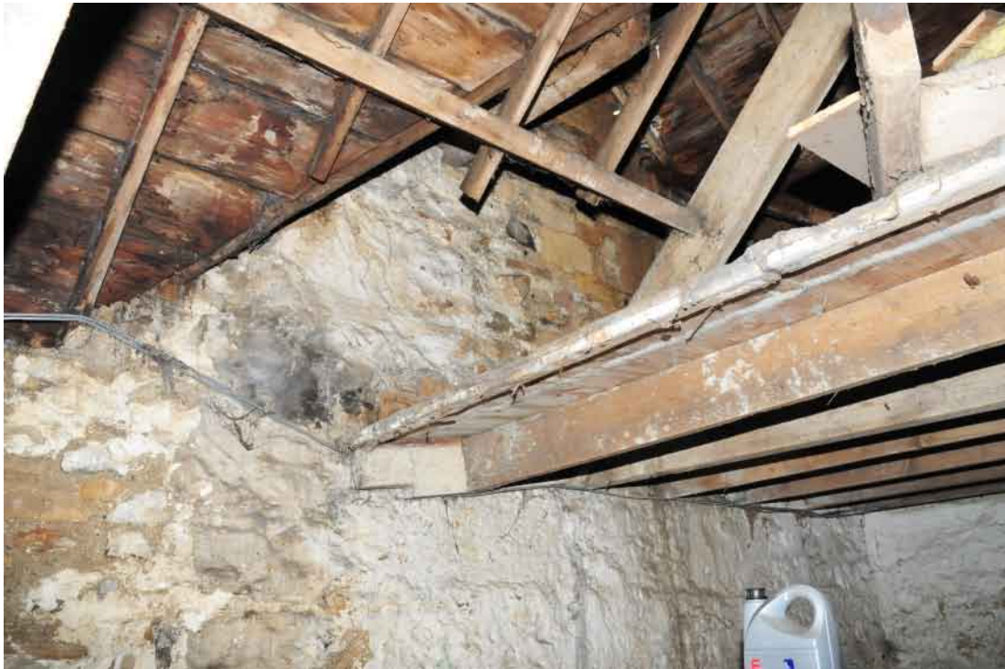
Fig. 17 Building 2 interior of out building 1 and 2, roof junction
