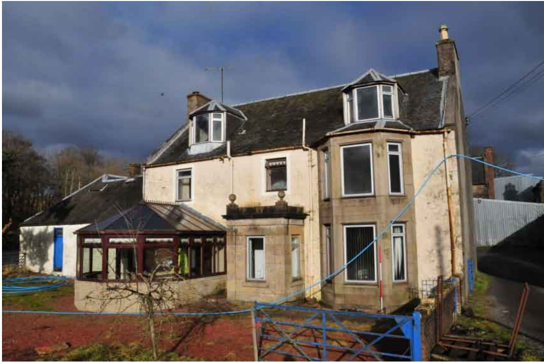
Fig. 9 Building 1 from the south
