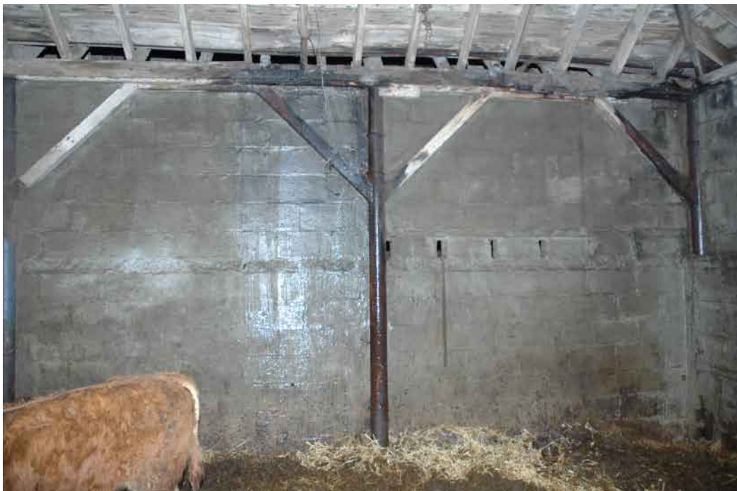
Fig. 38 Shed 1, detail of Victorian pillars and roof truss
