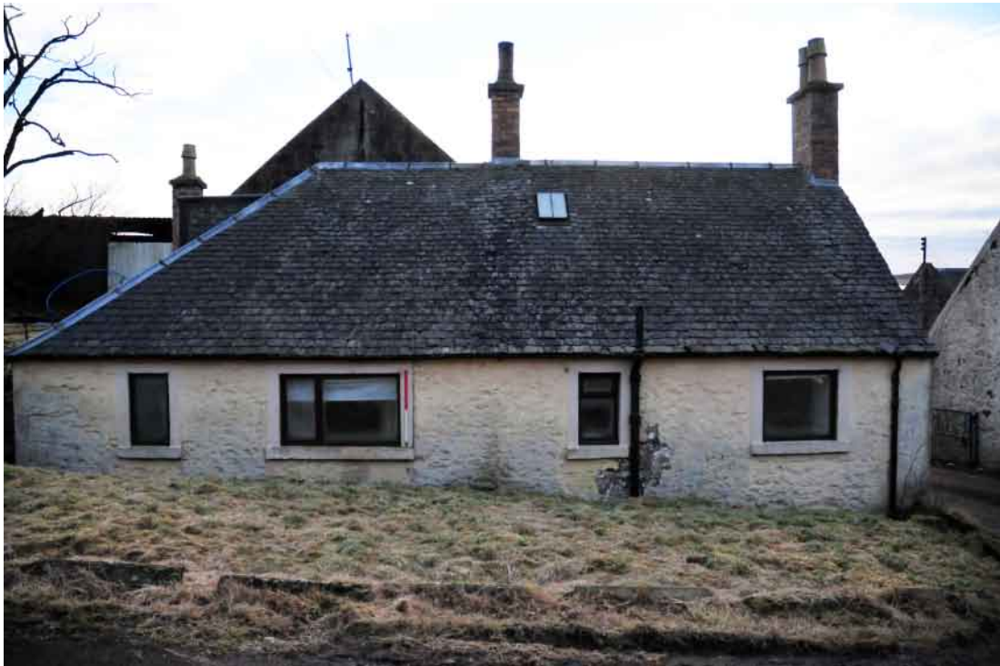
Fig. 19 Building 3 from the north-west
