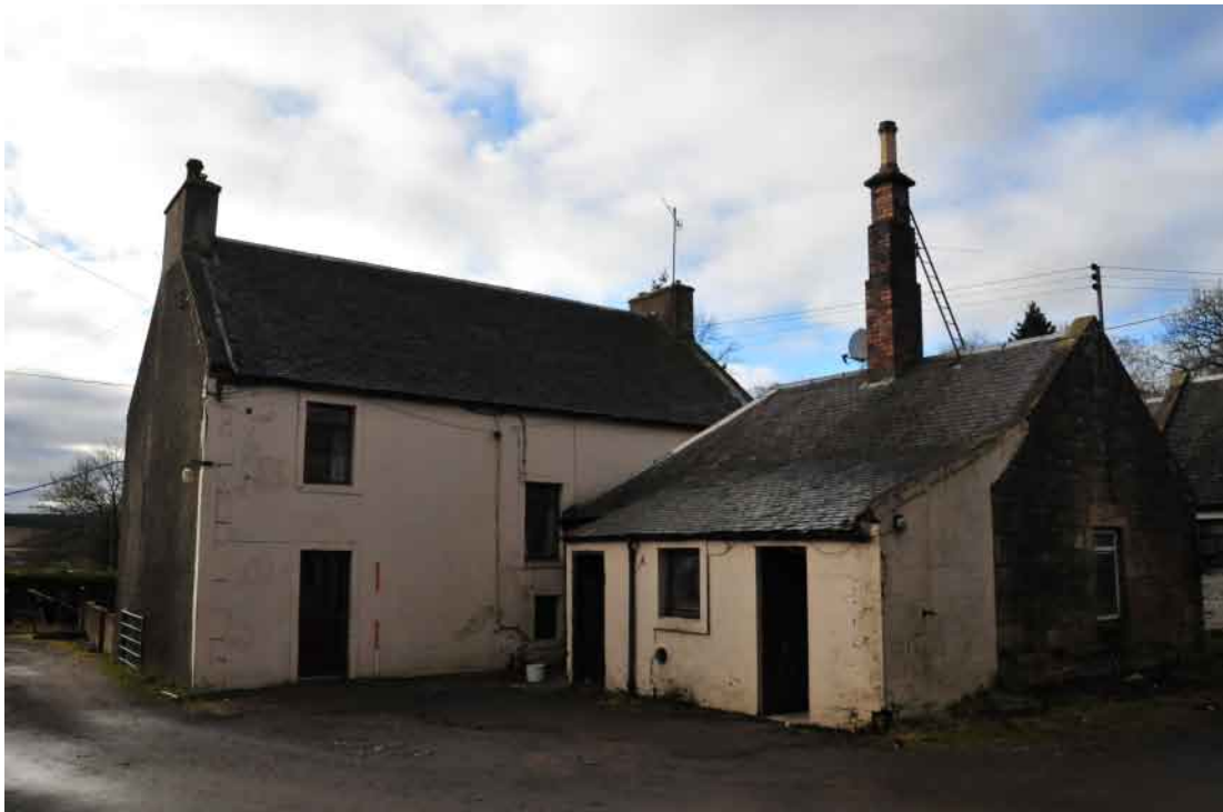
Fig. 10 Building 1 from the east
