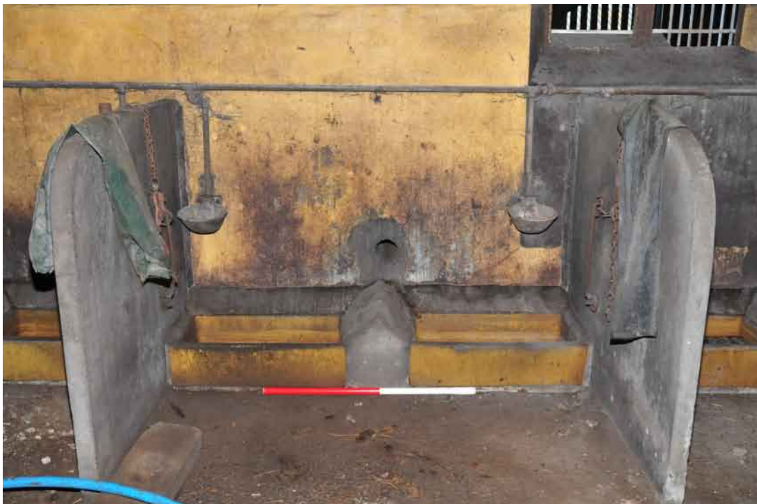
Fig. 32 Building 6 interior of rearing room stalls
