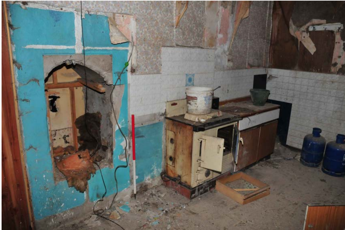
Fig. 13 Building 1 interior of extension kitchen
