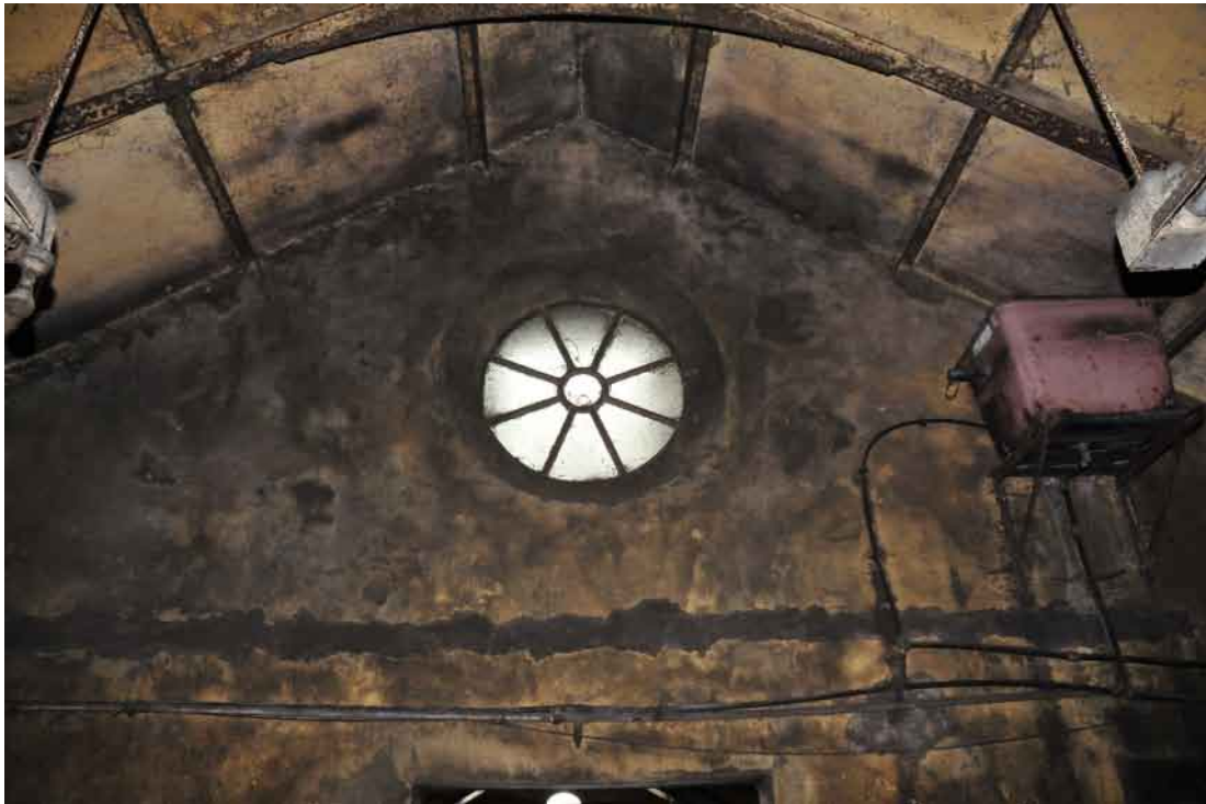
Fig. 31 Detail of oculus within the south-west facing gable of Building 6
