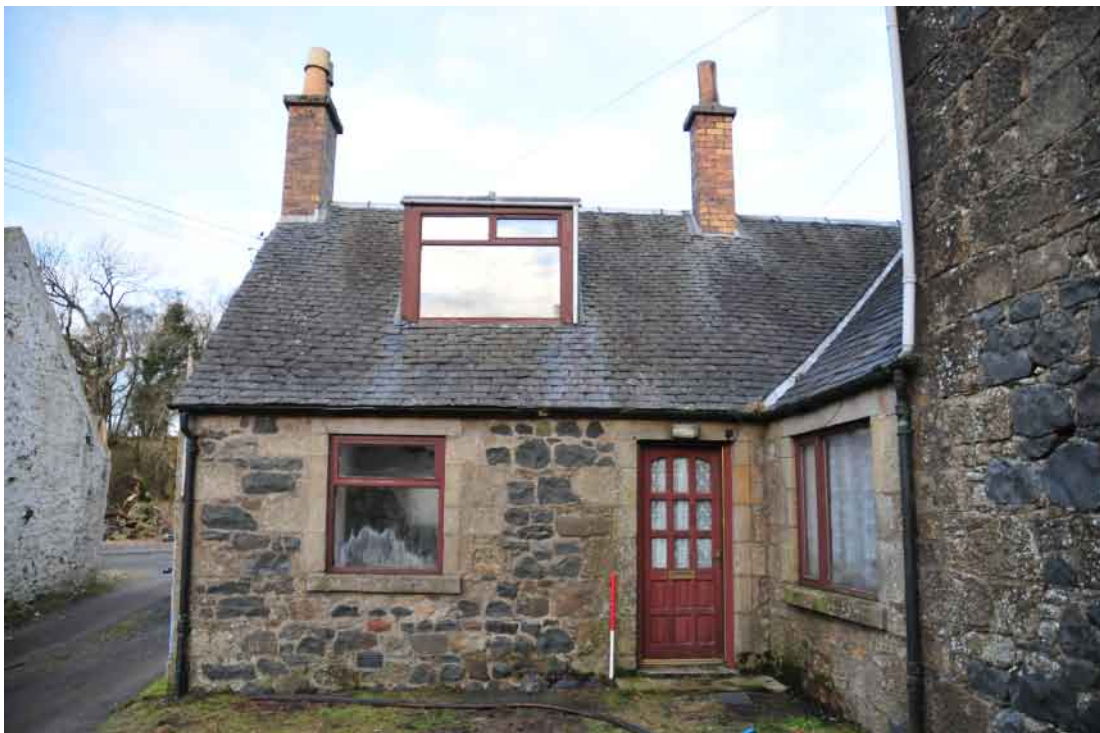
Fig. 18 Building 3 from the south-east
