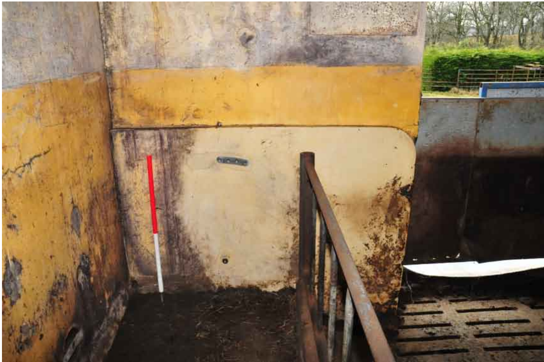
Fig. 33 Building 6 interior, detail of ceramic-coated milking stall
