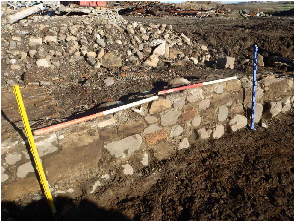
Fig. 6 Wall 006 from the south-west
