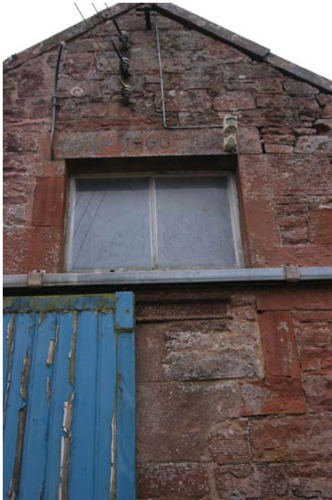
Plate 19-Building 5, north-east facing gable, with 1866 date on the lintel
