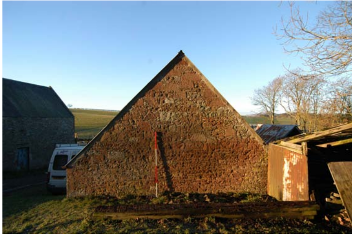
Plate 9-Building 3, south-east facing gable
