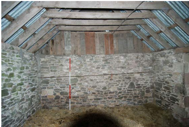
Plate 7 - Building 2, Unit 1, southwest-facing elevation, partition wall
