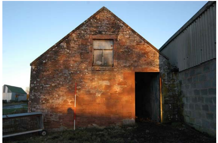
Plate 20-Building 5, south-east facing gable
