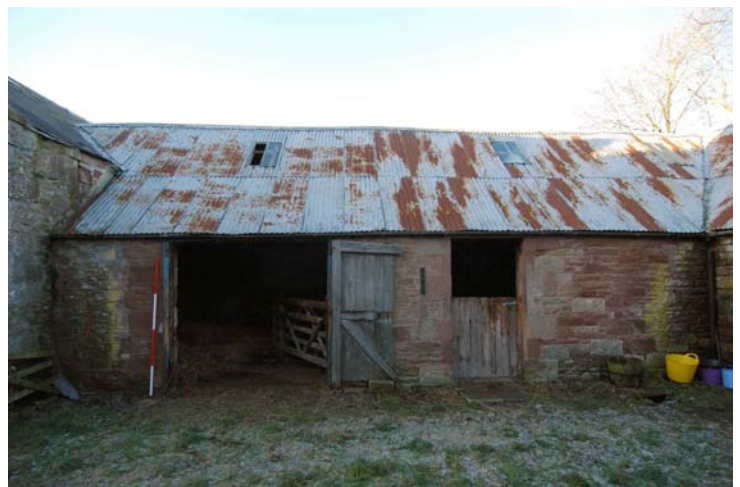
Plate 4 - Building 2, Unit 1, northeast-facing elevation with blocked loft windows
