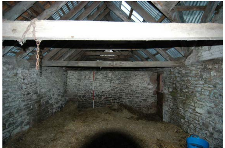
Plate 8 - Building 2, Unit 3, north-facing elevation and roof truss tie-beams
