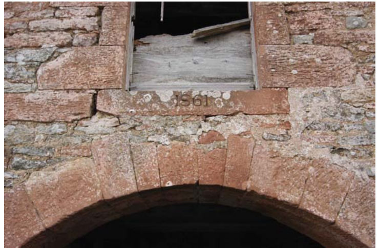
Plate 2 - Building 1, south-west facing elevation, sill with a date stone of 1861
