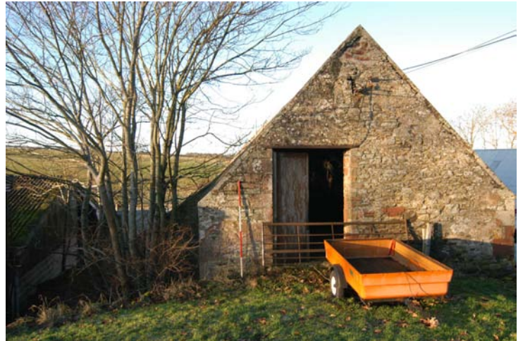
Plate 14-Building 4, south-east facing gable
