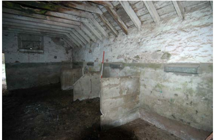
Plate 22-Building 5, general shot of the stalls at the south-west end
