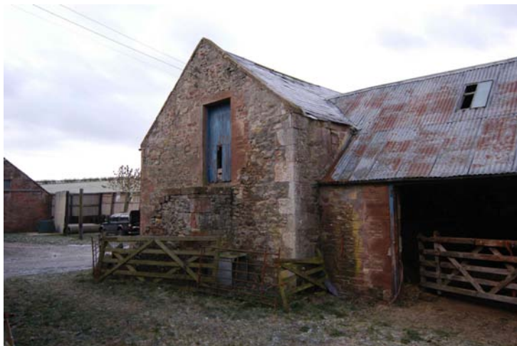
Plate 3 - Building 1, south-east facing gable
