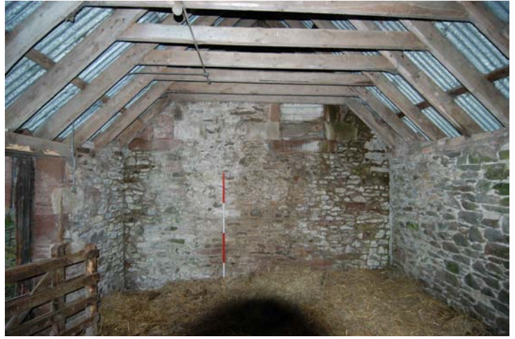
Plate 6 - Building 2, Unit 1, northeast-facing elevation with blocked loft windows
