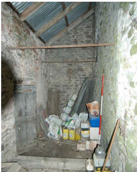
Plate 17-Building 4, interior of rear outshot building, roof detail
