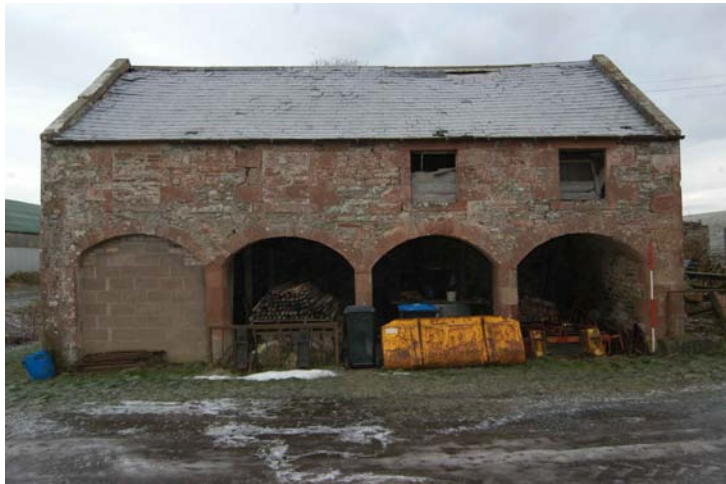
Plate 1 - Building 1, south-west facing elevation
