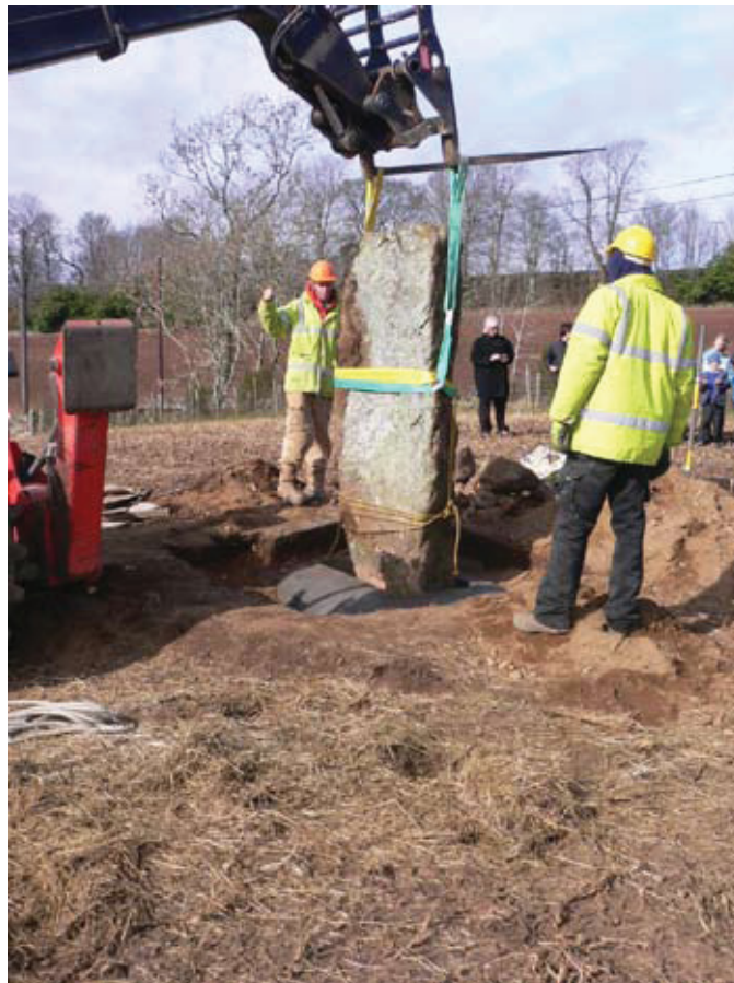
Fig. 16 - Manoeuvring the stone into the concrete sleeve
