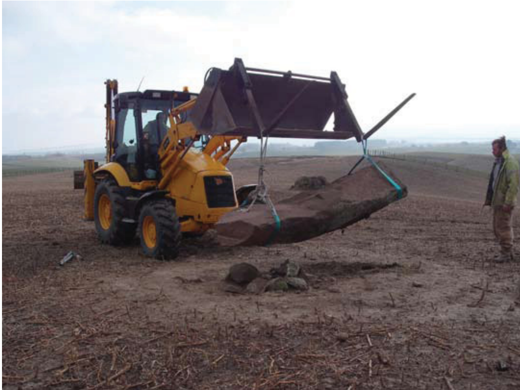
Fig. 4 - Stone being moved prior to excavation
