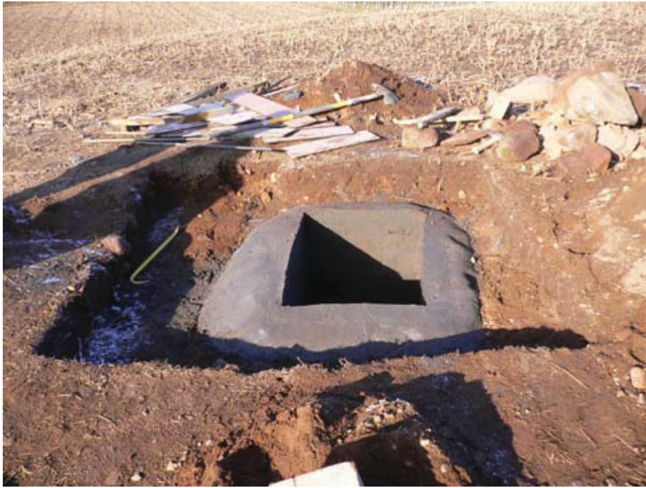
Fig. 15 - Prepared concrete socket
