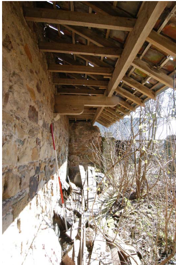
Plate 10 - Unit 14, cattle court feeding stall roof trusses and supporting timber
