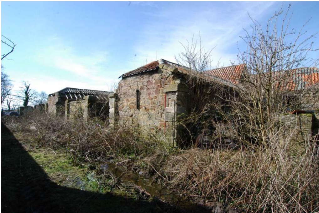
Plate 9 - Units 14 and 15 cattle courts with stall roofs in situ
