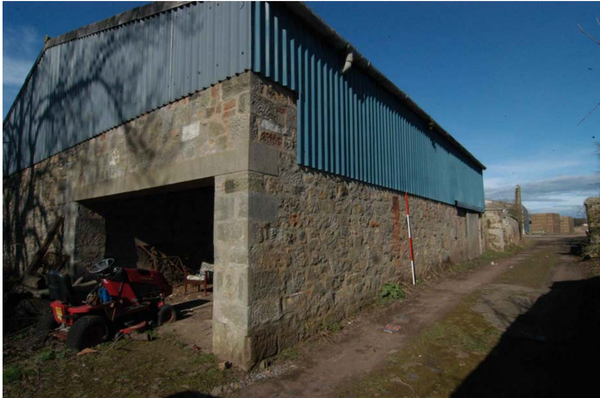
Plate 15 - Unit 22, steel-framed workshop
