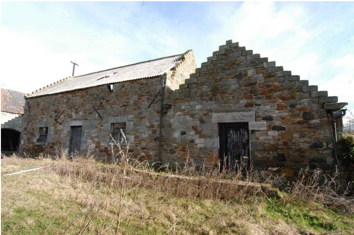
Plate 2 - Units 2 and 4 south-facing elevation
