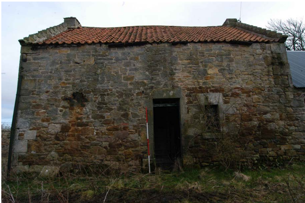
Plate 12 - Unit 16, farmhouse, south-facing elevation
