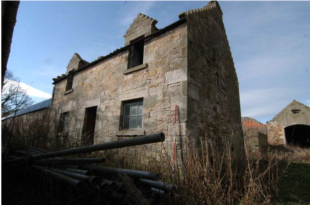
Plate 11 - Unit 16, farmhouse, east-facing elevation and crowstep gable
