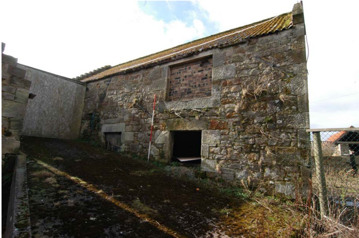
Plate 3 - Unit 4, north-facing elevation
