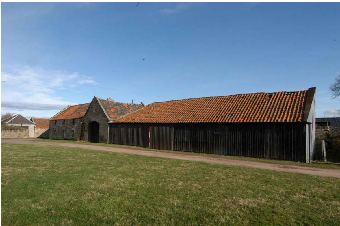
Plate 8 - Units 5-7 west-facing elevation
