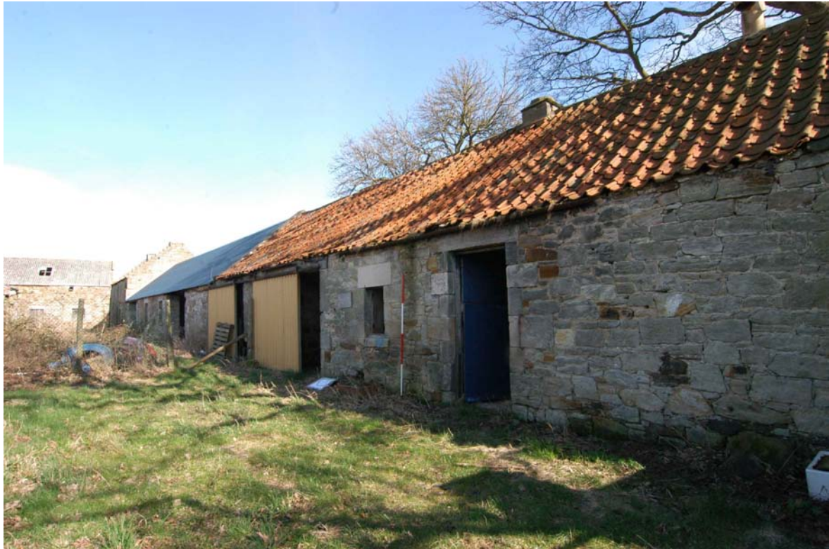
Plate 13 - Units 17-20, animal houses, west-facing elevation
