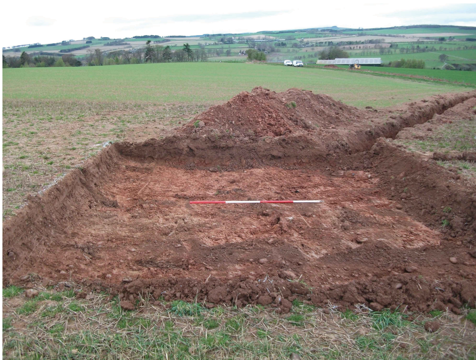
Fig. 3 Turbine Base 2 from the east
