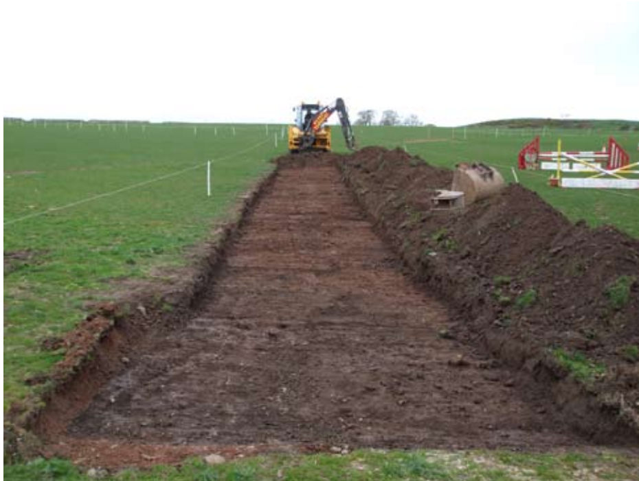
Fig. 2 Access track under excavation
