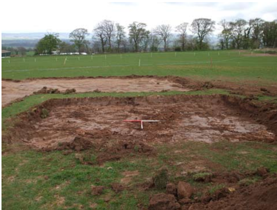
Fig. 3 Turbine Base 1 stripped to natural subsoil
