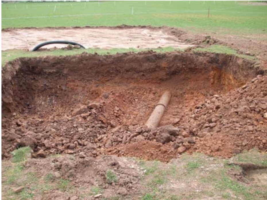
Fig. 4 Turbine Base 1 showing modern water main
