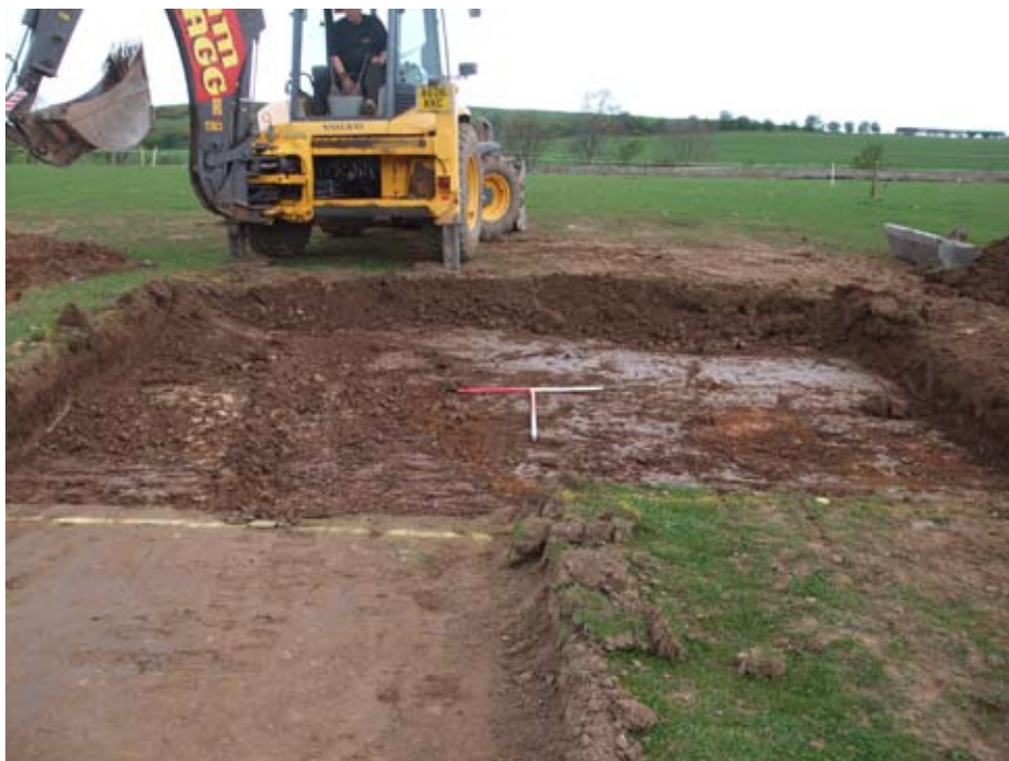
Fig. 5 Turbine Base 2 stripped to natural subsoil
