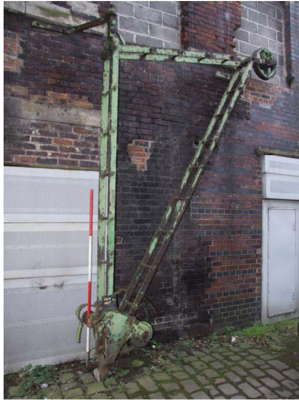
PLATE 5 Crane on Bank Place (scale: 2.0m).
