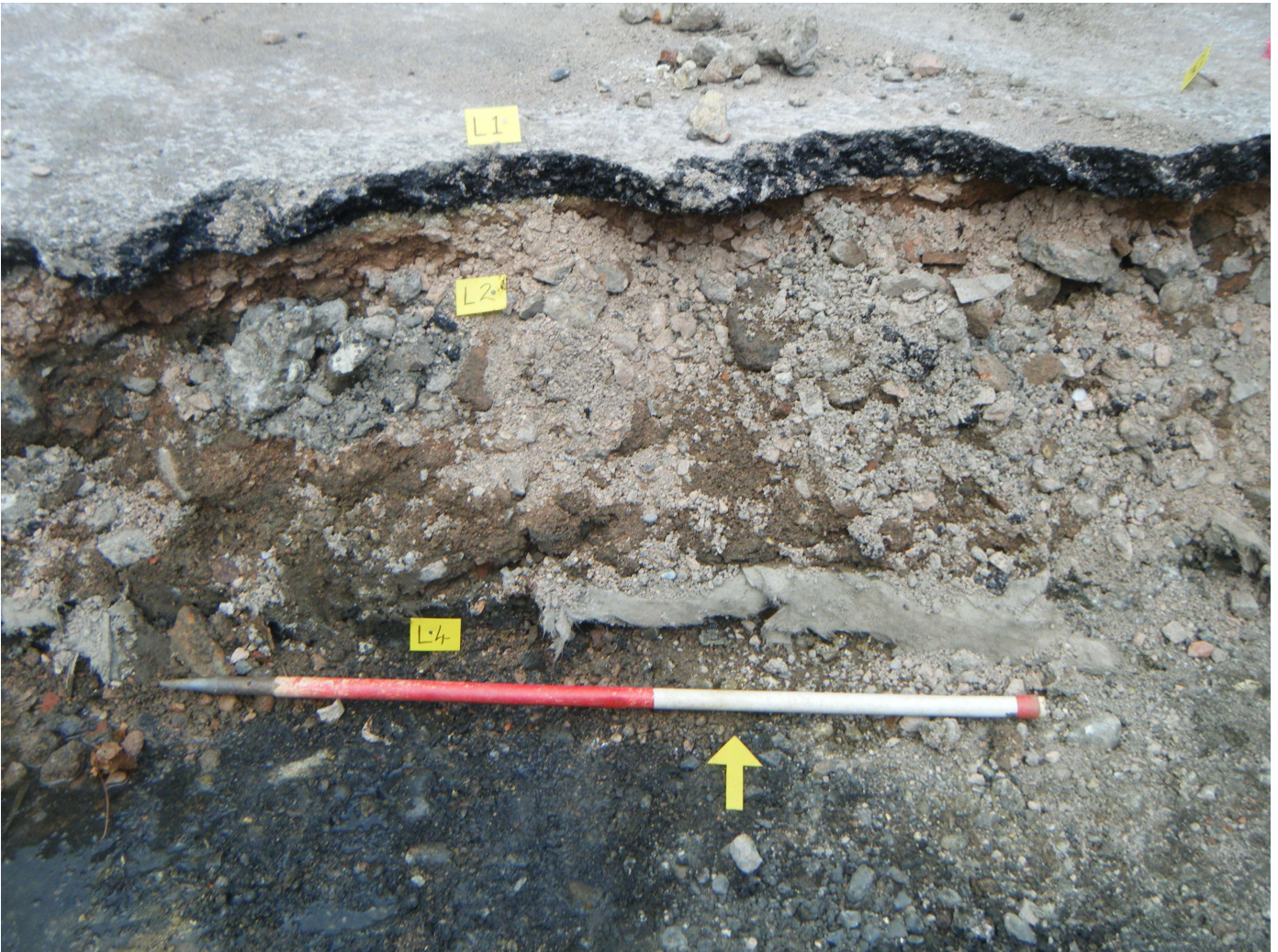
012 Trench rep sx west end view N Page 6/9
