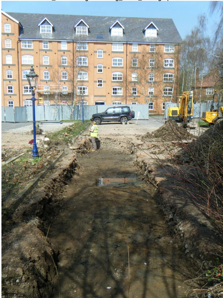
015 Trench shot view N
