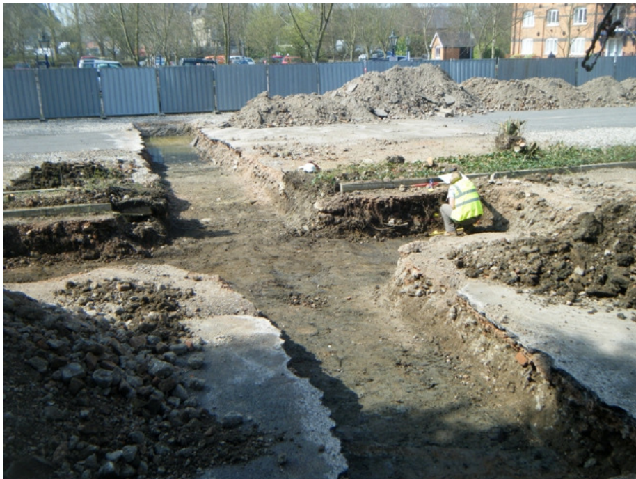
Plate 1: general site shot, view north-west
