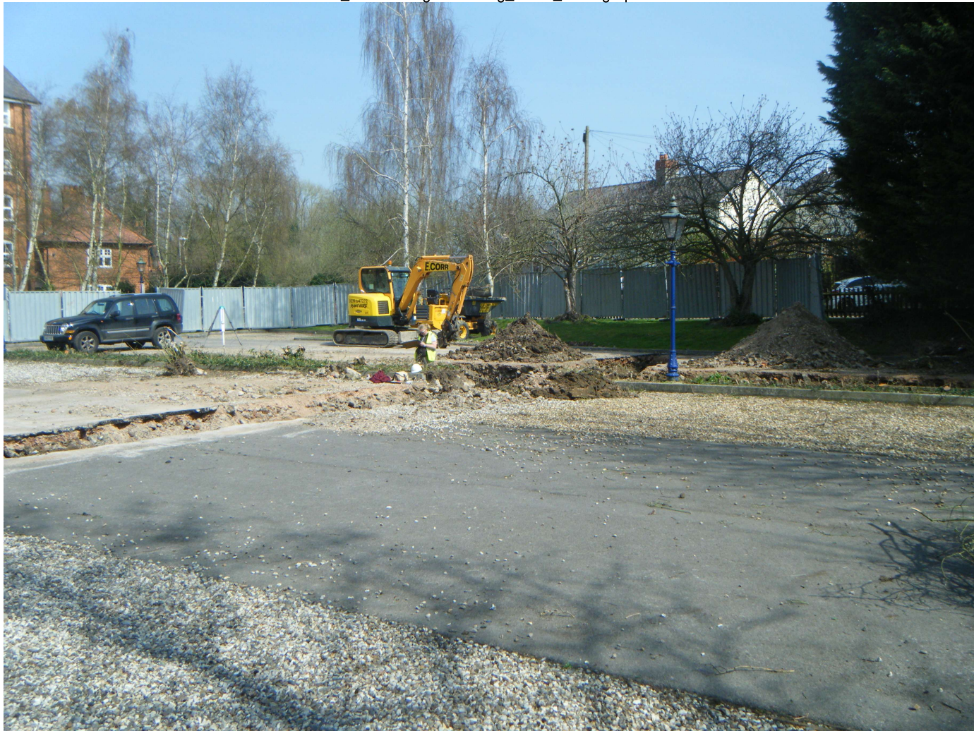
007 Site shot view NE
