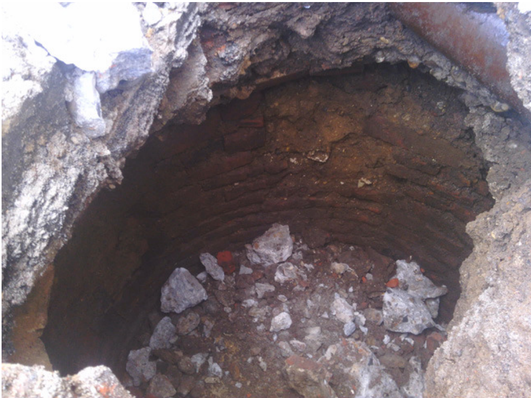
Photograph 2 Test-pit 1, view inside soakaway/cesspit F1, looking southeast
