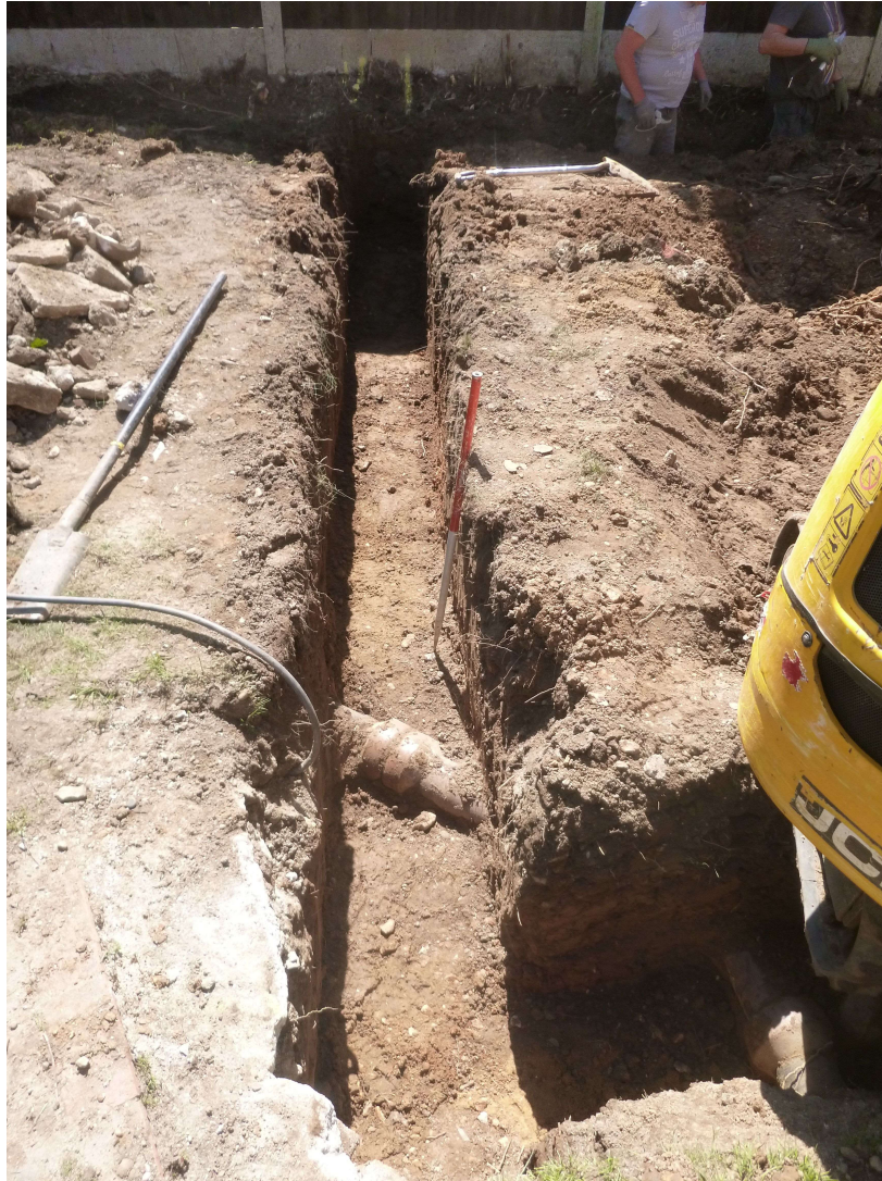
Photograph 2 Foundation trench – view south-east
