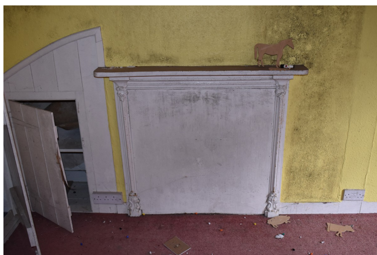
Photograph 26 Detail of blocked fireplace in room 15. Photograph taken facing north.
