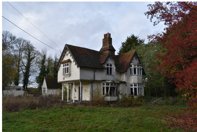
Photograph 2 Modern eastern and southern elevations, showing bay-window extensions, replacement windows and altered chimney. Photograph taken facing north-west.
