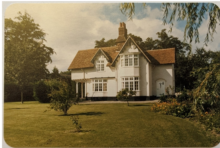
Photograph 3 East elevation of the house, taken from 1986 sales catalogue ERO SALE-D1321.
