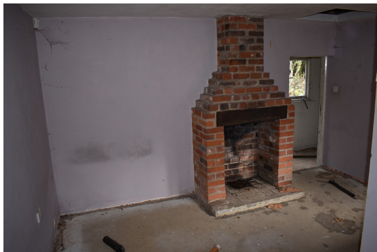
Photograph 12 Interior of room 3, showing rebuilt fireplace. Photograph taken facing north-east.
