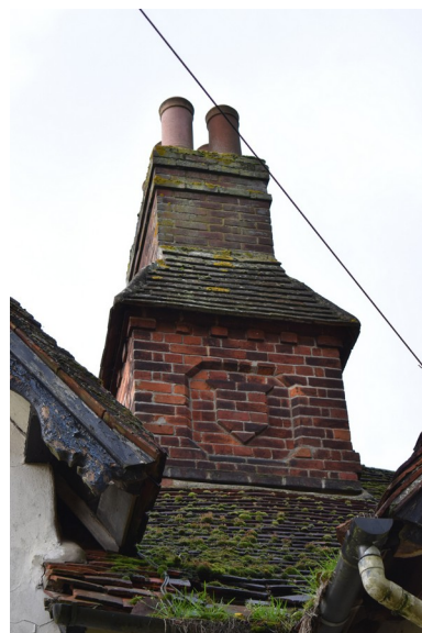
Photograph 5 East side of chimney-stack, showing shield emblem. Photograph taken facing north-west.
