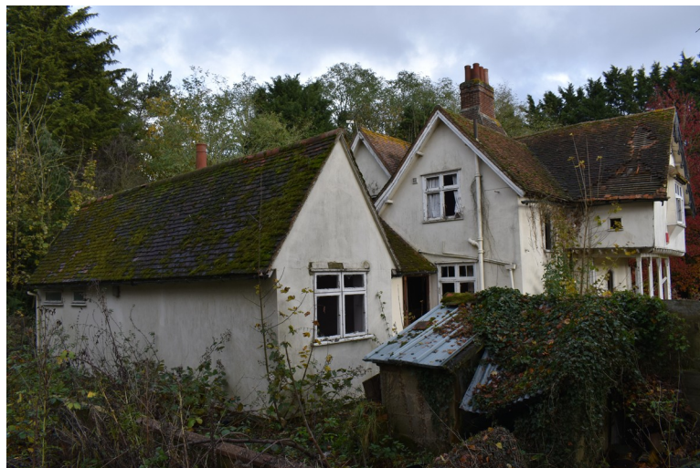
Photograph 7 Western elevation of building. Photograph taken facing north-east.
