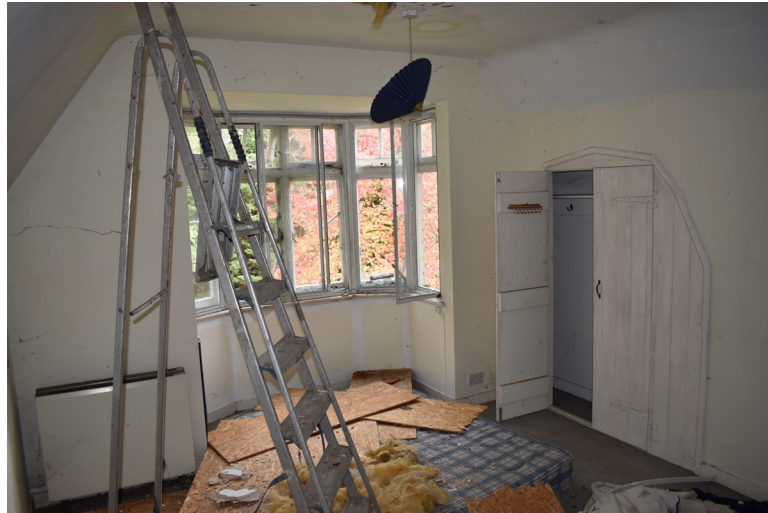
Photograph 23 Interior of room 12, showing oriel window extension and inserted cupboard to right. Photograph taken facing south-east.
