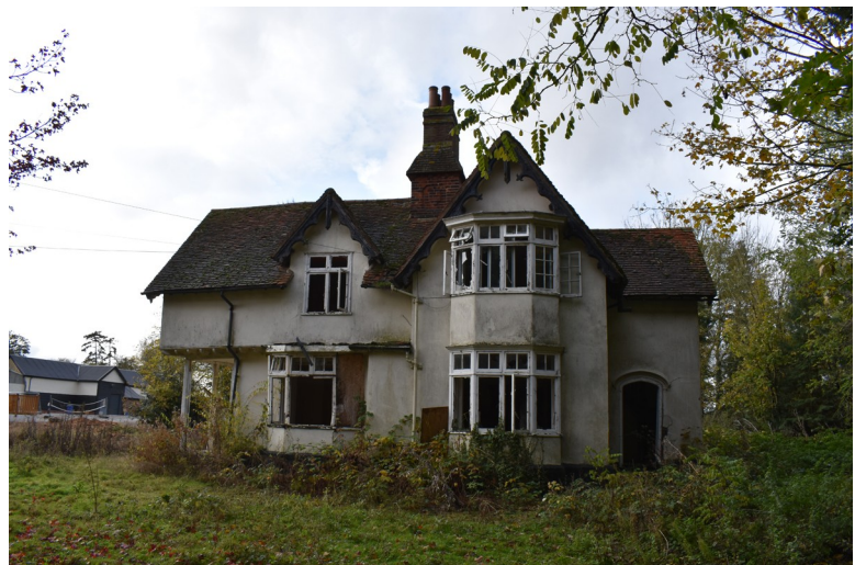
Photograph 10 Eastern elevation of building. Photograph taken facing west.
