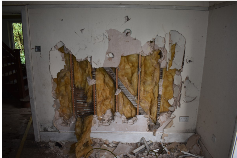
Photograph 19 Exposed section of timber-framing in room 9. Photograph taken facing north.
