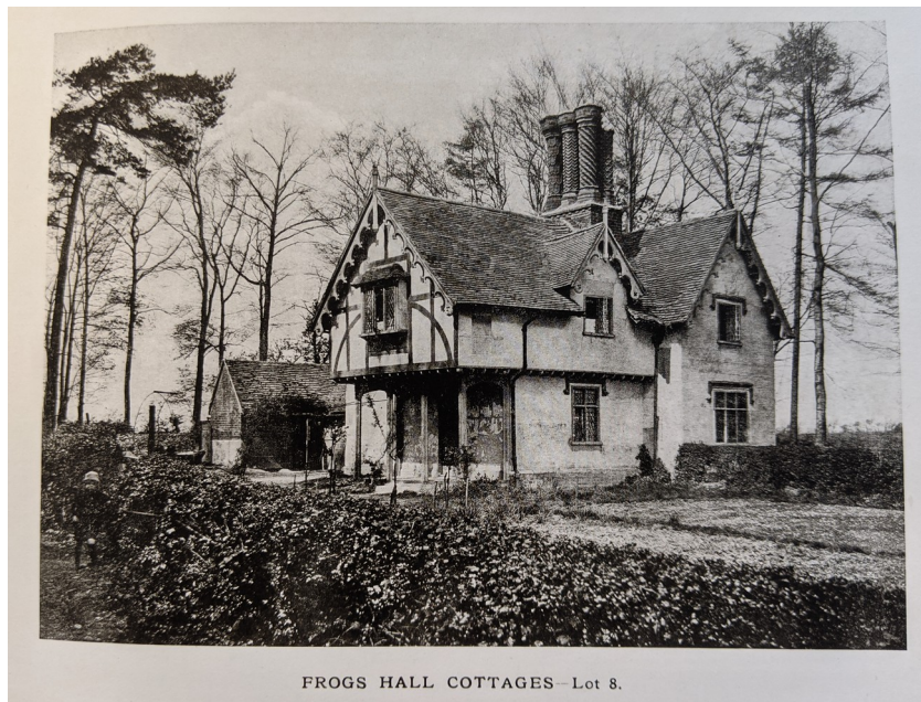
Photograph 1 Eastern and southern elevations of the house, taken from the 1921 sales catalogue. Note the original windows, chimney and faux timber-framing on the suspended section of the upper storey. Taken from ERO Sale-A57. Photograph taken facing north-west.
