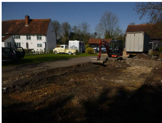
Photograph 1 Stripped area – looking northwest
