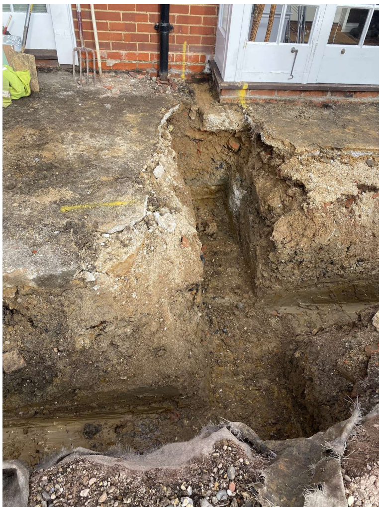
Photograph 2 The foundation trenches, looking northwest
