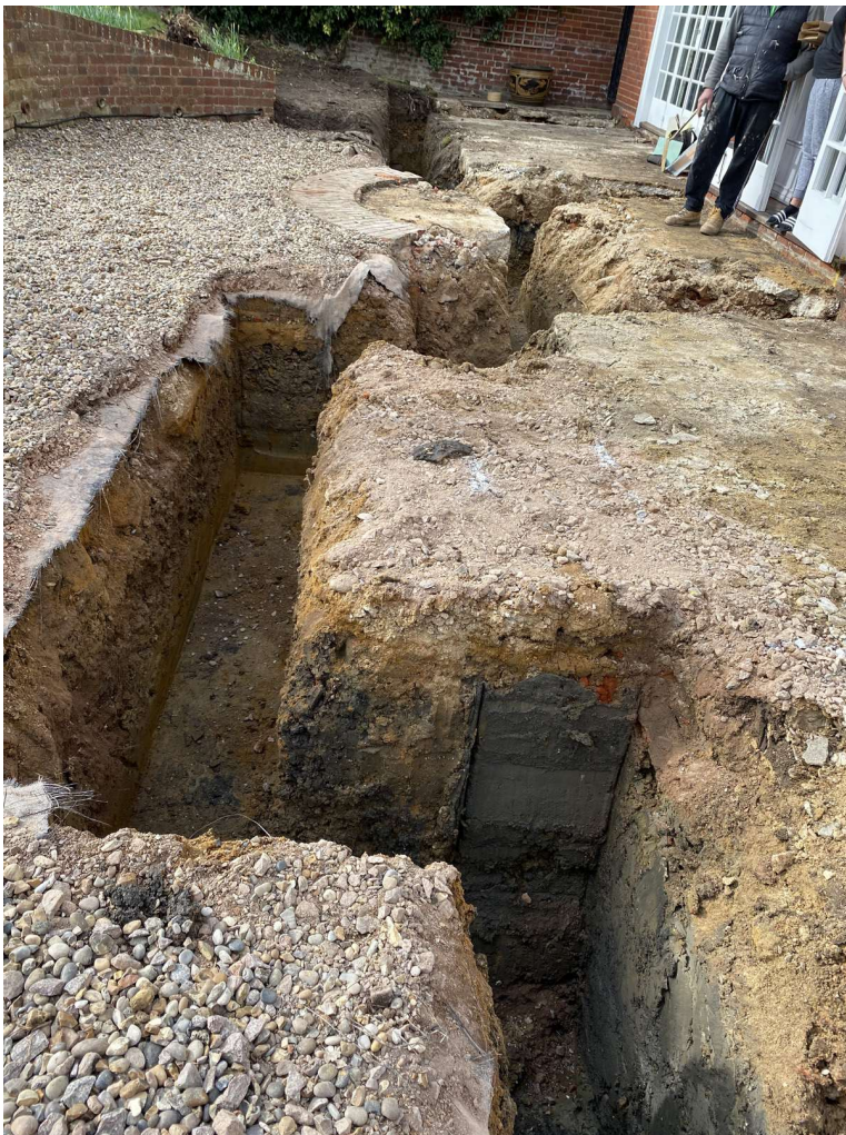
Photograph 1 The foundation trenches, looking southwest
