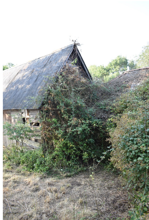
Photograph 4 North-west elevation of outbuilding, showing overgrowth. Photograph taken facing south.
