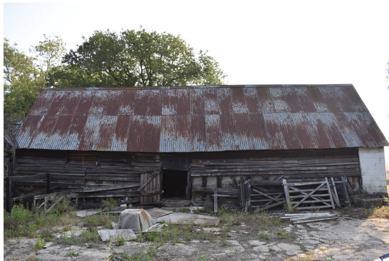
Photograph 1 South-west elevation of outbuilding, bays 2 and 3. Photograph taken facing north-east.
