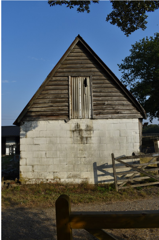
Photograph 3 South-east elevation of the outbuilding. Photograph taken facing north-west.
