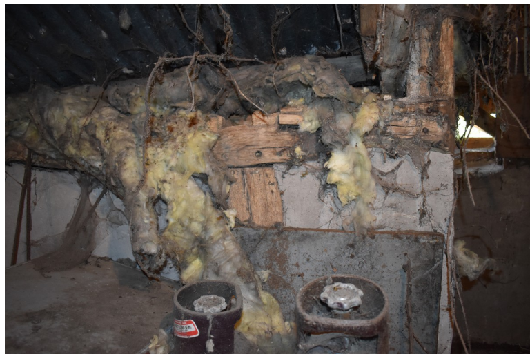
Photograph 7 Detail of small section of exposed ?hand-sawn timber in bay 1. Photograph taken facing north-east.
