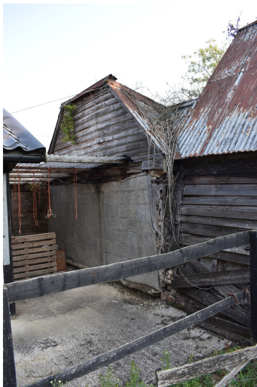
Photograph 2 South-west elevation of outbuilding, bay 1, showing concrete block infilling. Photograph taken facing north.
