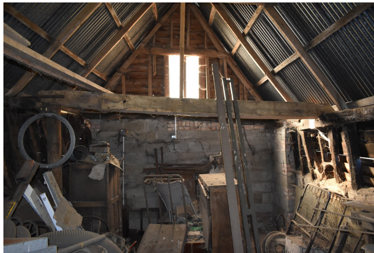
Photograph 15 Interior of bay 3. Photograph taken facing south-east.
