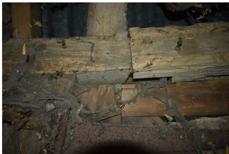
Photograph 14 Detail of face-halved scarf in bay 2, above double-doors on north-east elevation. Photograph taken facing north-east.
