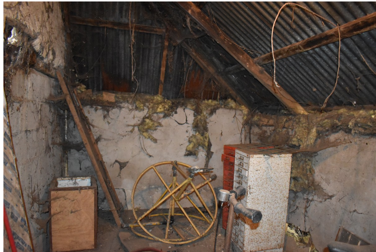
Photograph 6 Interior of bay 1. Photograph taken facing north-west.
