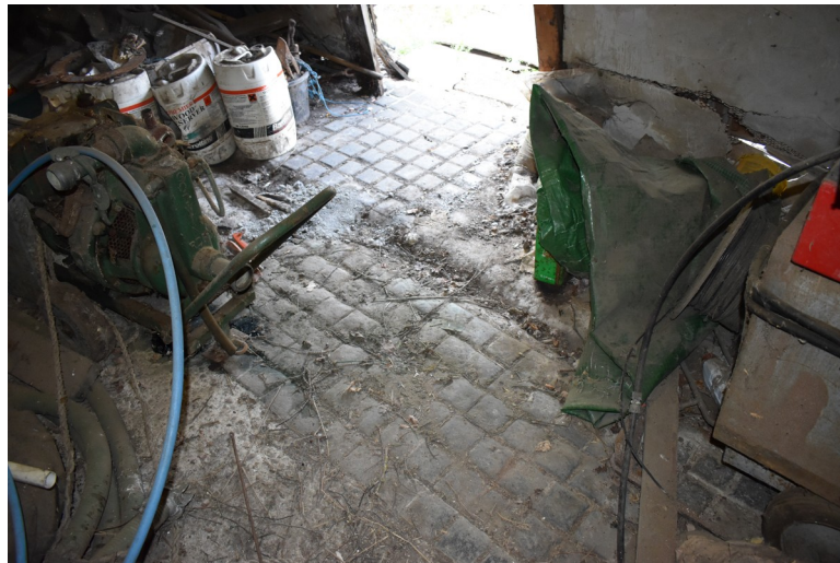
Photograph 13 Detail of surviving cobbled floor and drainage run in bay 2. Photograph taken facing south.
