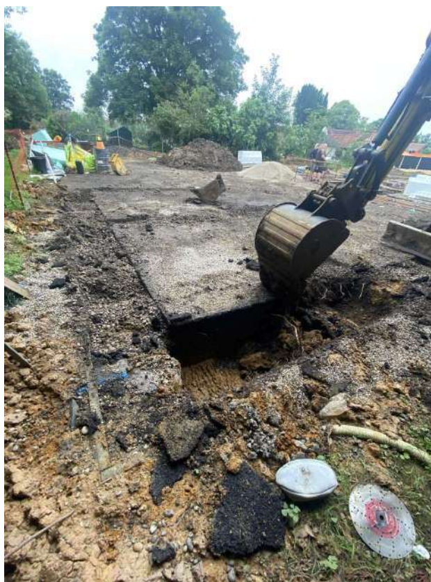
Photograph 5 Garage foundation trench – view NW
