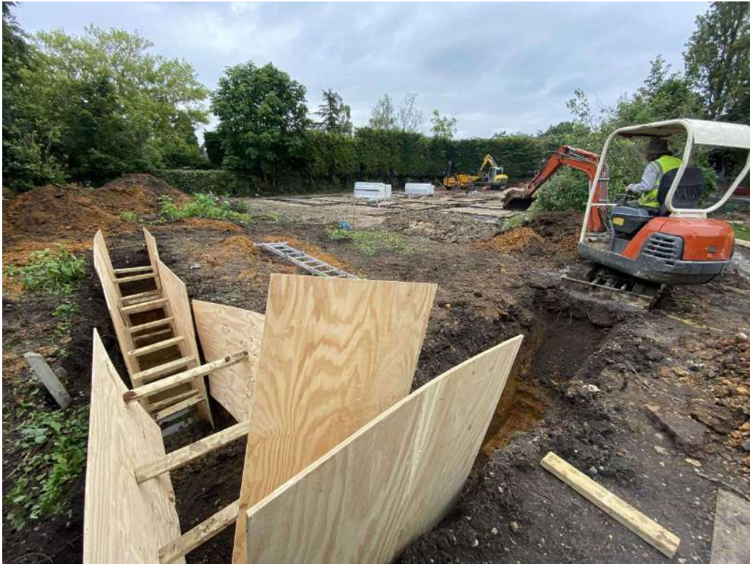
Photograph 3 Site shot with Summer house foundation trench in foreground – view S
