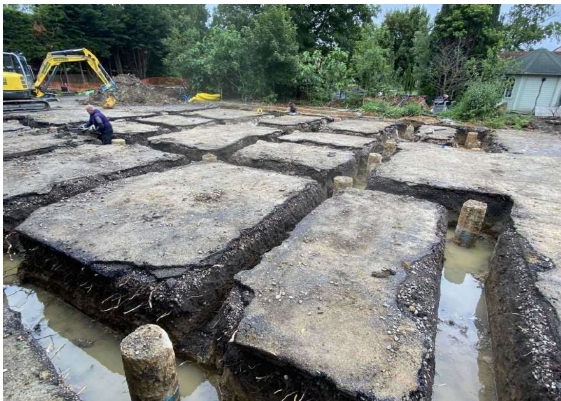
Photograph 1 Main house foundation trench – view W
