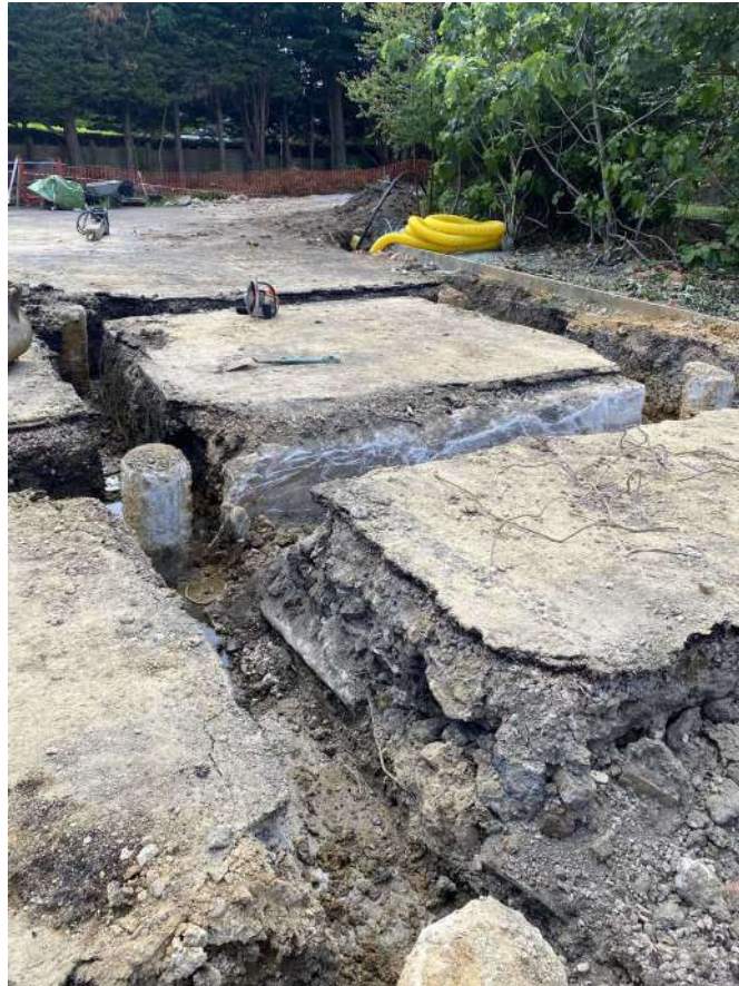
Photograph 2 Main house foundation trench with swimming pool backfill – view W
