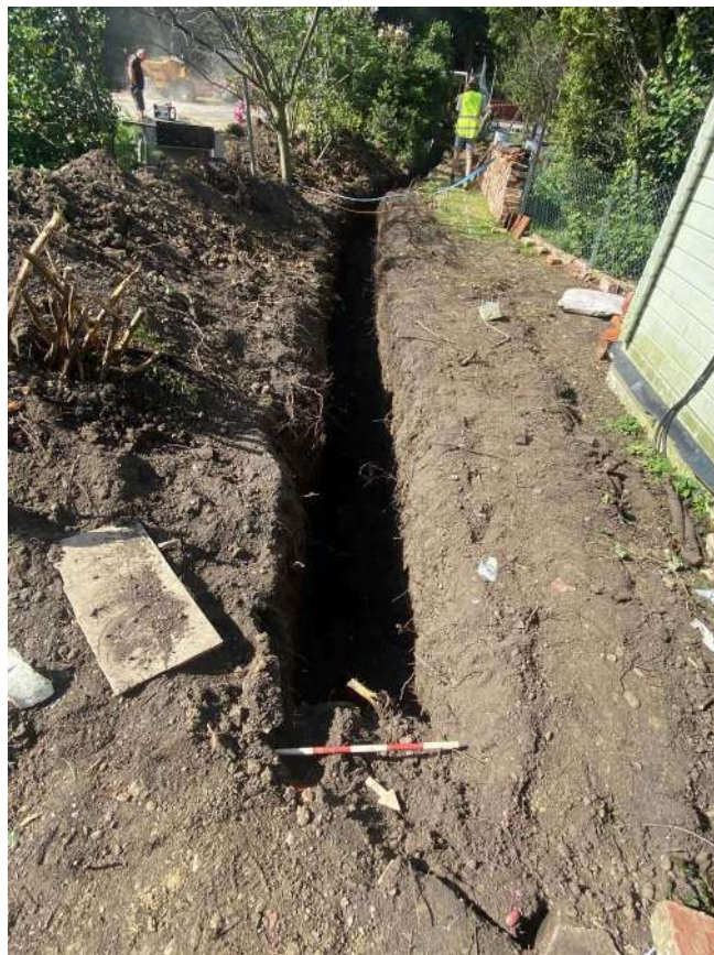
Photograph 4 Garden wall foundation trench – view SW
