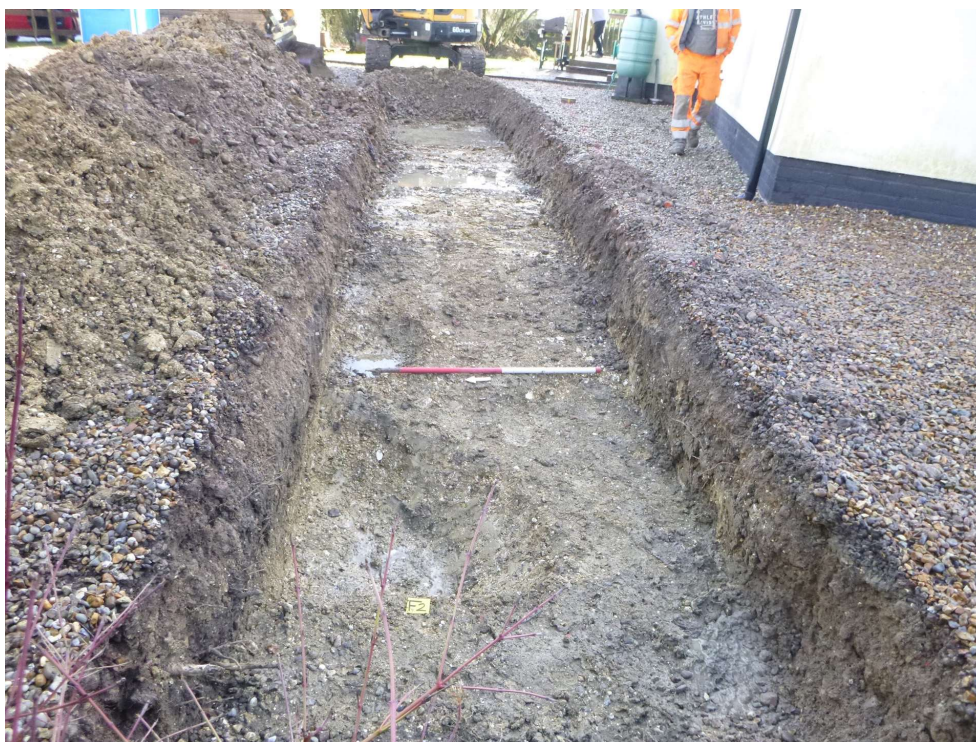
Photograph 1 Trench T1 with F1 and F2 in foreground, looking southeast
