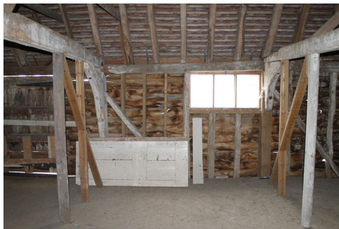
Photograph 17 Southern elevation of bay 2 on first-floor, showing modern studs, window and scarf joint. Photograph taken facing south.
