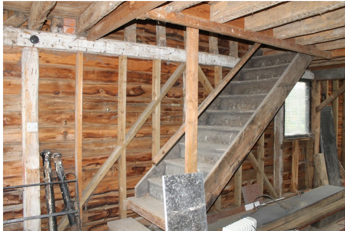
Photograph 14 Inserted staircase in bay 1. Photograph taken facing north-west.
