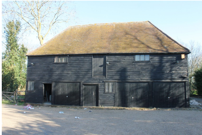
Photograph 1 Southern elevation of building. Photograph taken facing north.
