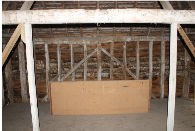
Photograph 13 Detail of western elevation of bay 1, showing re-used hand-sawn timber. Photograph taken facing west.
