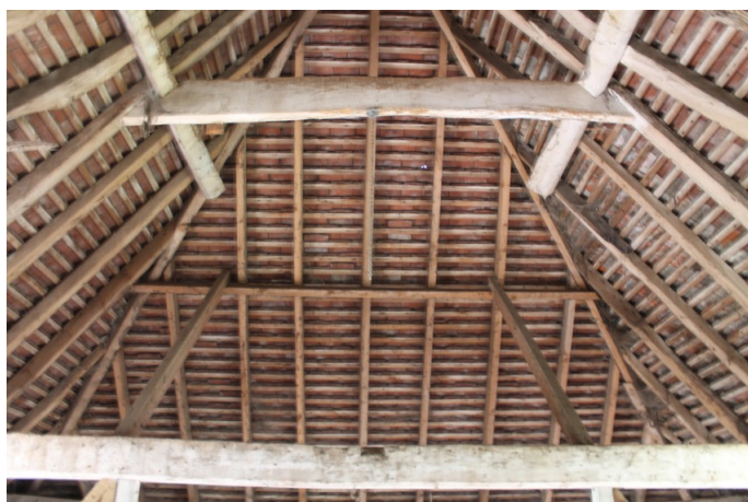
Photograph 12 Detail of roof hip above bay 1, entirely constructed of machine-cut timber.
