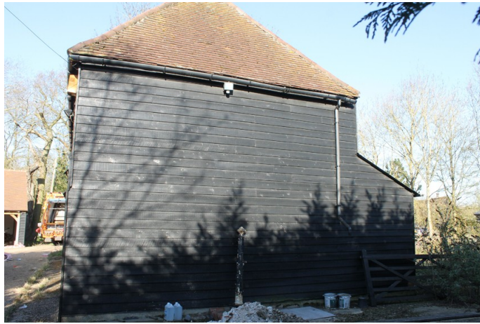
Photograph 3 Eastern elevation of building. Photograph taken facing west.
