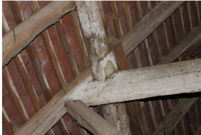
Photograph 18 Detail of carpenter's mark 'II' on collar and rafter between bays 2 and 3. Photograph taken facing north-east.
