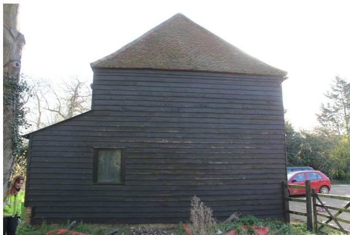
Photograph 5 Western elevation of building. Photograph taken facing east.
