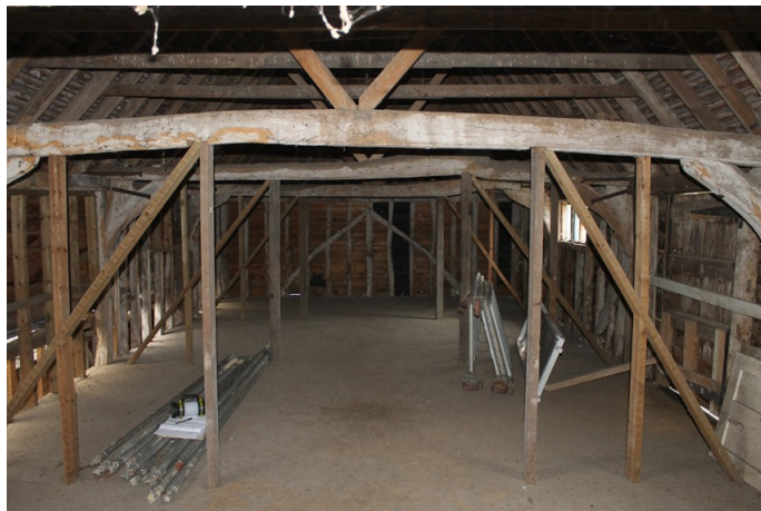
Photograph 7 First-floor, showing tie-beams and machine-cut timbers. Photograph taken facing east.
