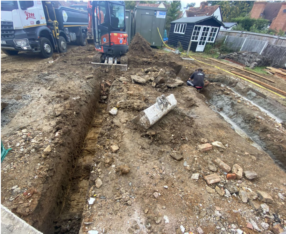
Photograph 3 Excavation of footings on north-west side of property, looking north-west
