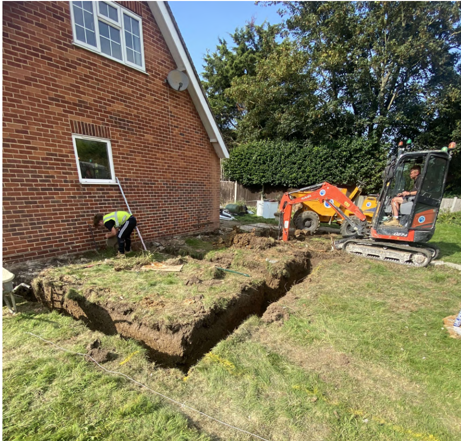
Photograph 1 Excavation of footings on south-east side of property, looking north
