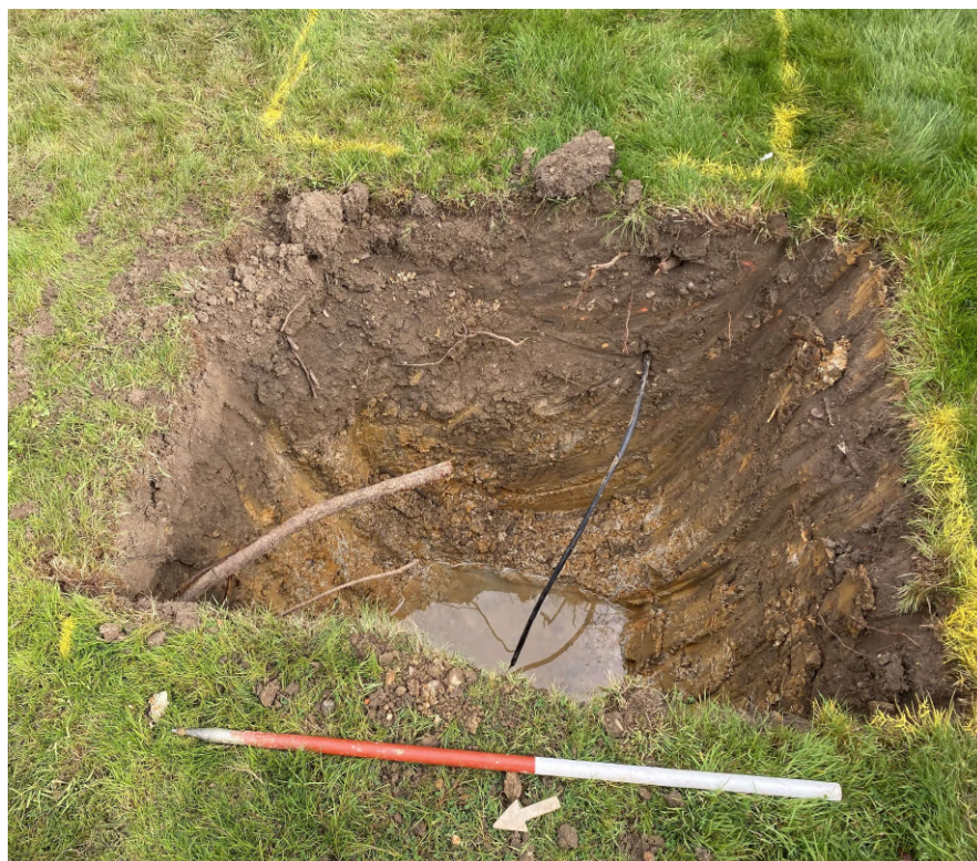
Photograph 5 Partial excavation of northern soakaway, looking west
