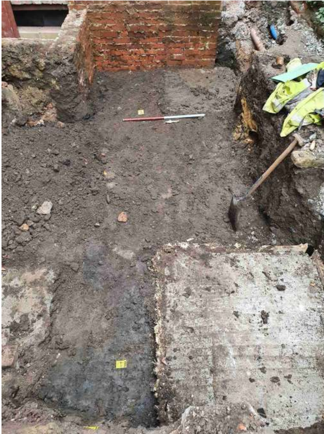
Photograph 2 F1 and L2, plus poured concrete pads – view east
