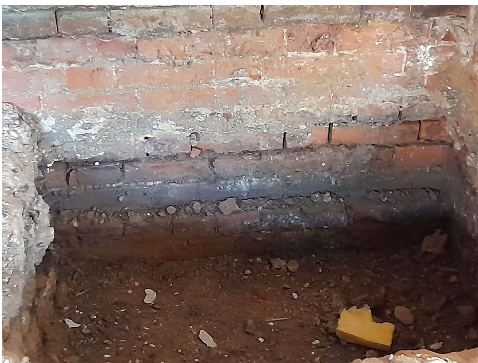
Photograph 1 Test pit showing depth of foundations, looking northeast.
