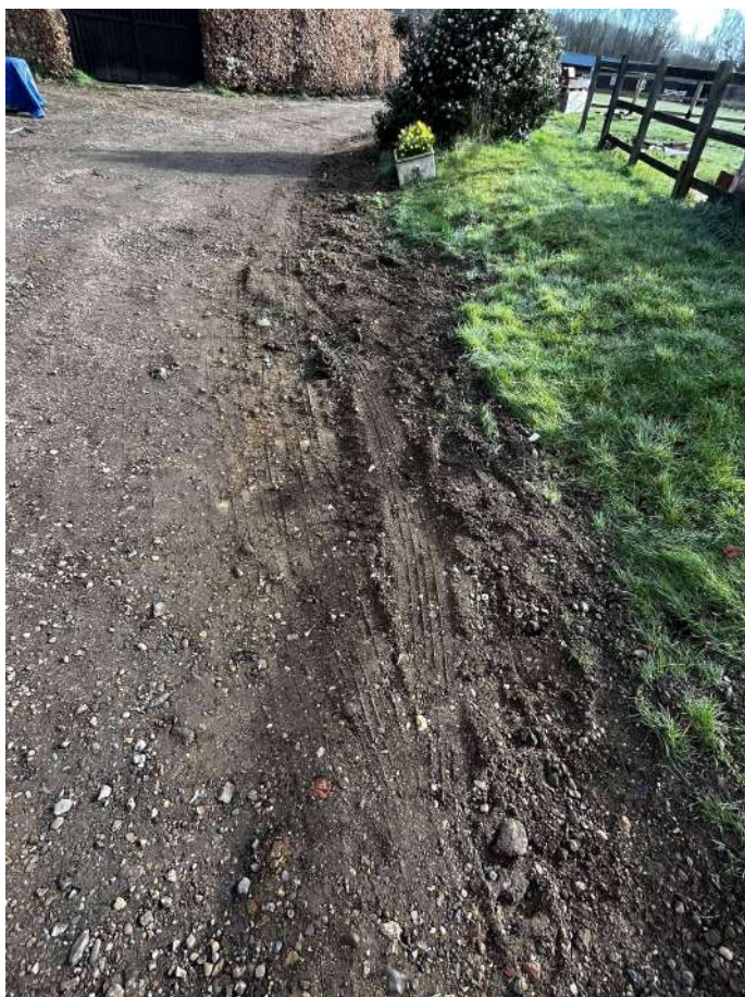
Photograph 8 Cable trench, looking south-east
