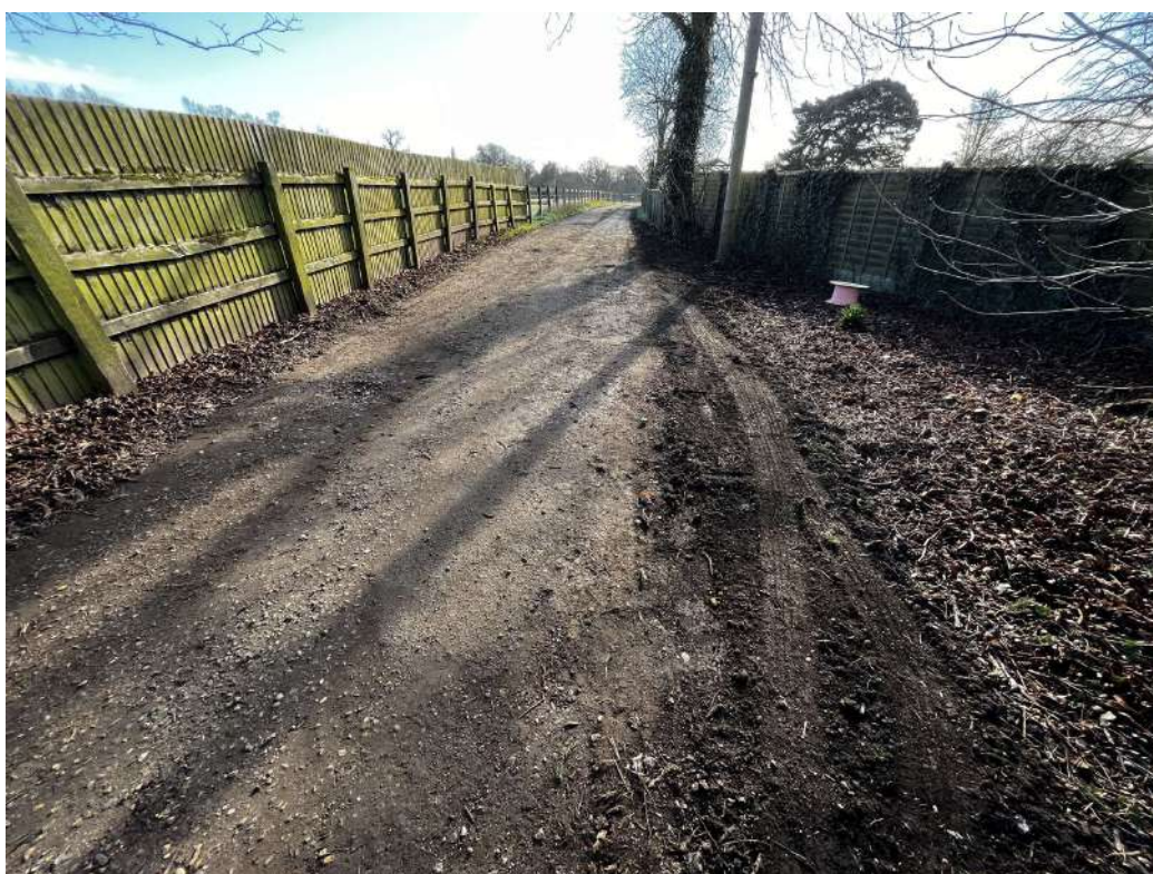
Photograph 7 Backfilled cable trench, looking south
