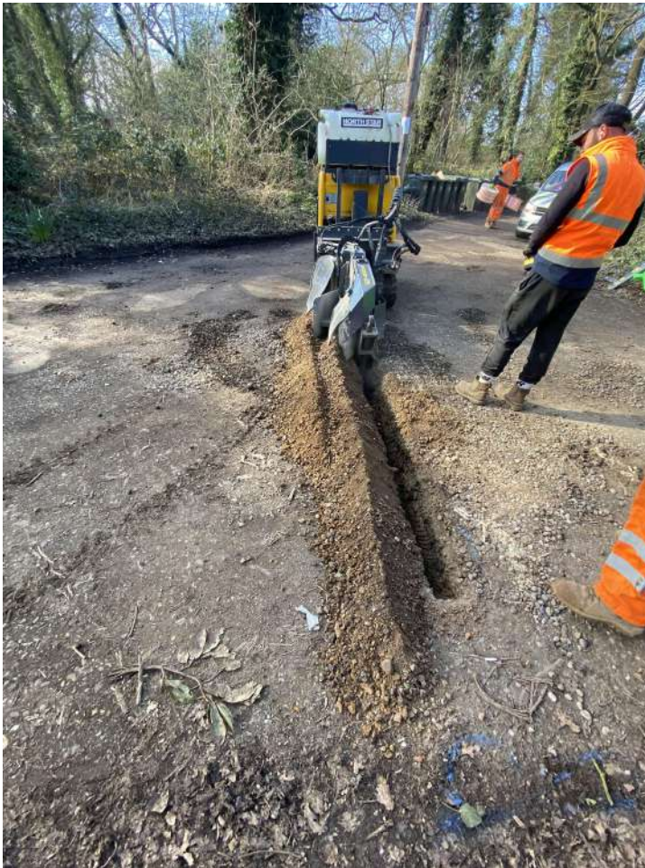
Photograph 1 Cable trench, looking south-west
