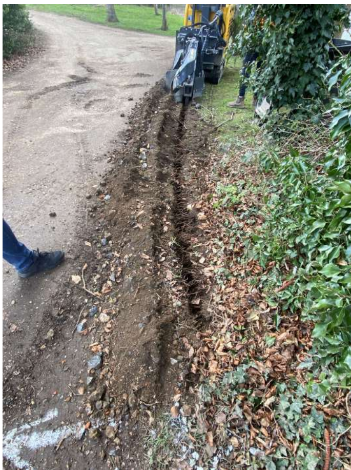
Photograph 6 Cable trench, looking south-east
