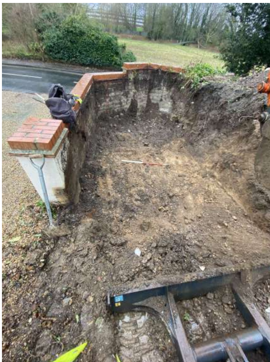
Photograph 1 Excavation of the bank to natural, looking west
