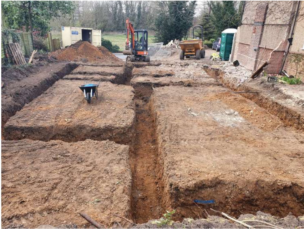
Photograph 4 Site shot of completed foundation trenching, looking west
