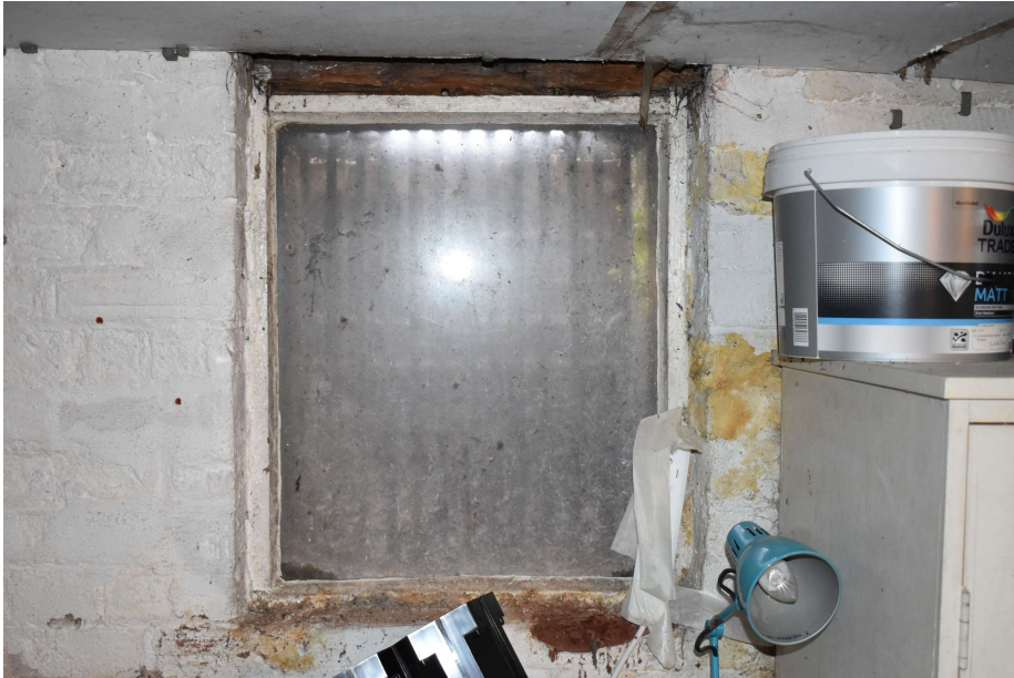
Photograph 5 Detail of window. Photograph taken facing south.
