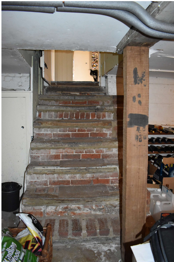
Photograph 4 Detail of interior stairs. Photograph taken facing north.
