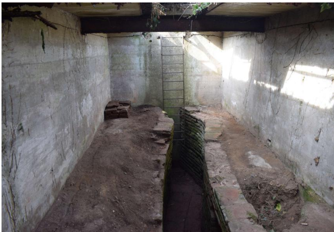
Photograph 2 Interior of drain, looking south south-east.
