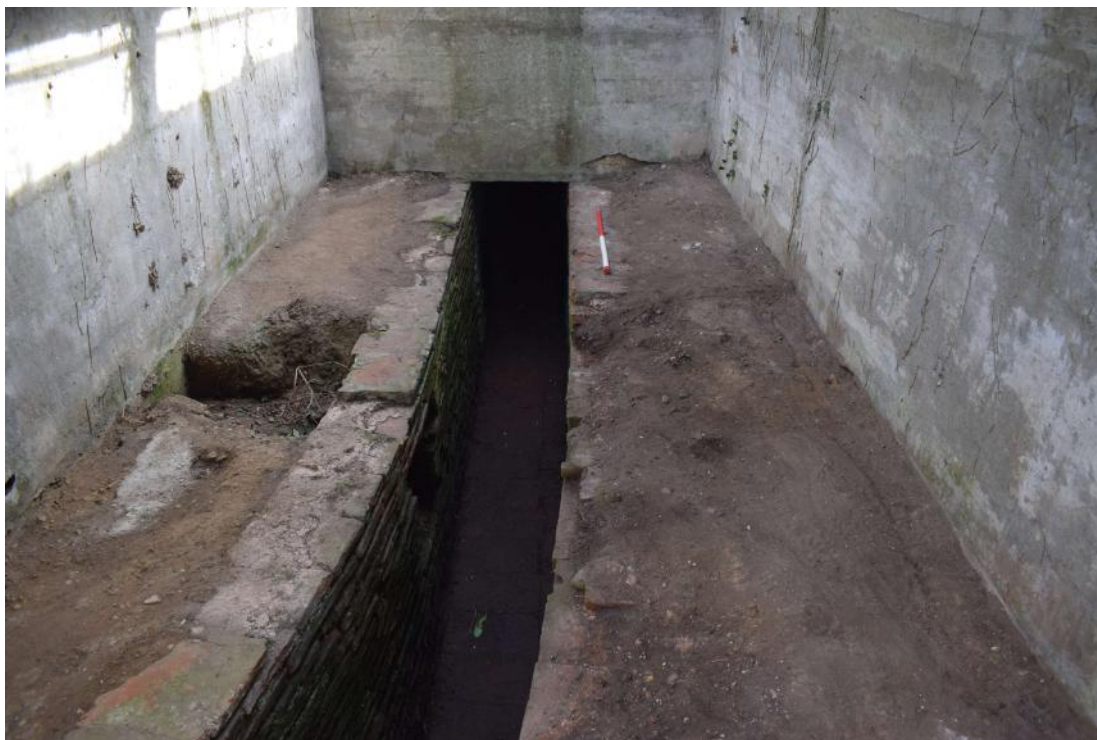
Photograph 1 Interior of drain, looking north north-east.
