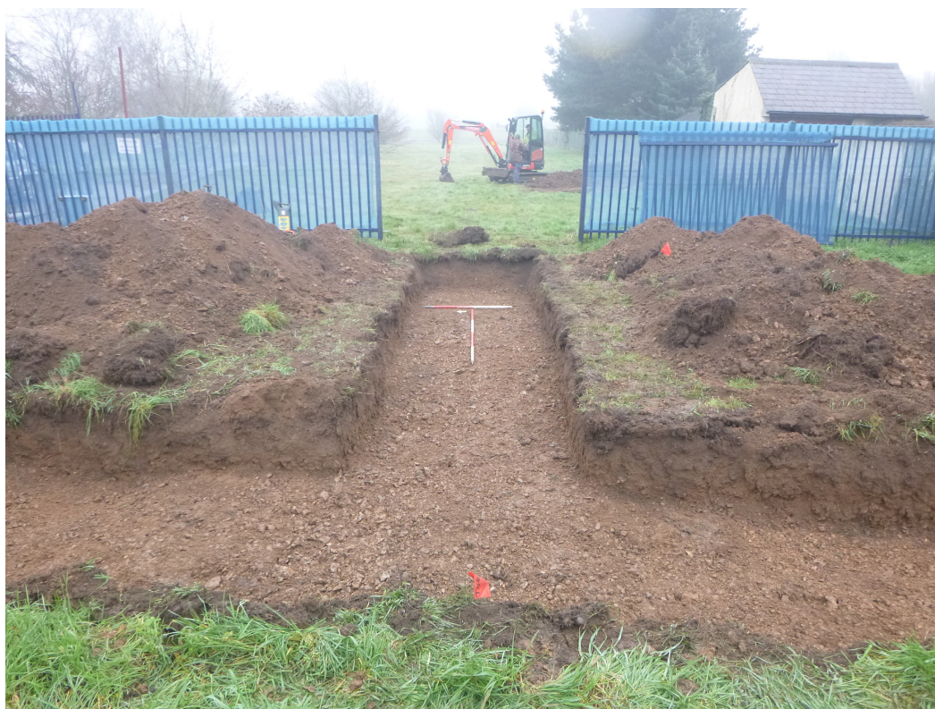
Photograph 1 Trench 2 – view east
