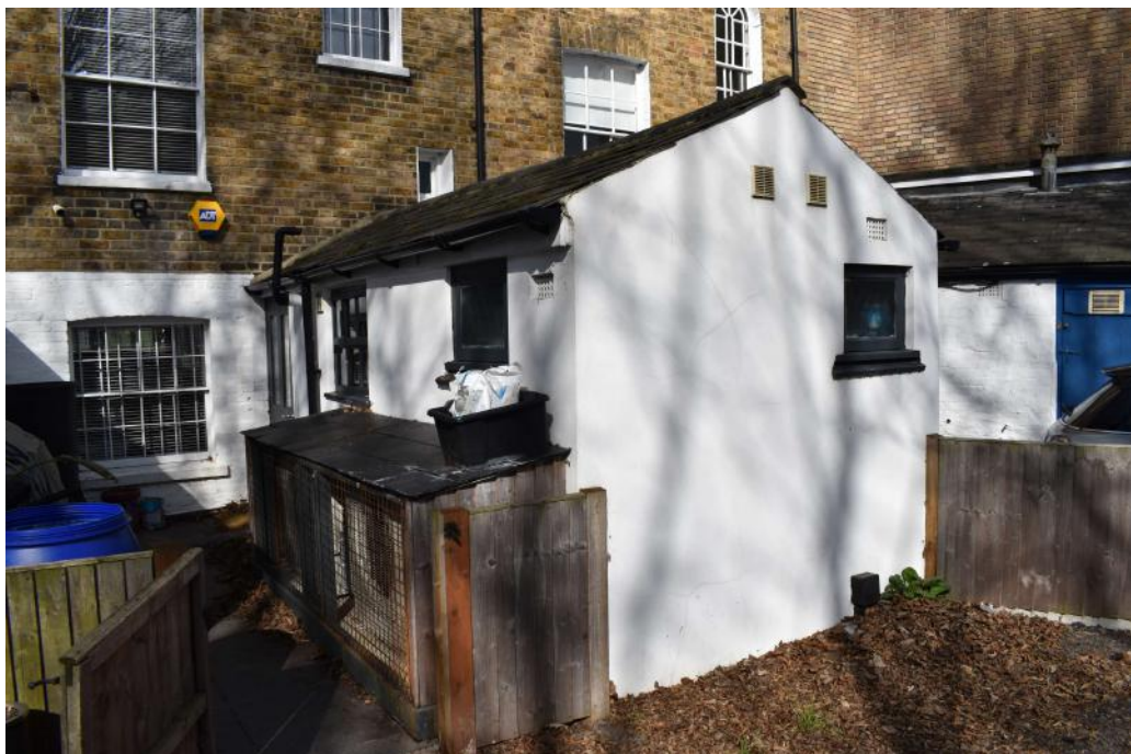
Photograph 7 South-east and south-west elevations of no 61. Photograph taken facing north.
