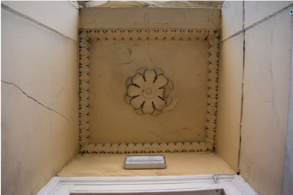
Photograph 4 Detail of original plaster decorative ceiling in entrance way of no 63.
