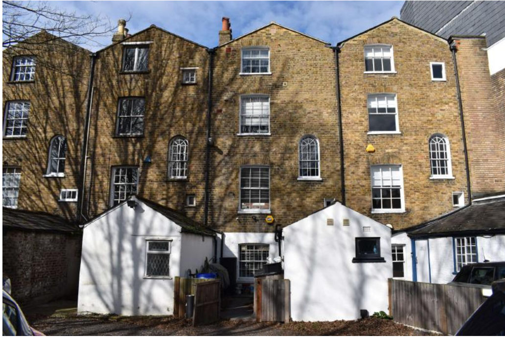
Photograph 5 South-east elevation of nos 61 and 63. Photograph taken facing north-west.
