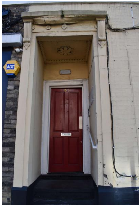
Photograph 3 Detail of entrance to no 63. Photograph taken facing south-east.
