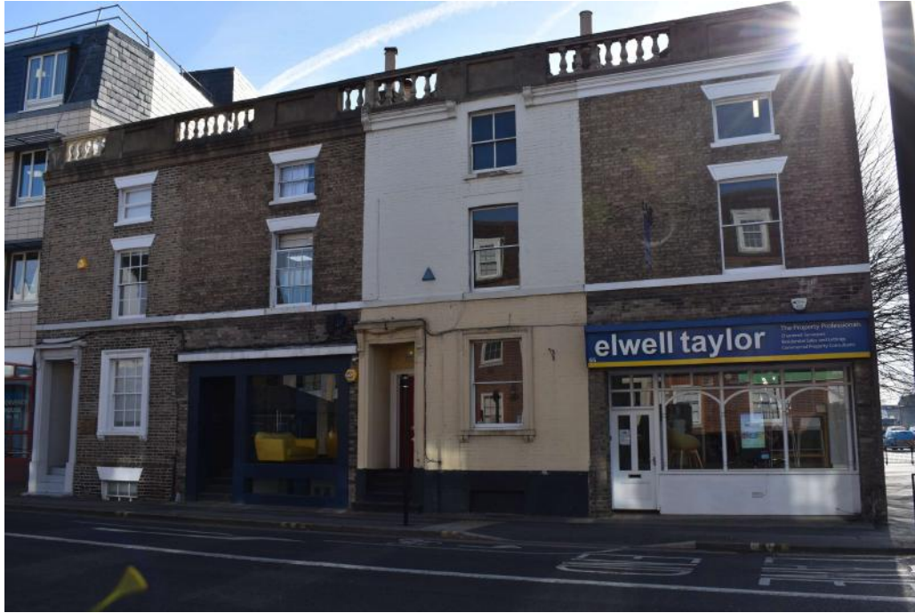
Photograph 1 North-west elevations of no 61 and 63. Photograph taken facing east.
