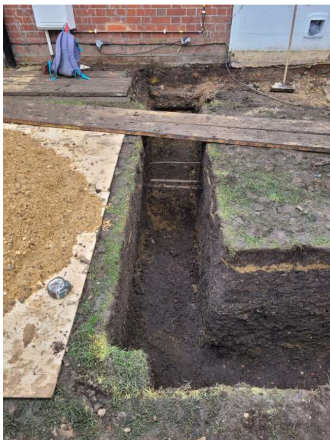
Photograph 4 Working shot of trench, south-south-east
