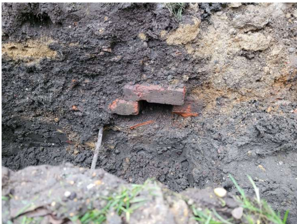
Photograph 1 Culvert F1, looking east-north-east
