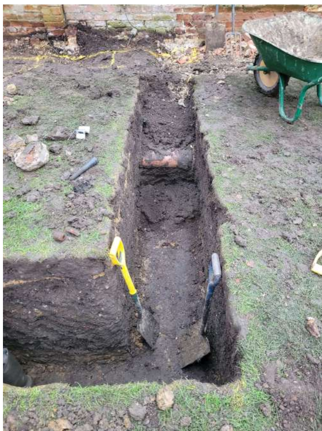
Photograph 3 Working shot of trench, looking west-south-west
